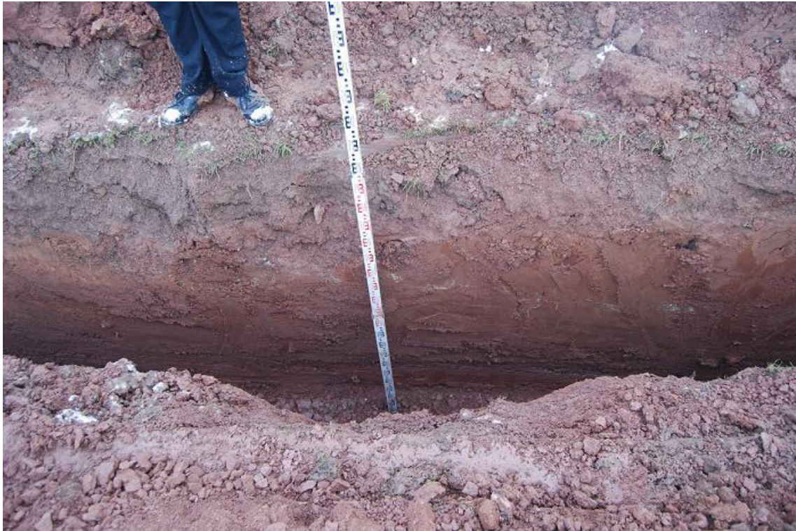
Plate 8, West facing section of the Service Trench
