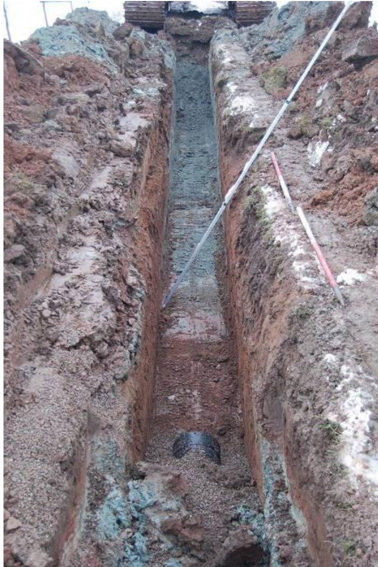
Plate 10, The Service Trench and the variation in natural, facing north
