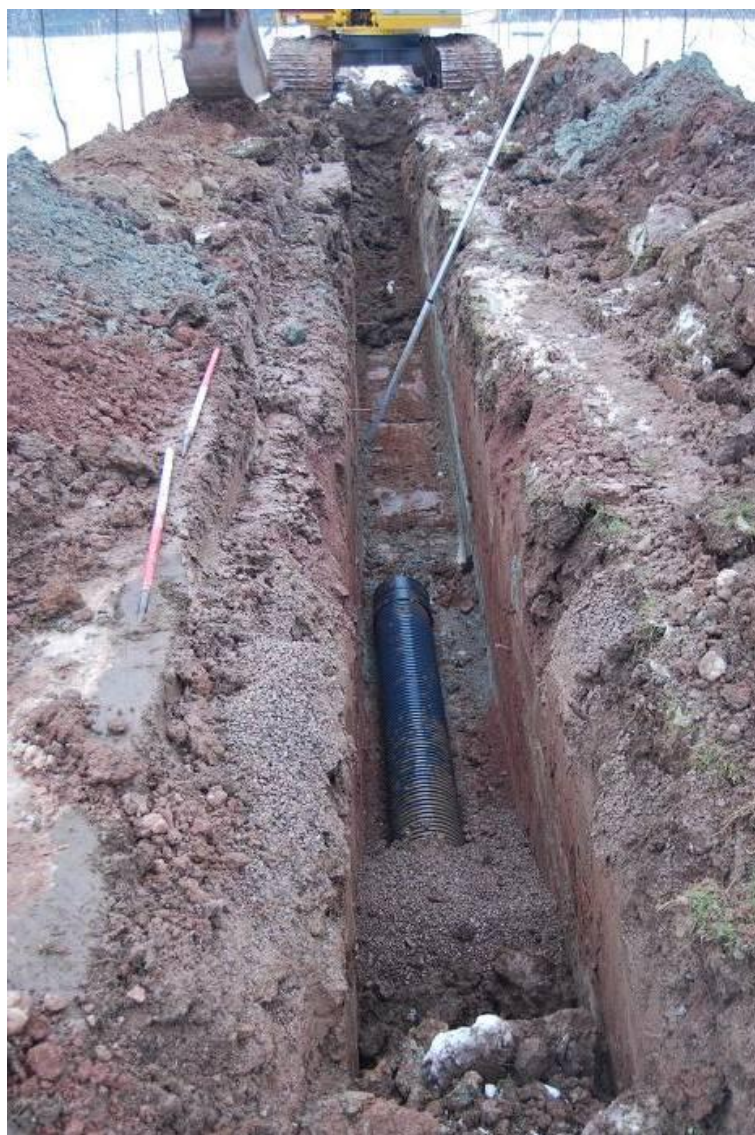
Plate 9, The Service Trench, facing north
