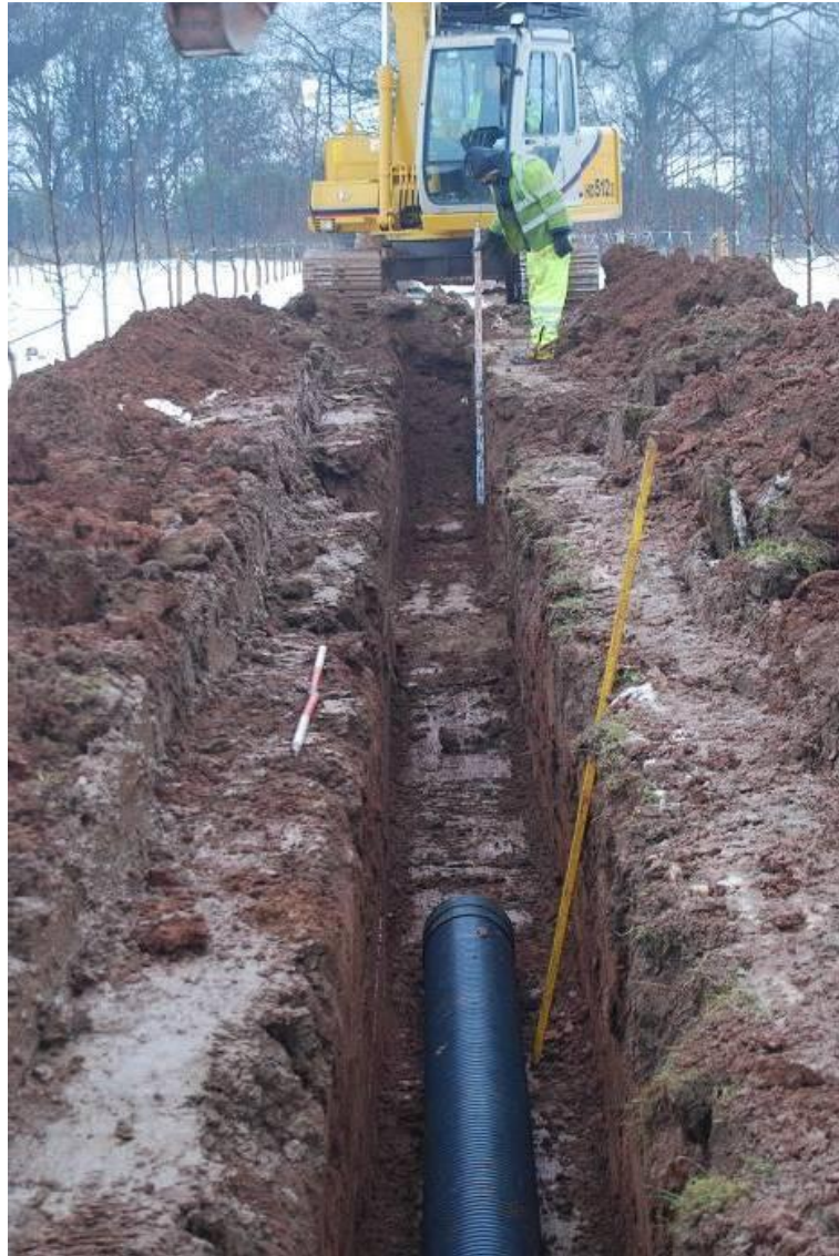
Plate 13, The Service Trench from the north
