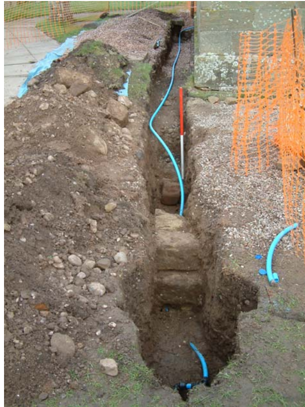
Plate 5. Service trench to the west of the nave viewed from the south
