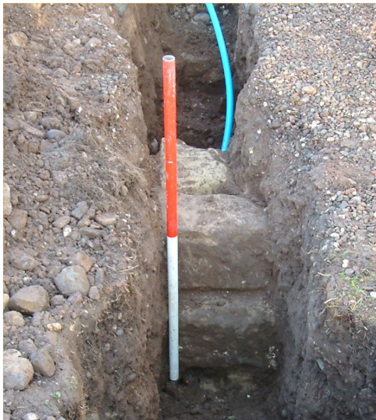
Plate 4. Possible foundation 1007 from the south
