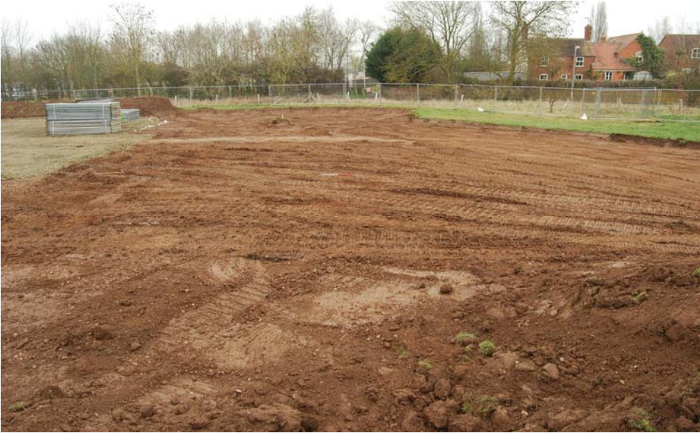
Plate 2: The north end of Area 2, looking north.
