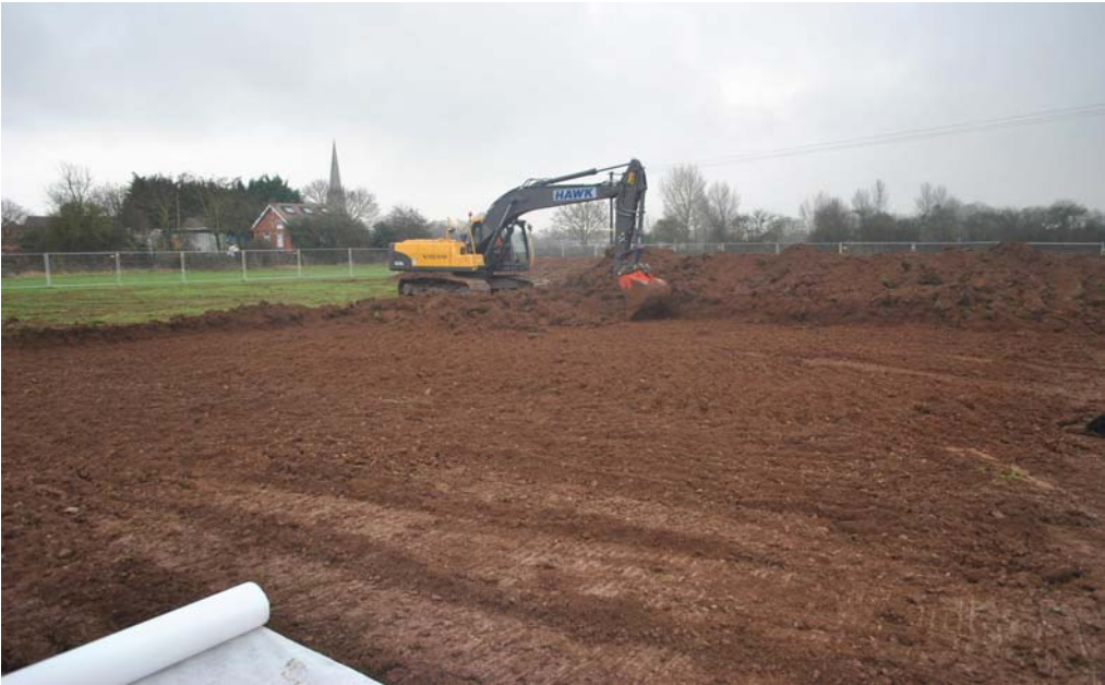
Plate 1: Area 1, the compound during stripping, looking southeast.
