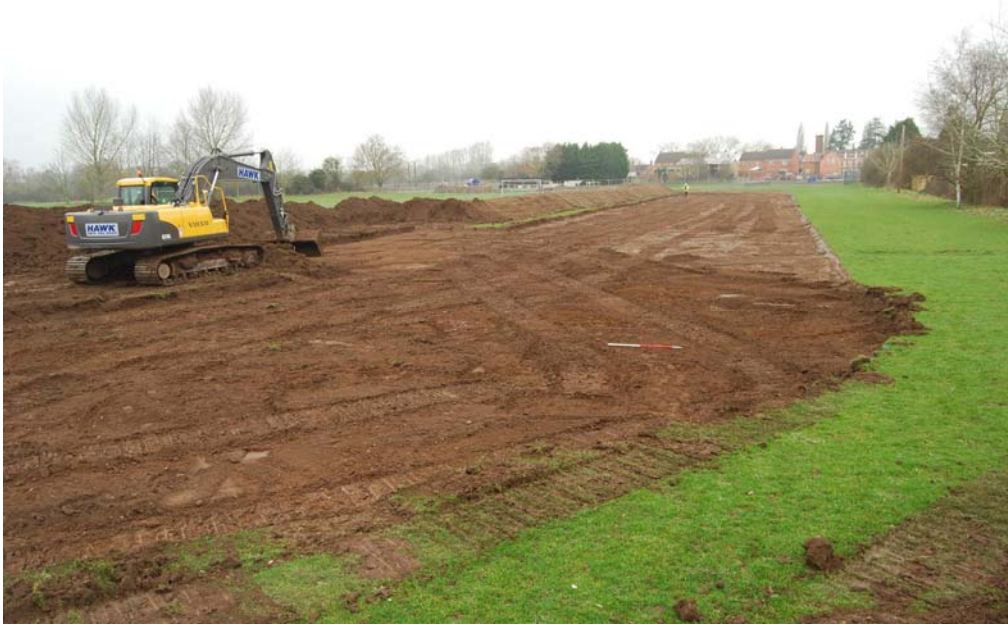
Plate 4: Area 3 during stripping, looking north.
