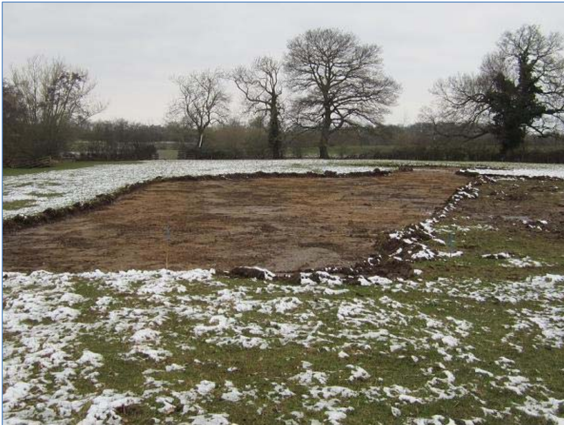
Plate 5 Furze farm topsoil strip showing furrows running northwest-southeast. View southeast
