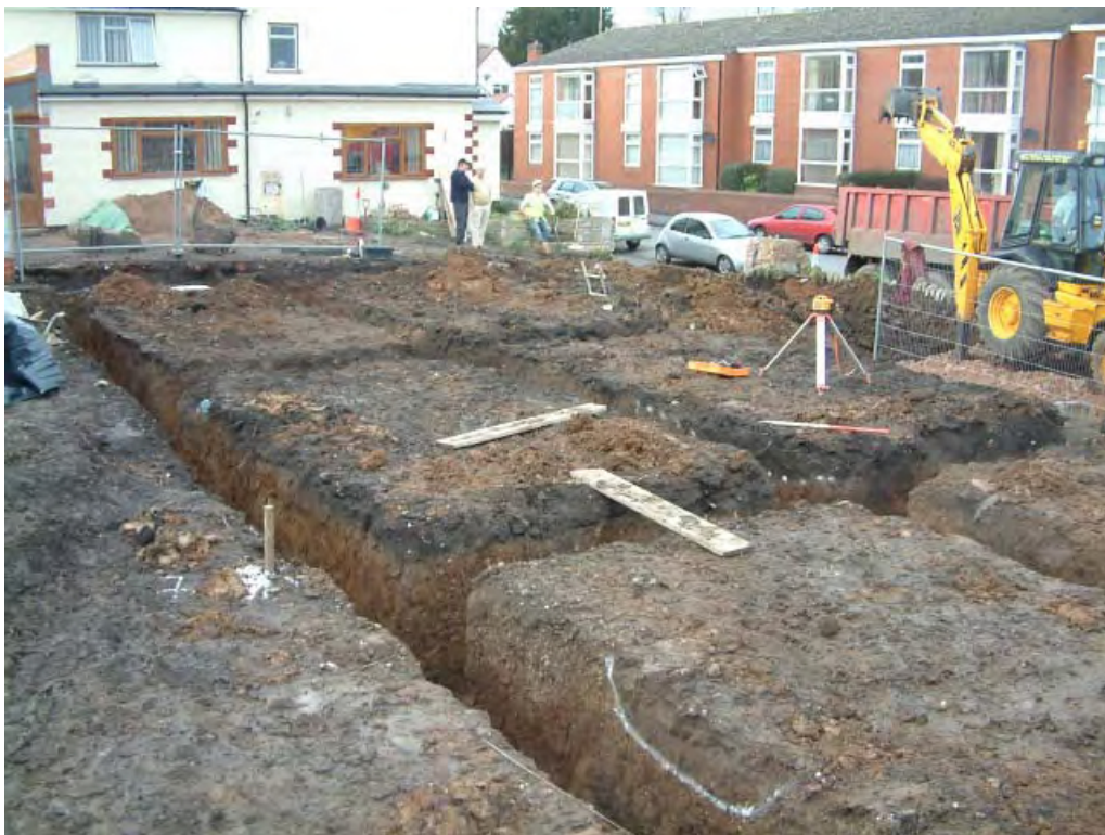
Plate 8 Main foundation trench, facing north-west.
