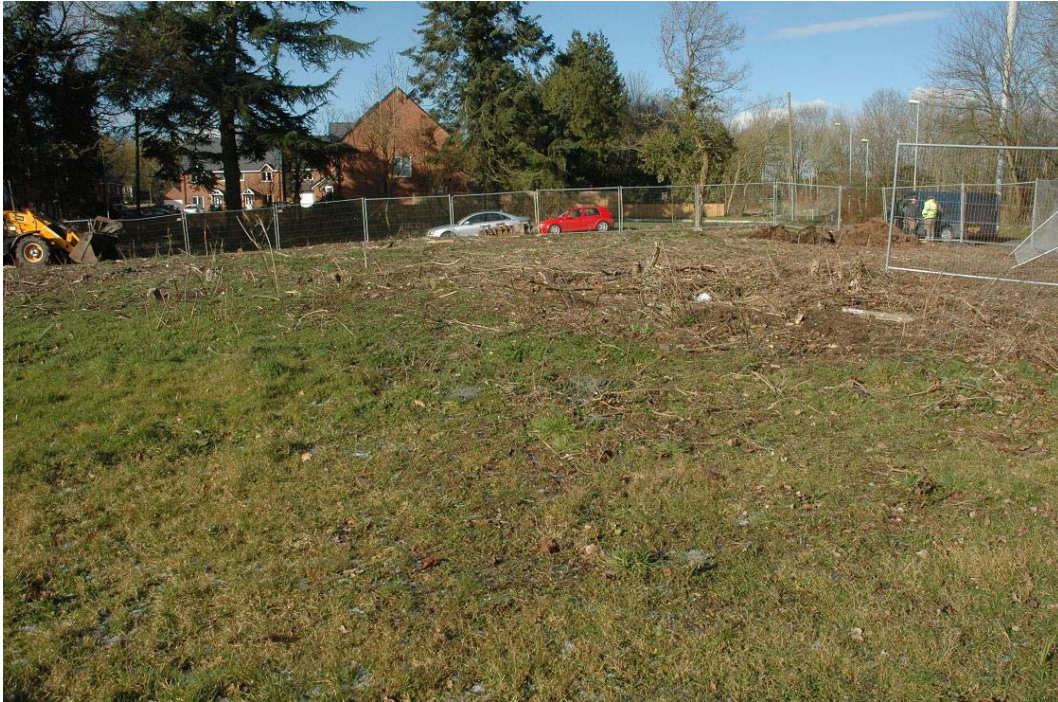
Plate 1 Site prior to excavation
