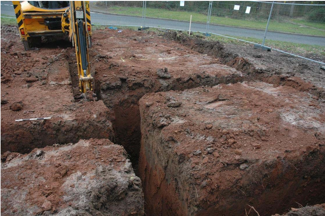
Plate 5 General south east looking shot of Plot 3 foundation trenches.
