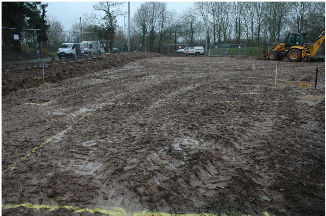
Plate 2 The site looking north after topsoil has been removed.
