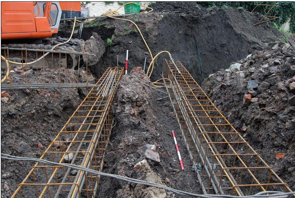
Plate 4: Trenching on north side of site, view west
