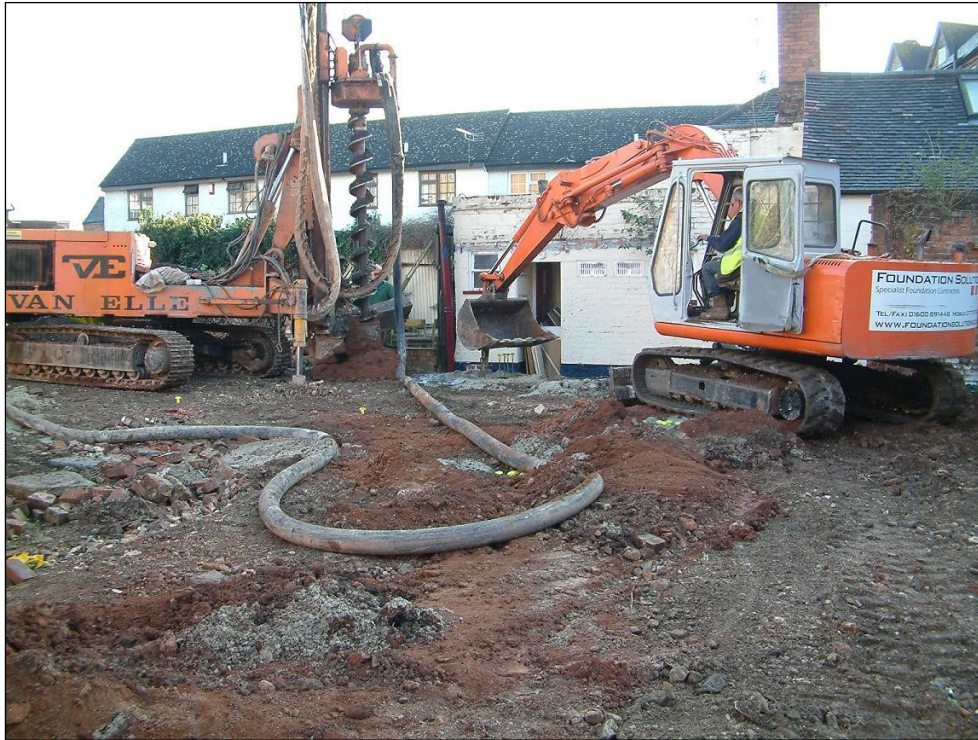
Plate 1: Example of borehole drilling in progress
