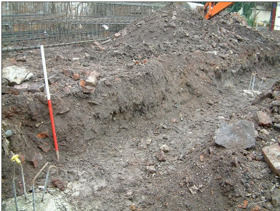
Plate 2: Foundation trenching along west side of site, view north-east
