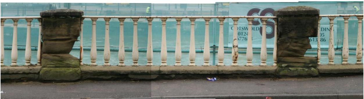
Plate 16: Bewdley Bridge abutment road side, pier 4 (on left) to 3
