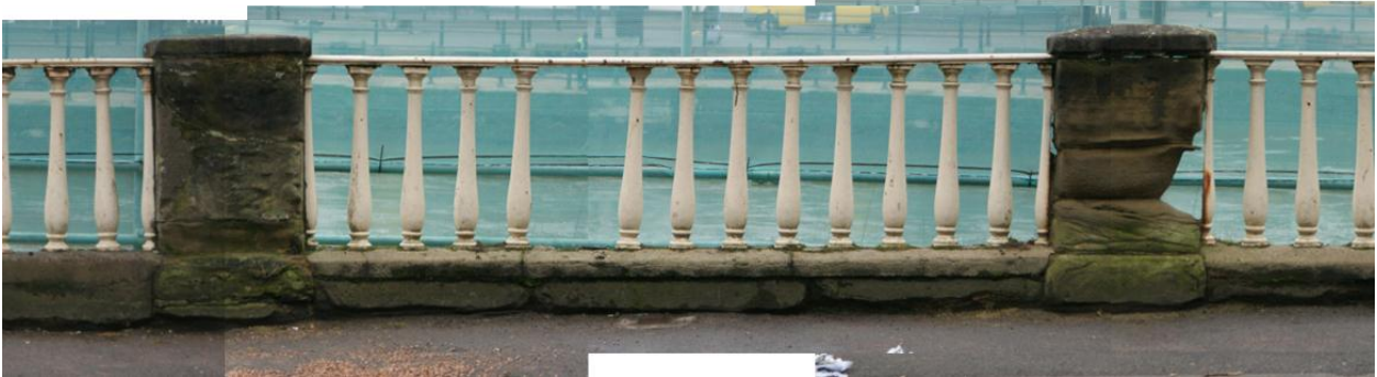
Plate 15: Bewdley Bridge abutment road side, pier 5 (on left) to 4
