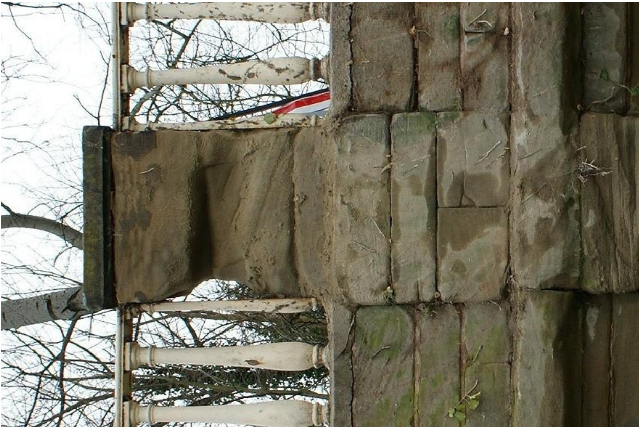
Plate 12: River side elevation of pier 2
