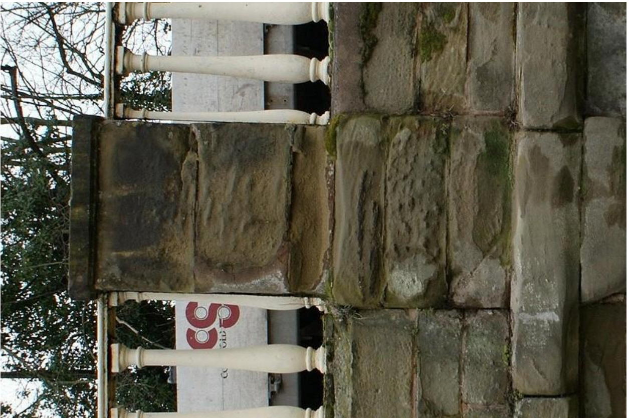
Plate 6: River side elevation of pier 5
