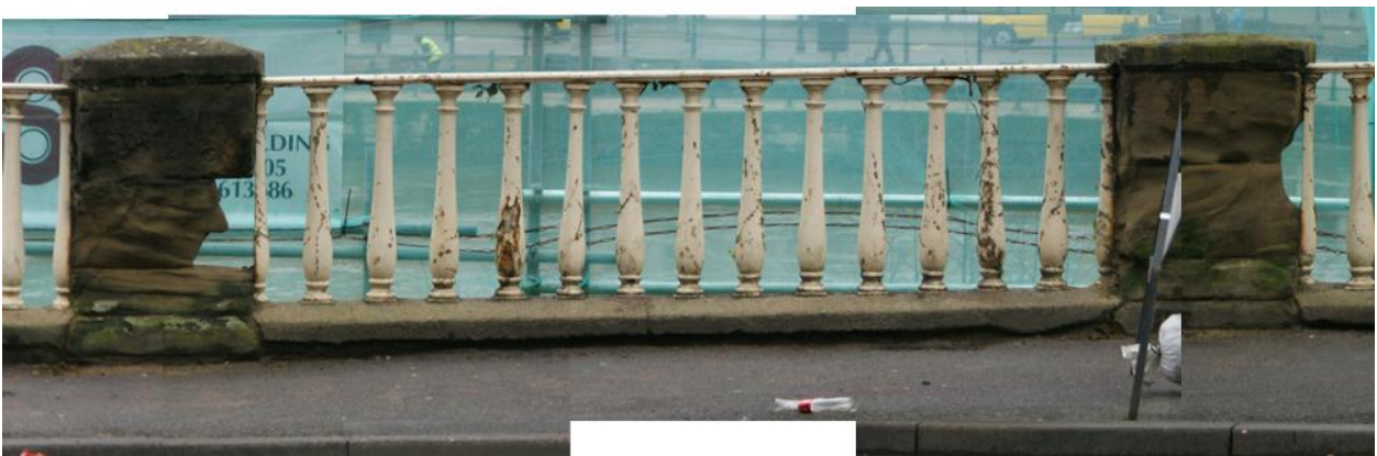
Plate 17: Bewdley Bridge abutment road side, pier 3 (on left) to 2
