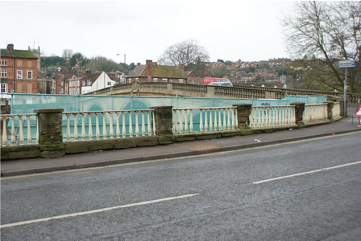
Plate 1: Road side elevation of Bewdley Bridge abutment (pier 6 on the left)
