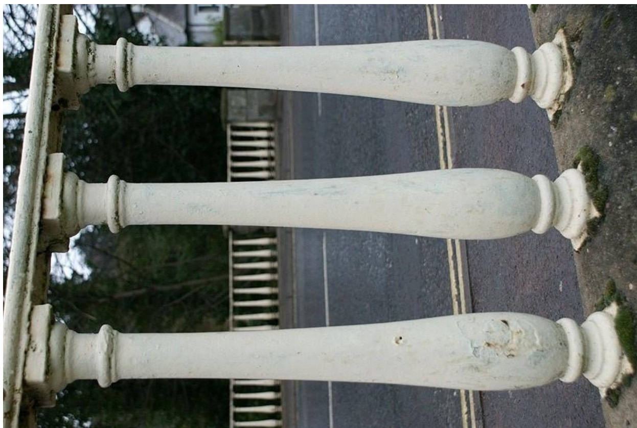
Plate 13: Detail of cast iron balusters on Bewdley Bridge abutment
