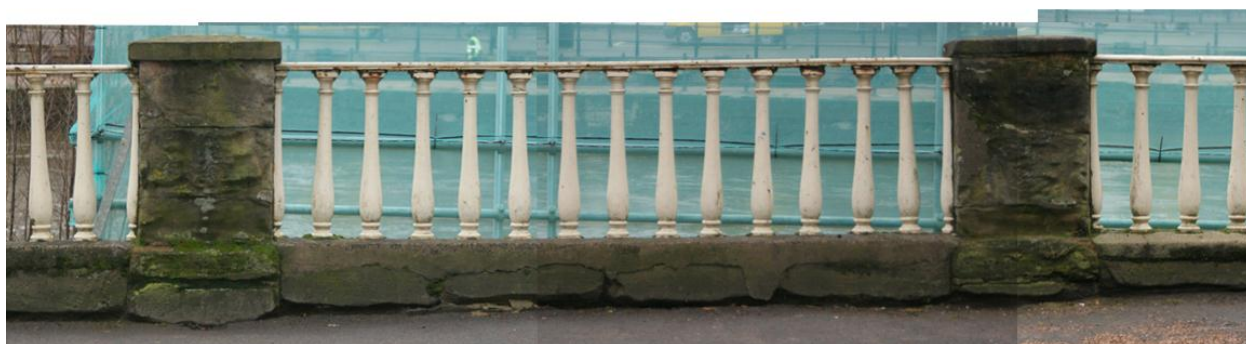
Plate 14: Bewdley Bridge abutment road side, pier 6 (on left) to 5
