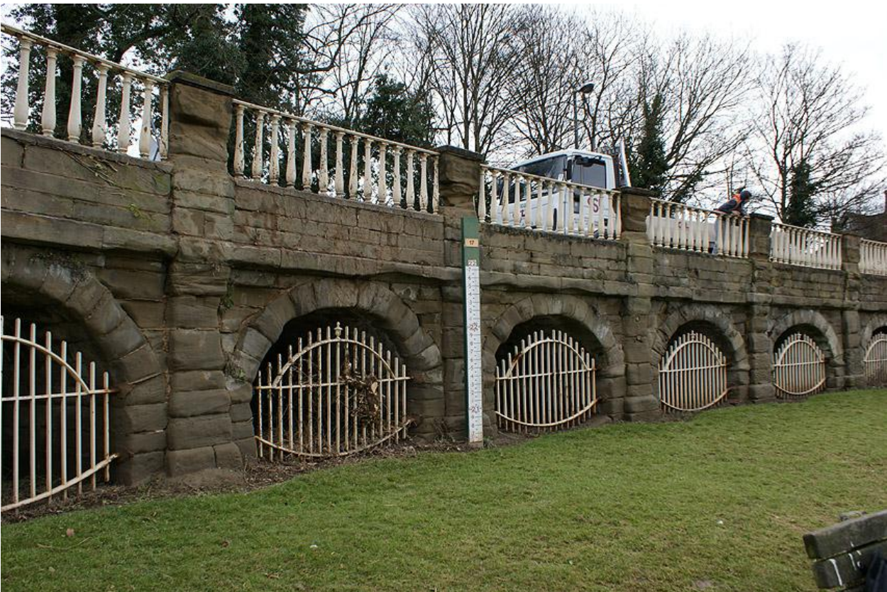
Plate 2: River side elevation of Bewdley Bridge abutment (pier 2 on the left)
