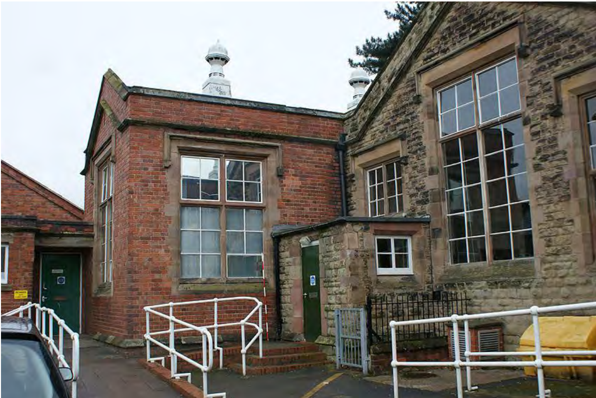
Plate 33: Classroom extension from the west
