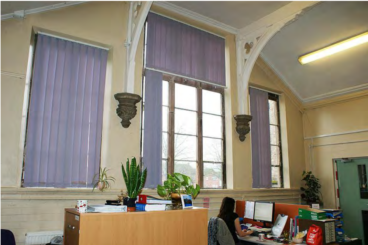
Plate 31: Interior detail of 1907 classroom
