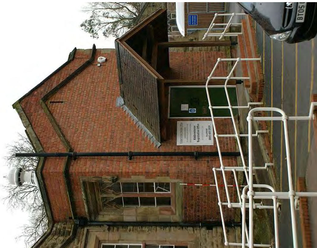
Plate 24: Classroom wing extension from the north
