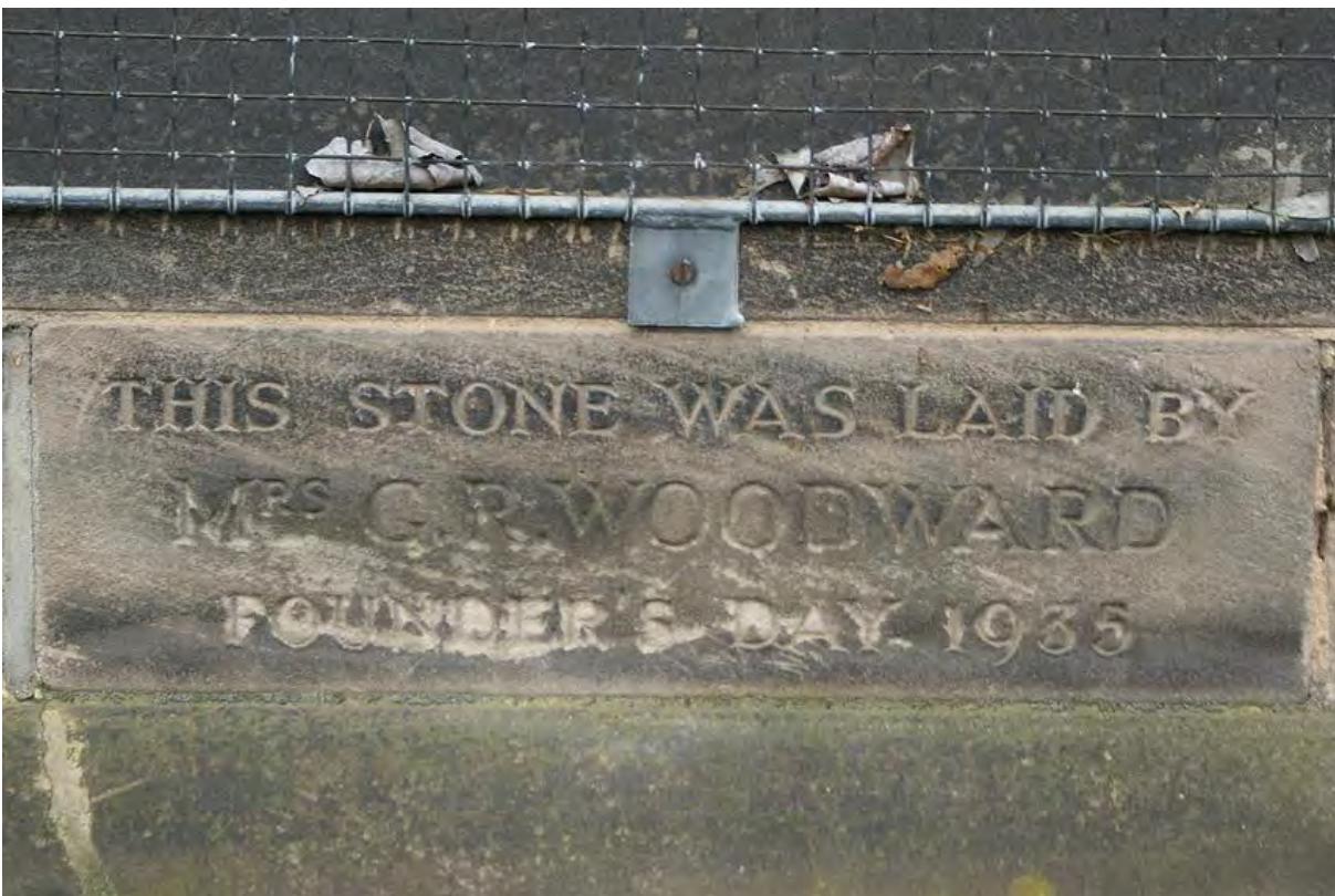
Plate 42: Foundation stone on library gable
