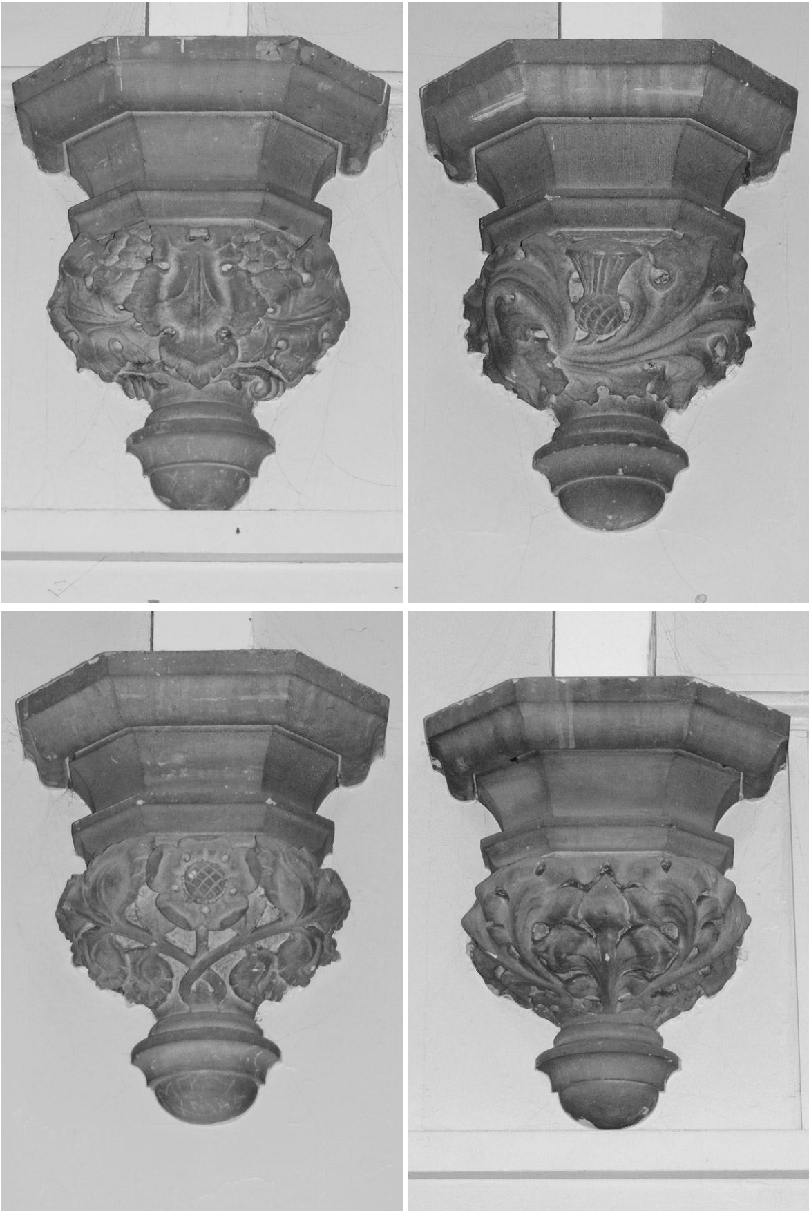
Plate 32: Interior corbel details
