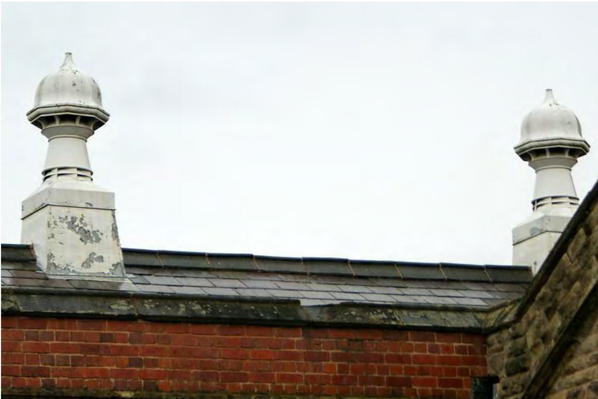
Plate 9: Finial roof vents
