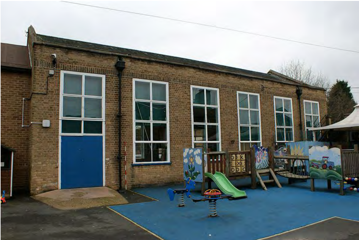
Plate 15: The hall wing of the 1938 school building from the south east
