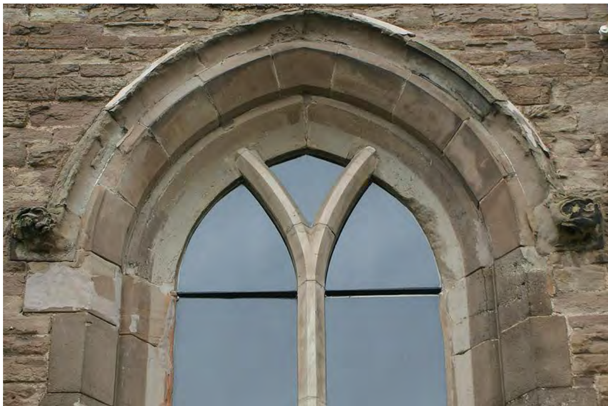
Plate 3: Hood mould and finials on window
