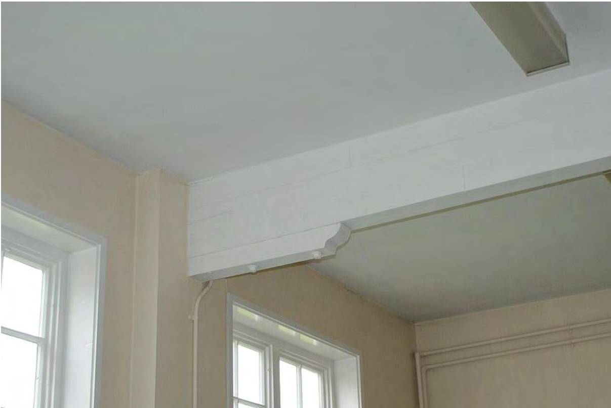
Plate 41: Former fives court roof truss
