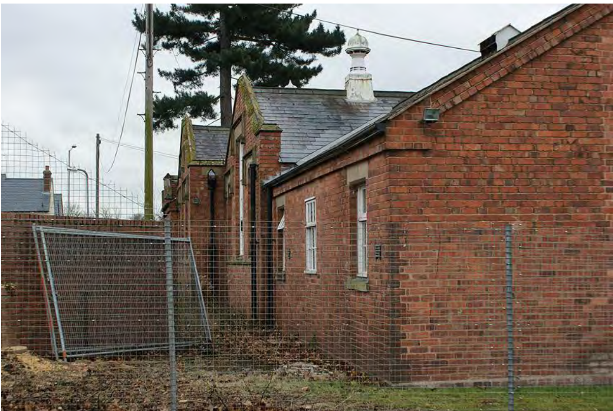
Plate 34: Simple brick extension from the north east
