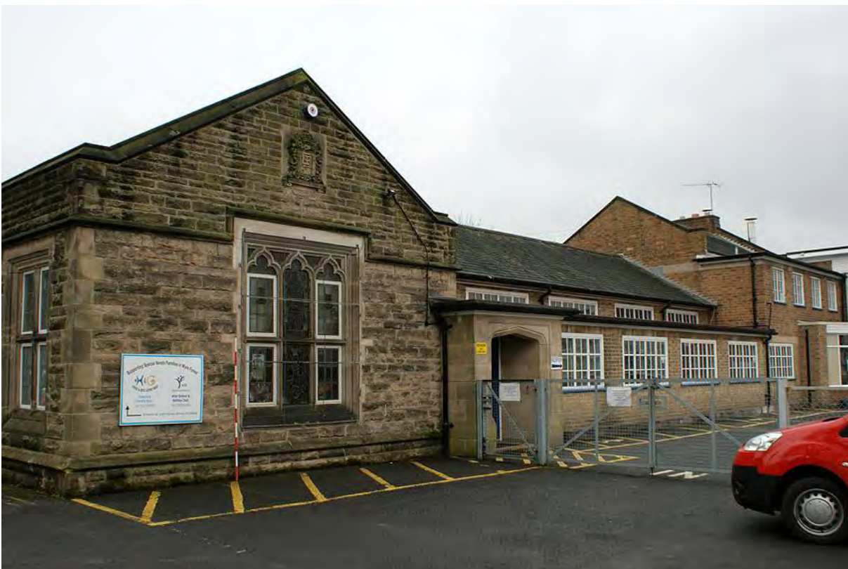
Plate 14: The library wing of the 1938 school building from the south east
