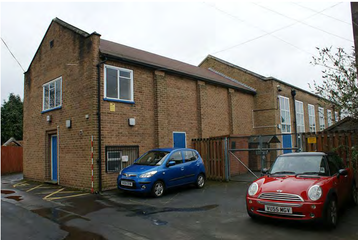
Plate 48: Swimming pool extension from the south east
