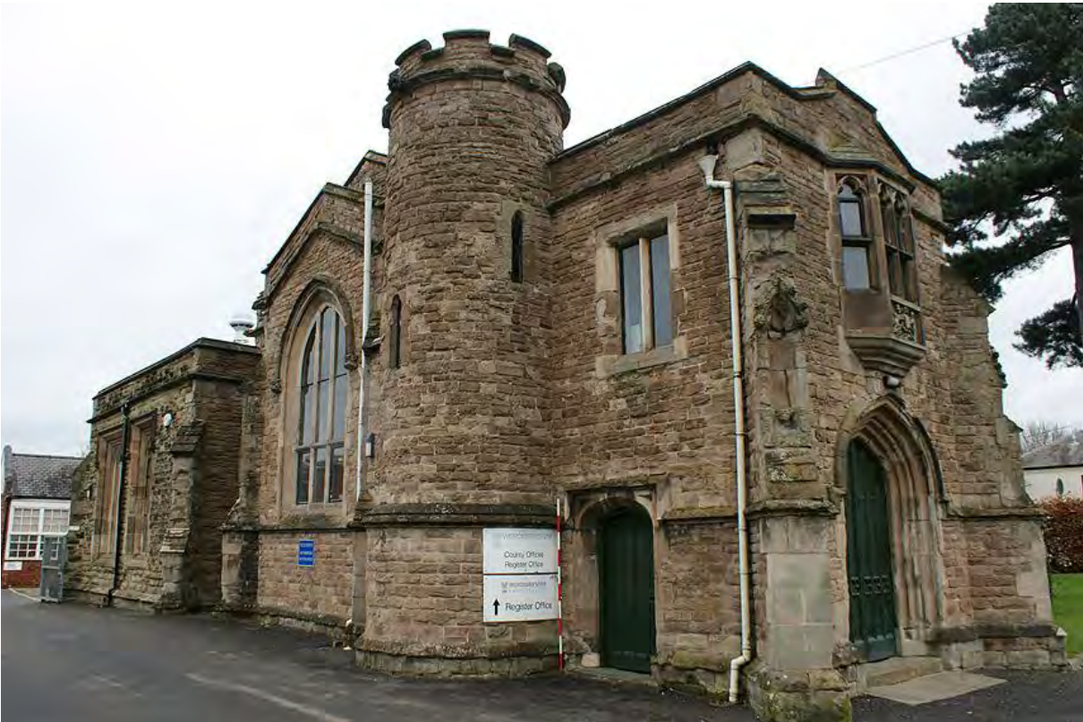
Plate 19: West elevation of 1848 school building showing castellated tower
