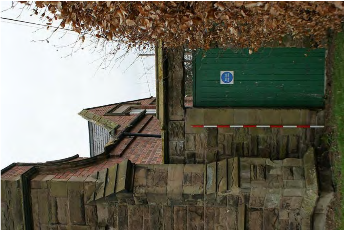
Plate 29: 1907 classroom from the south east
