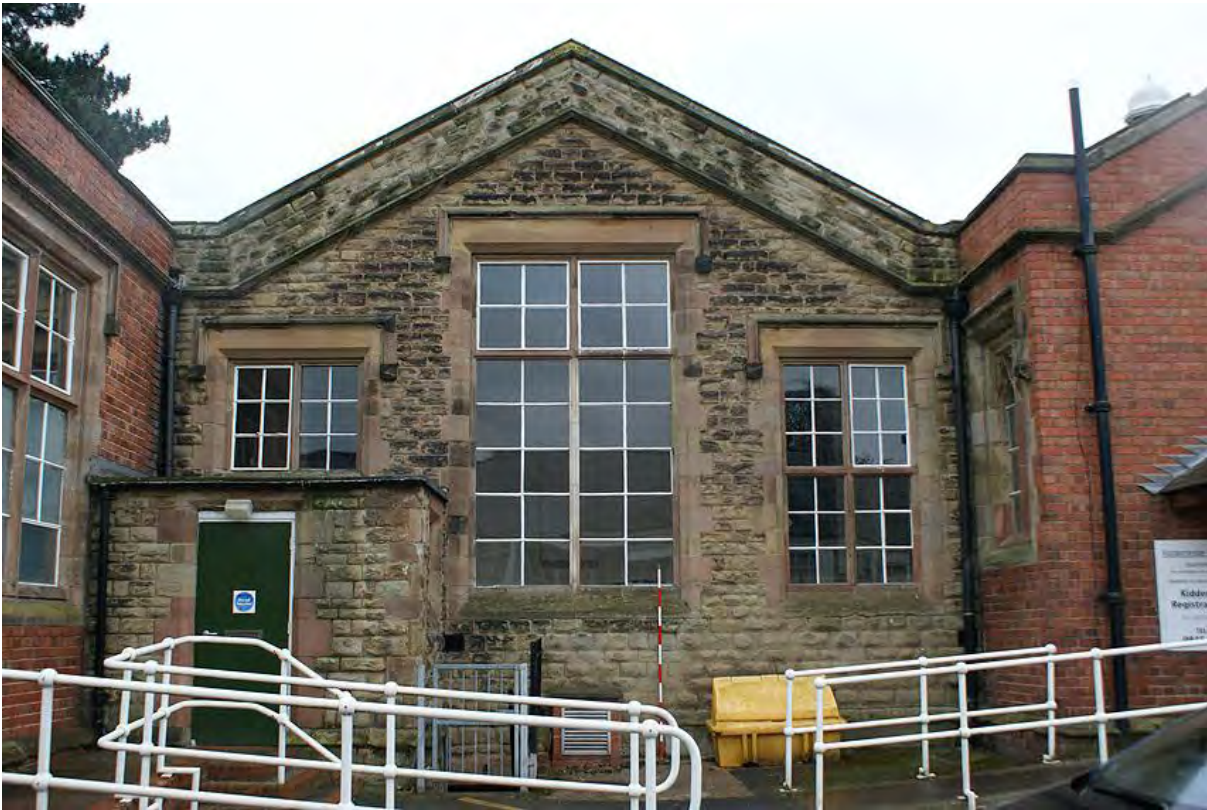
Plate 25: Room adjoining classroom wings
