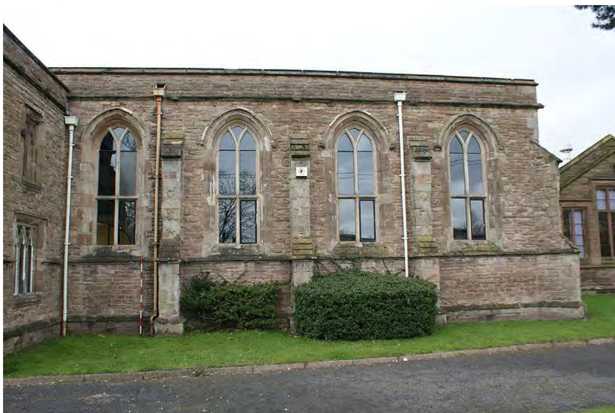
Plate 2: Windows of 1848 building from south east
