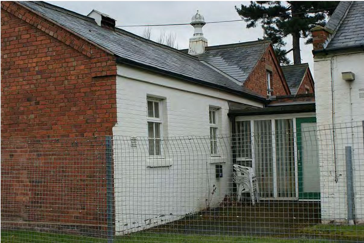
Plate 35: Simple brick extension from the north west
