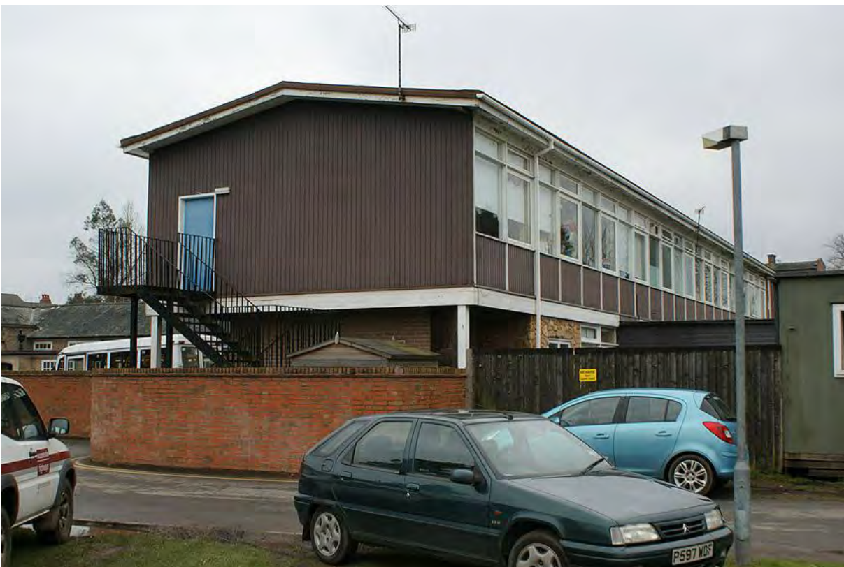
Plate 46: Two-storey classroom range from the north east
