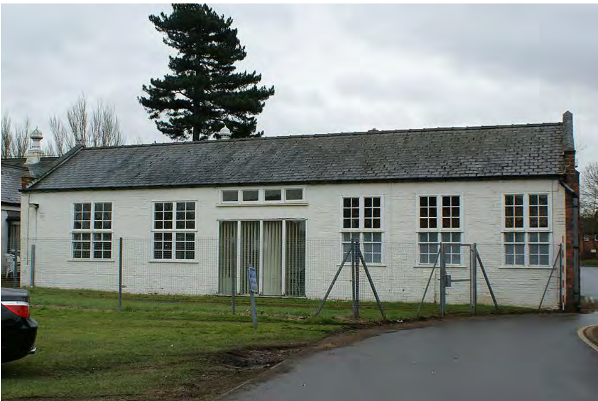
Plate 26: Fives court from the north west
