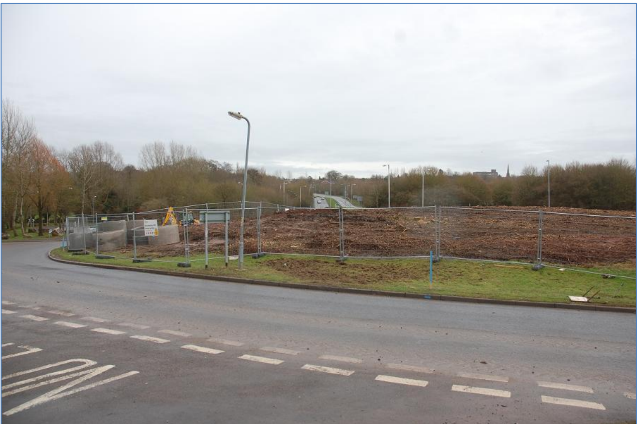
Plate 4 General shot of site location.
