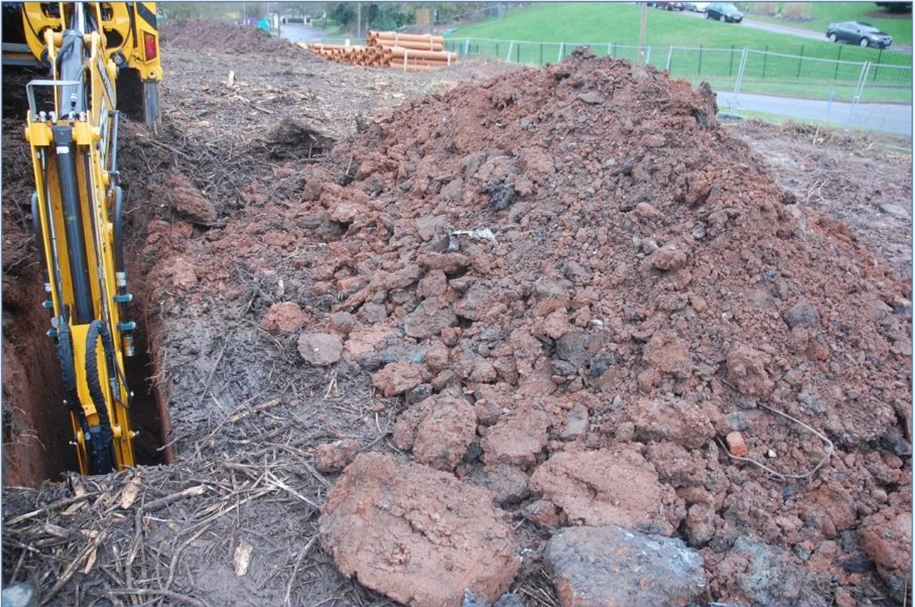
Plate 3 Mixed Mercian mudstone and 20 th Century demolition material from Trial Hole 2, view northeast
