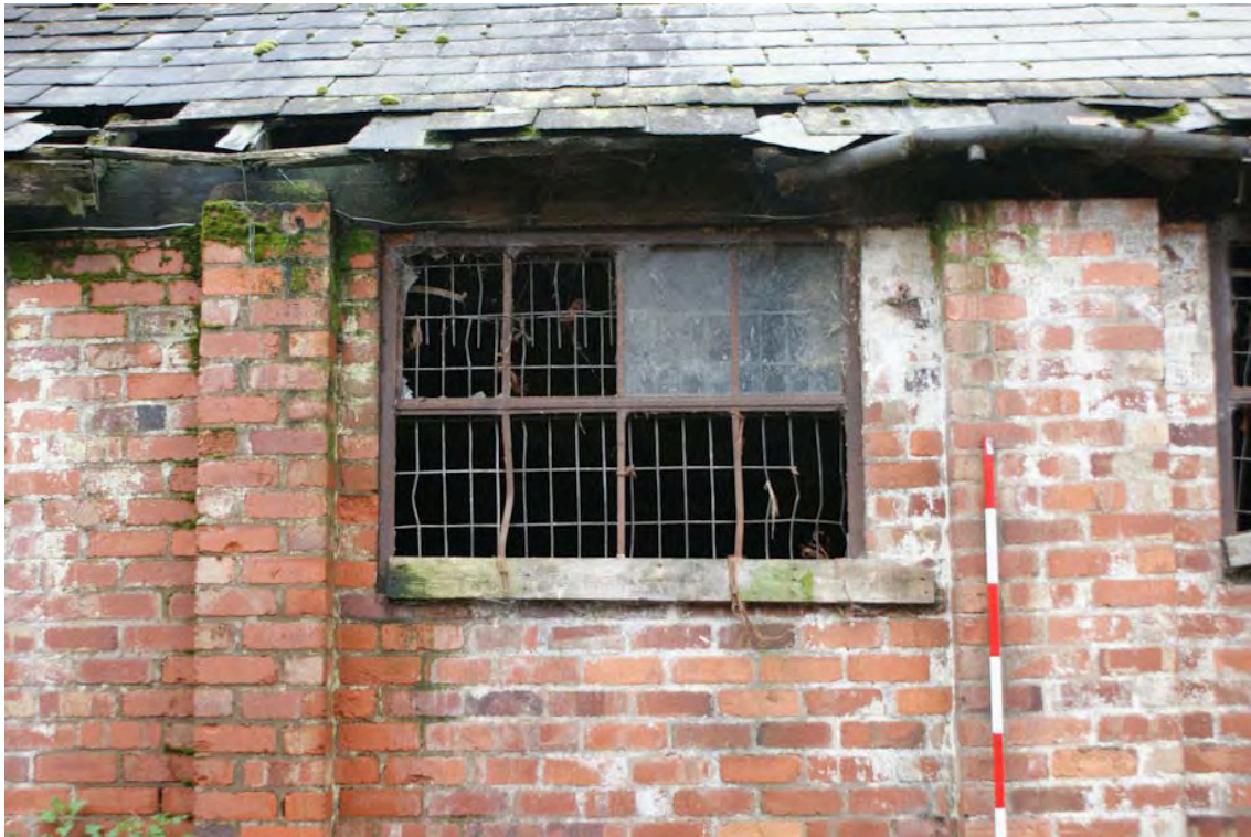
Plate 34: Detail of the window and pilasters in Building 5
