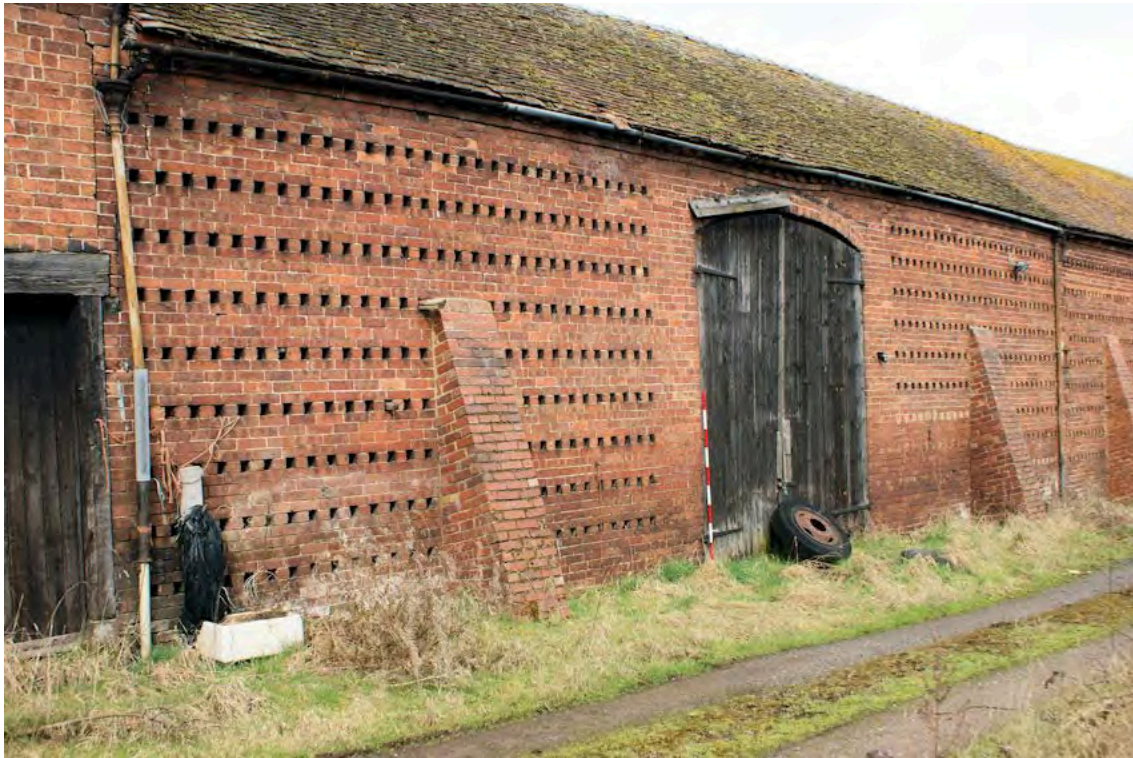
Plate 14: South east elevation of the 19 th century threshing barn, Building 6
