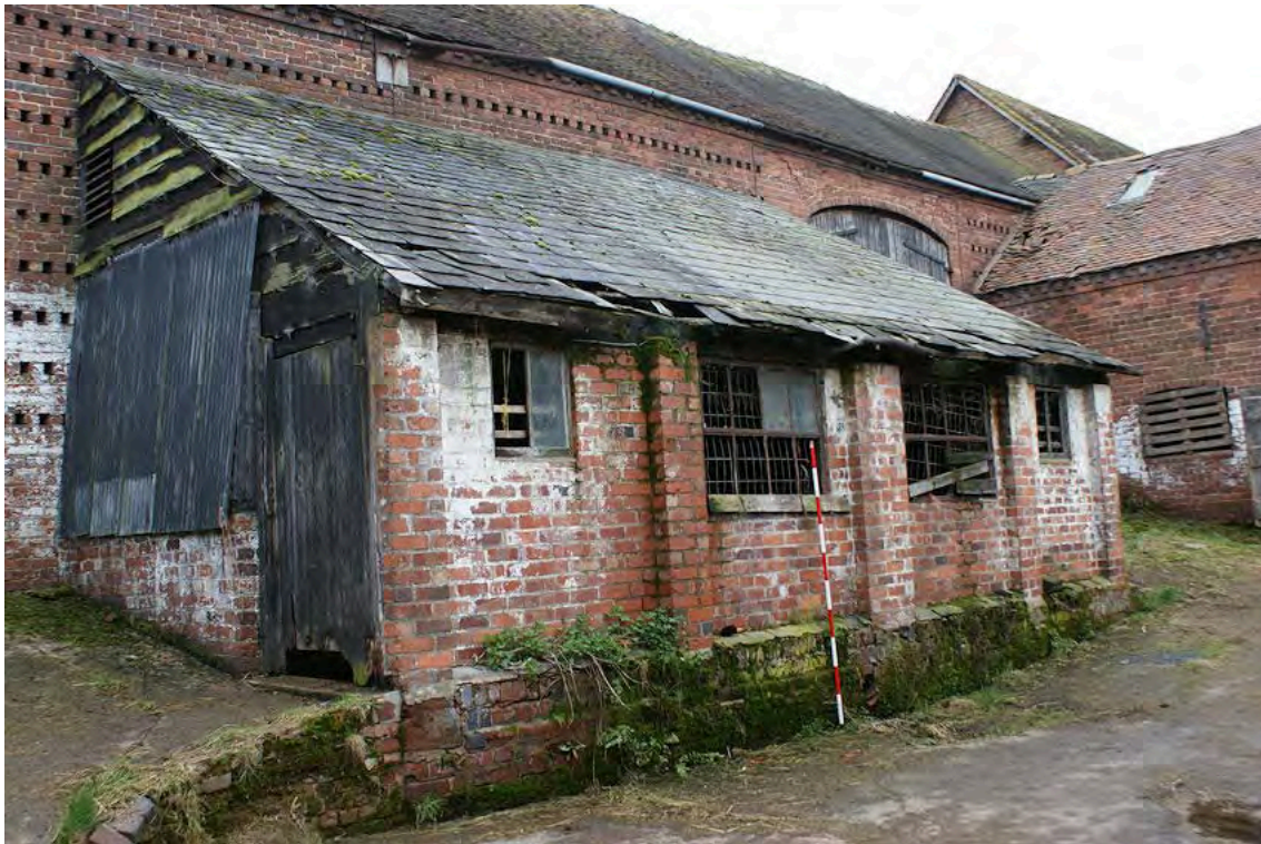
Plate 33: North west elevation of Building 5
