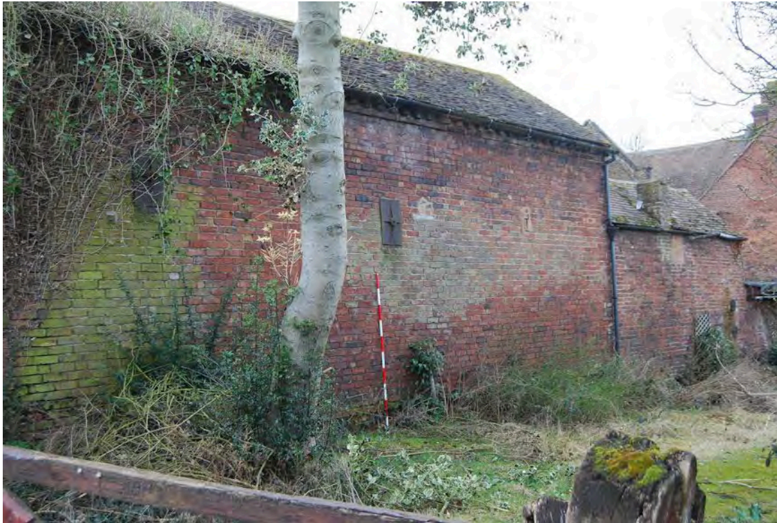
Plate 5: North east elevation of Building 2
