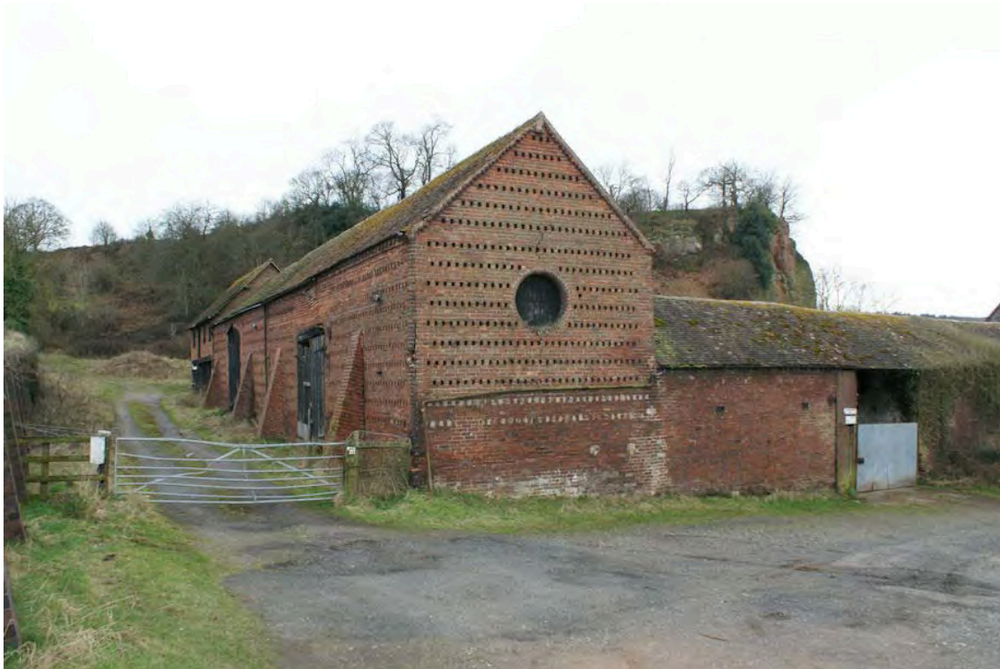
Plate 49: The south eastern elevation of Buildings 4 and 6, with early 20 th century buttresses
