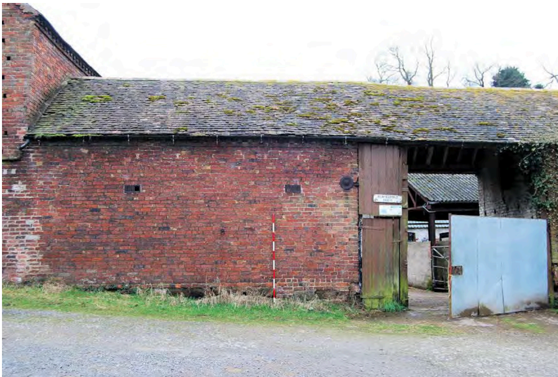
Plate 6: North east elevation of Building 3
