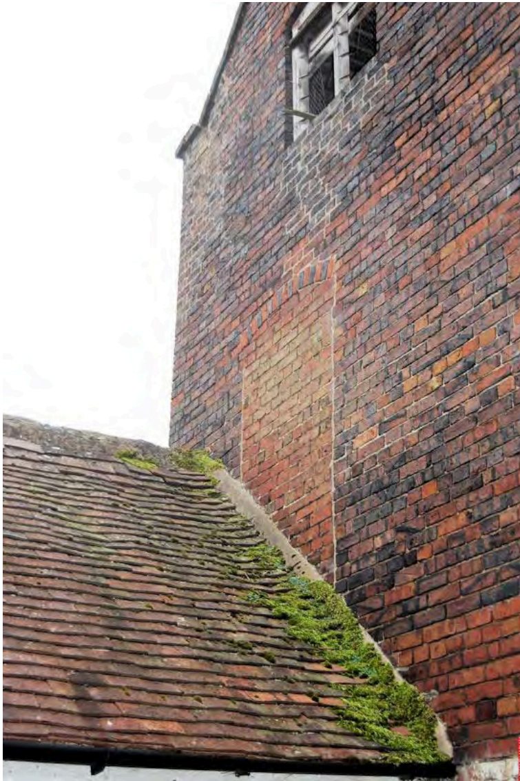
Plate 25: Blocked opening visible in the north west elevation of Building 10
