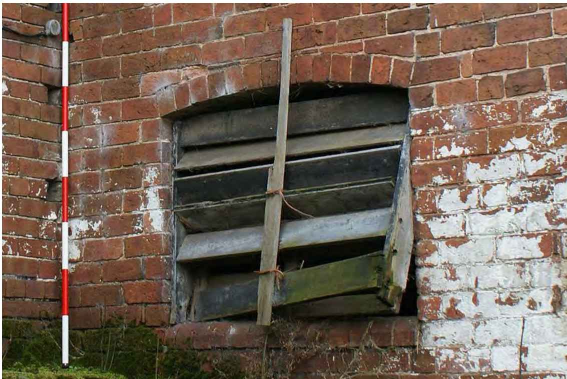
Plate 22: Example of the window including wooden louvers, Building 8
