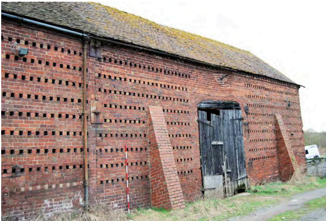
Plate 2: The south east elevation of threshing barn, Building 4
