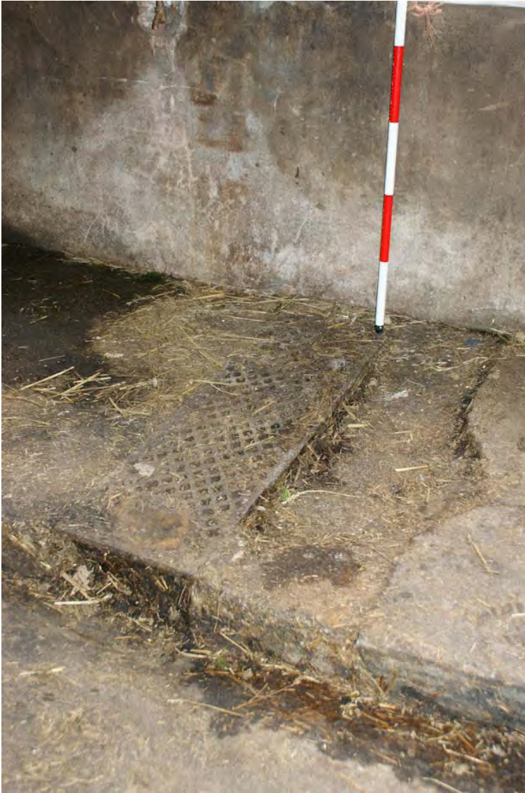
Plate 35: View of the internal effluent drainage channel within Building 5
