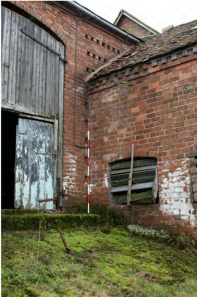
Plate 20: The building break between the two structures, Building 6 and 8
