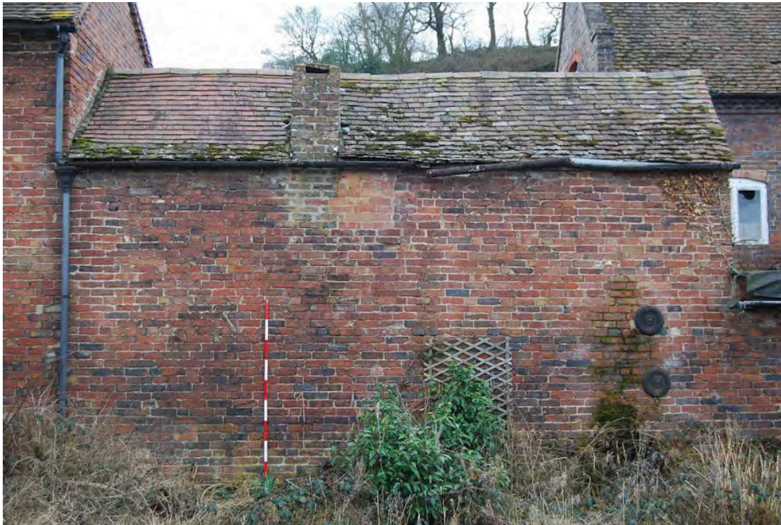
Plate 17: North east elevation of Building 1
