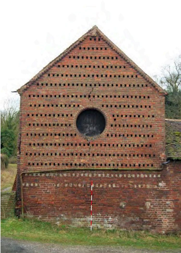
Plate 4: North east elevation of Building 4, including pitching eye
