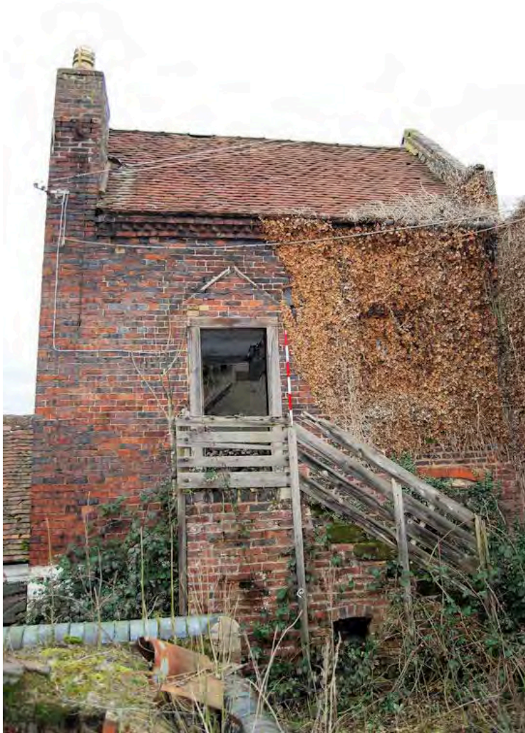
Plate 23: South west elevation of 19 th century Building 10
