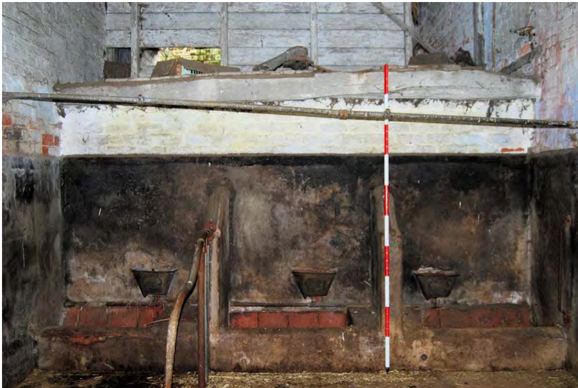
Plate 37: Internal view of Building 10, stables
