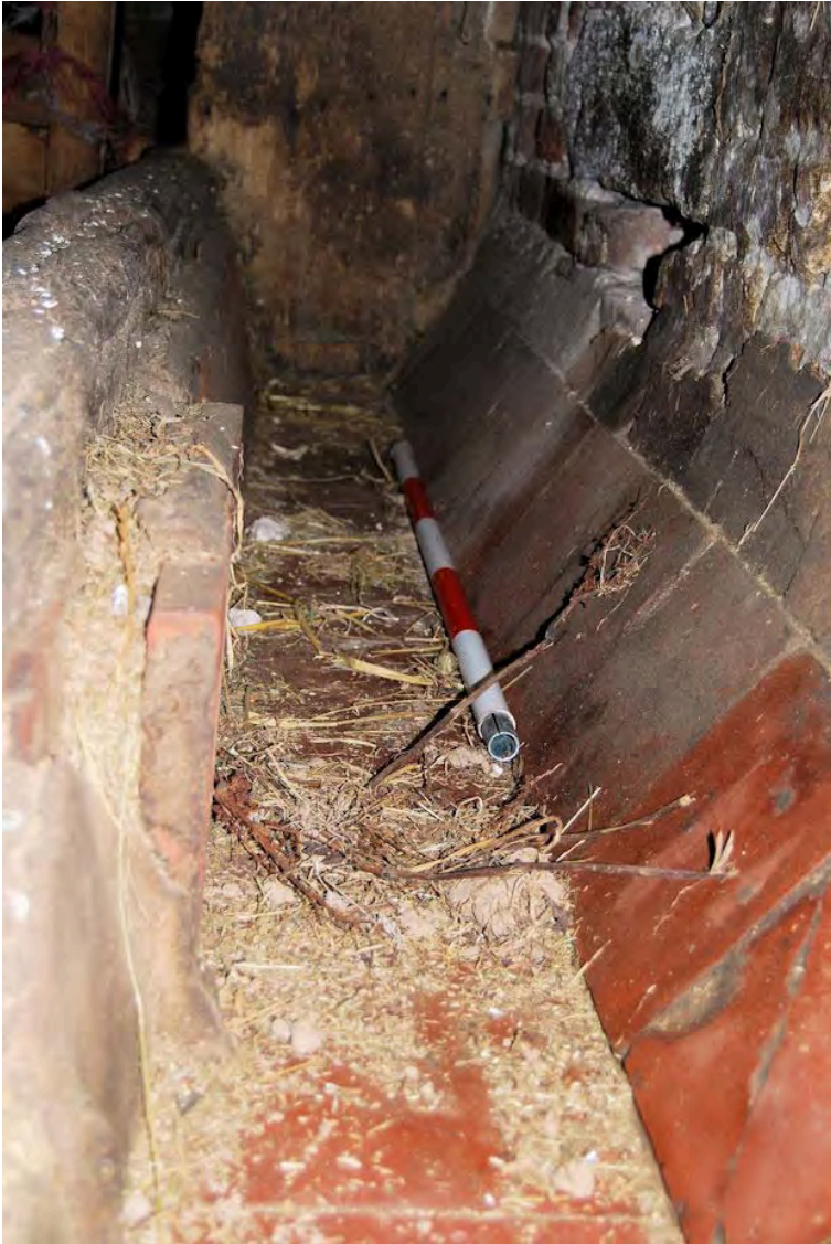
Plate 11: Example of the ceramic tiles lining the feeding trough, Building 2
