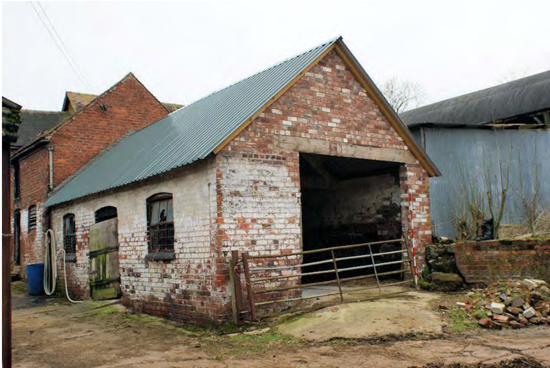
Plate 26: Building 9, view south
