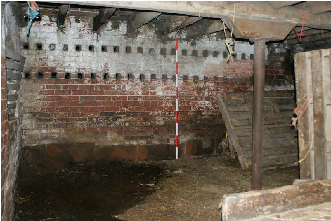
Plate 21: Brick piercing, interior of Building 8, north west elevation of Building 6
