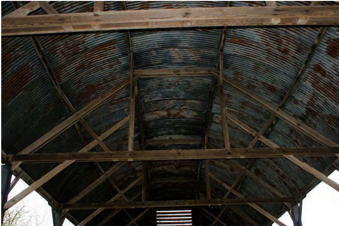
Plate 32: The internal view showing the queen-post construction of Building 12
