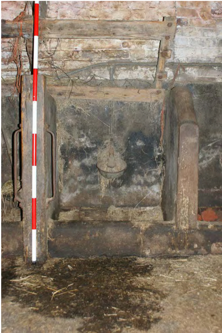
Plate 47: Example of the concrete trough and stalls with cast iron water pipes and bowls in Building 5
