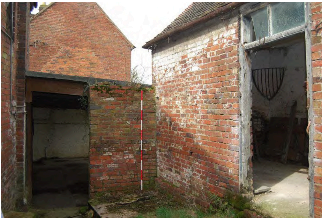
Plate 18: South west elevation of Building 1
