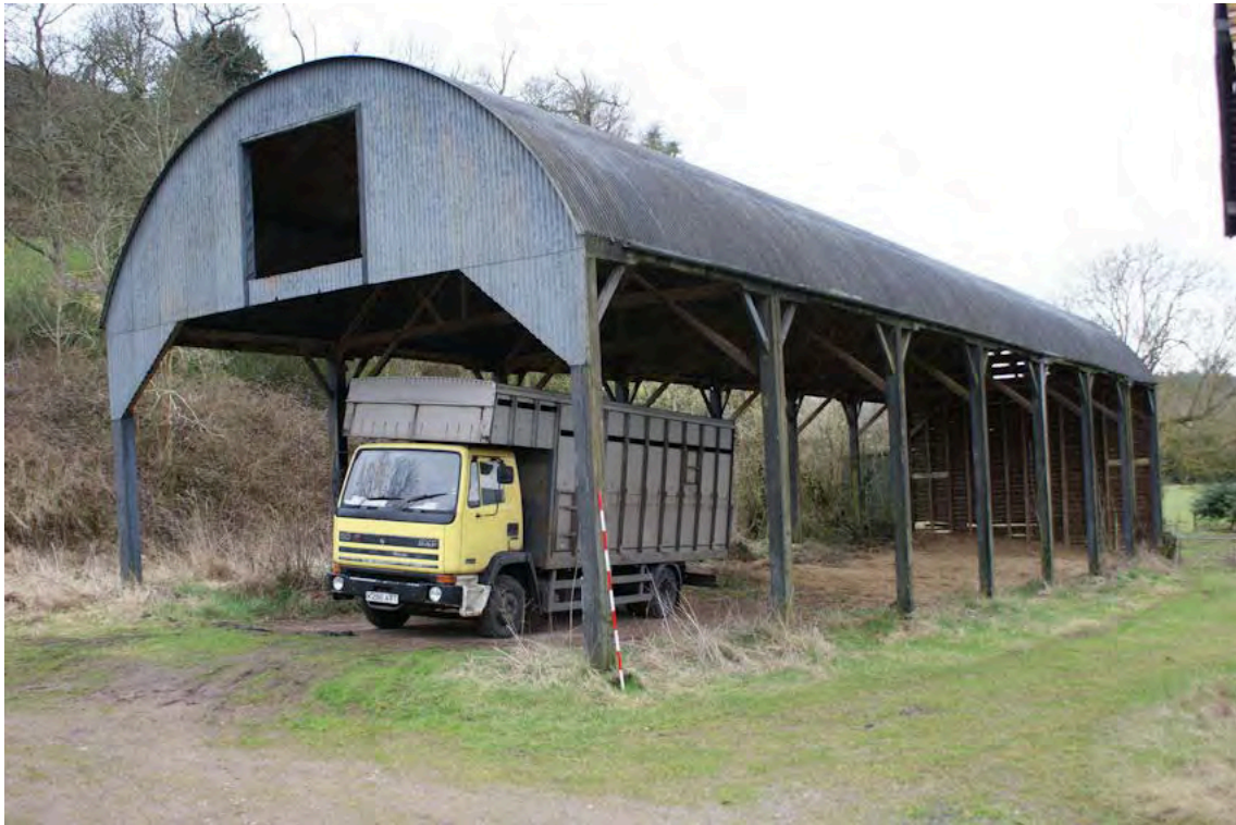
Plate 30: The Dutch barn, Building 12, view south
