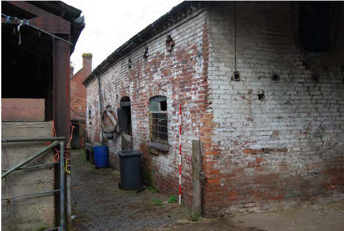
Plate 9: South west elevation of Building 2
