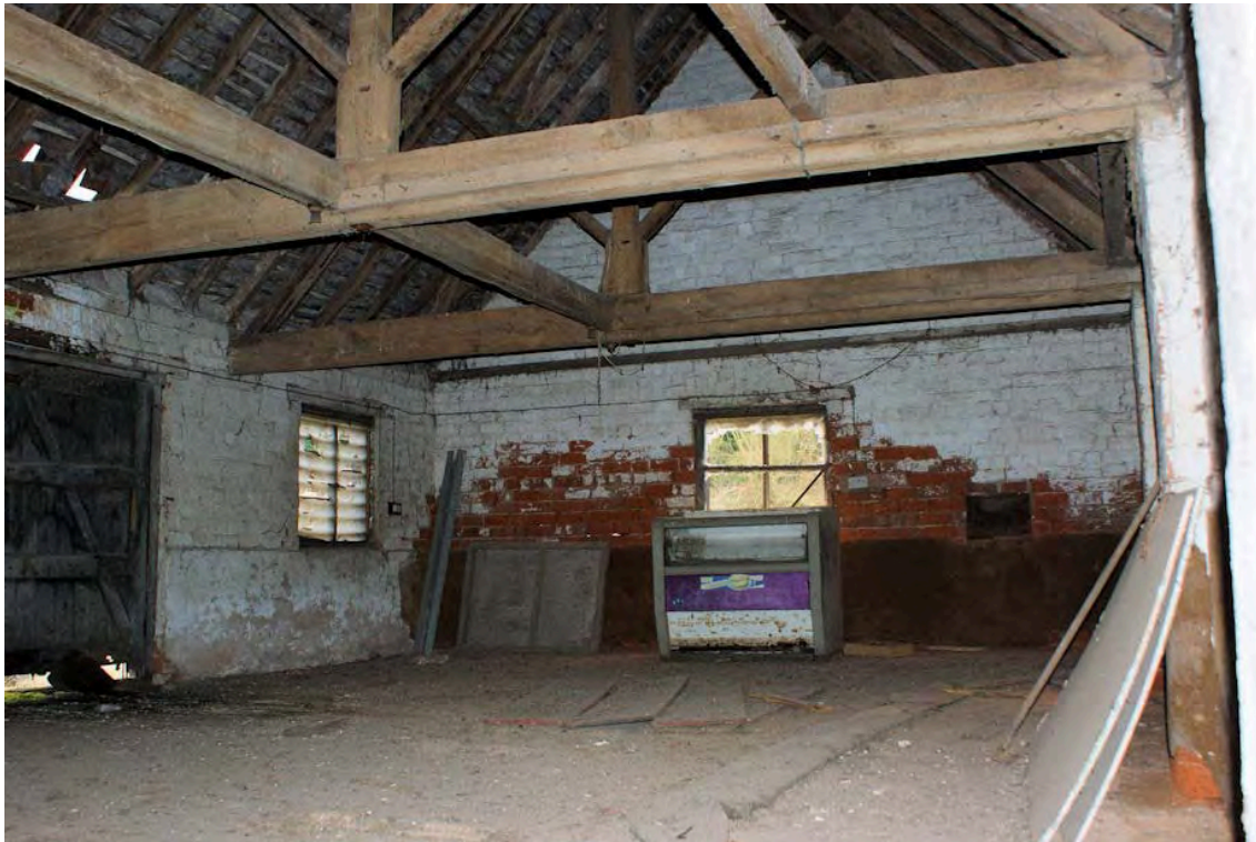
Plate 42: Granary above Cart shed (Building 7)
