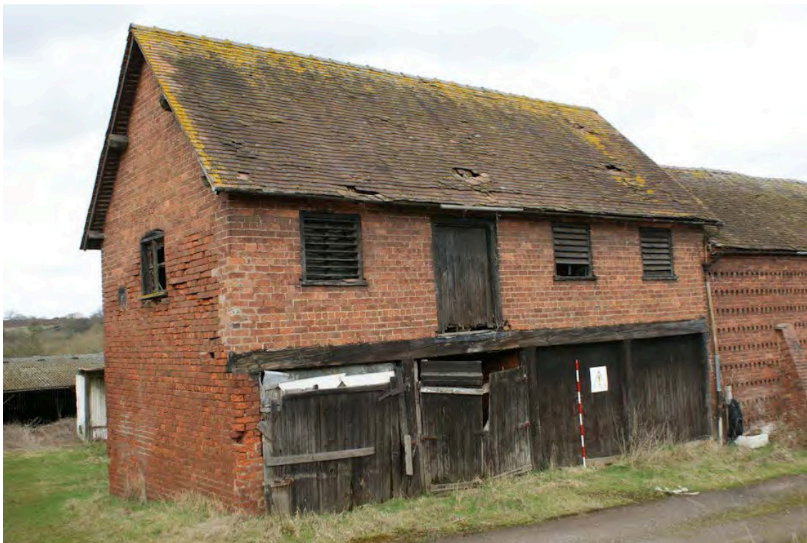
Plate 41: South east elevation of the cart shed (Building 7)
