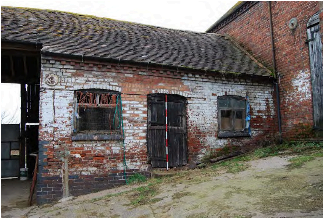
Plate 8: South west elevation of Building 3
