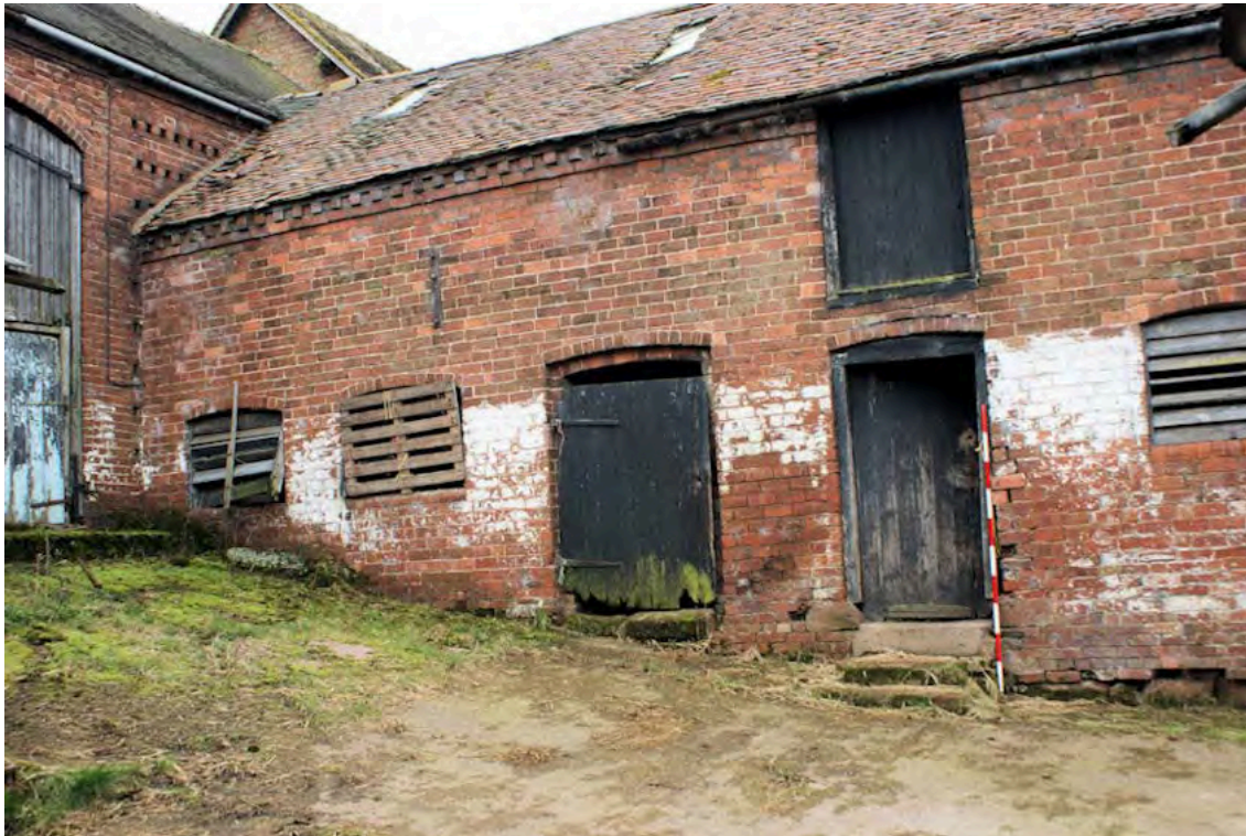
Plate 19: North east elevation of Building 8
