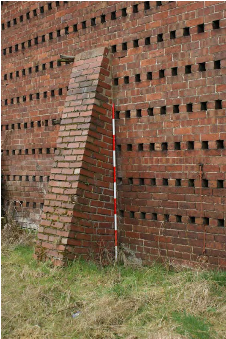
Plate 50: Detail of the buttress, Building 6
