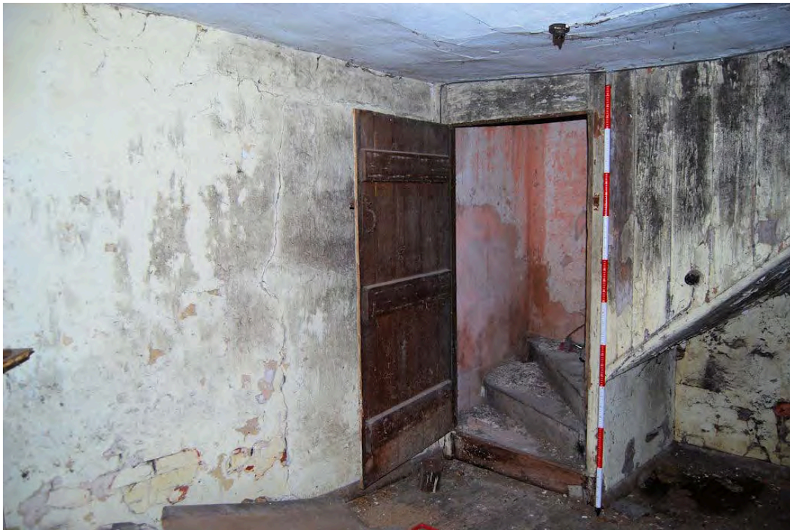
Plate 52: Staircase from the first to second floor within Building 10
