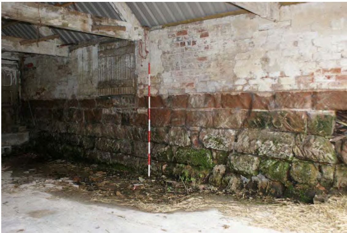
Plate 27: Detail of the construction technique used in Building 9, including large sandstone blocks
