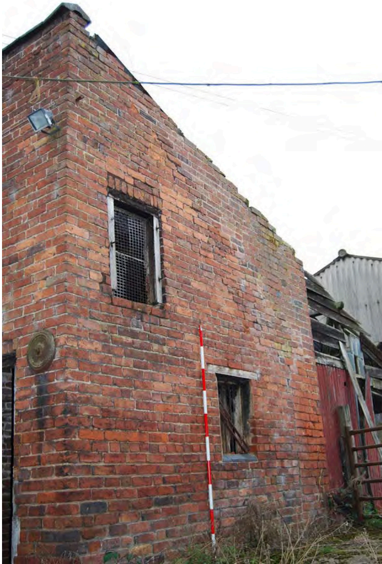
Plate 13: South west elevation of Building 10
