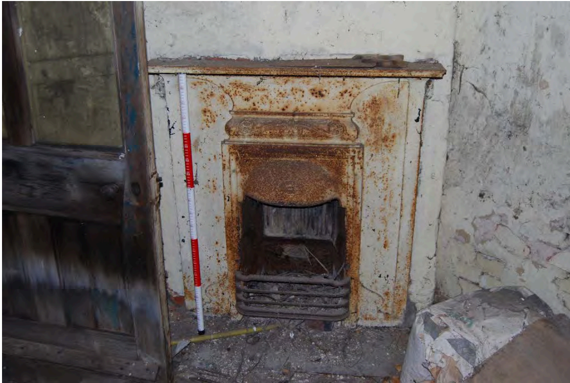
Plate 53: Detail of the first floor fireplace within Building 10
