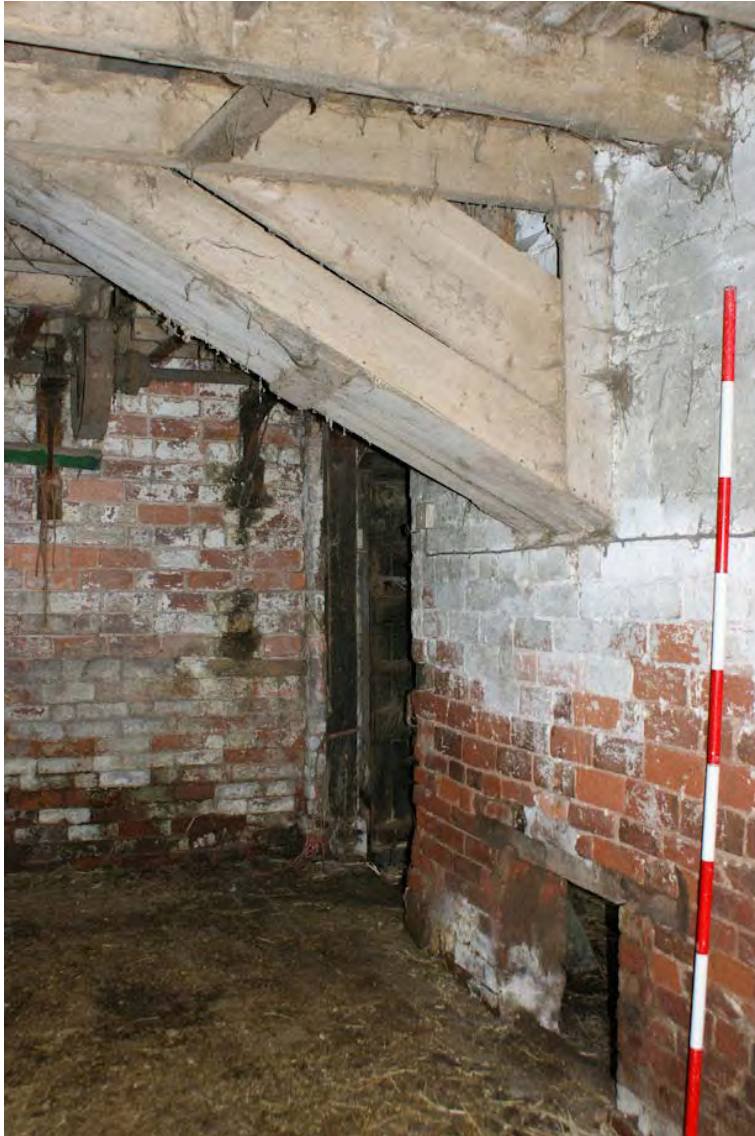
Plate 39: Internal view of Building 8 showing the chute to the adjacent building
