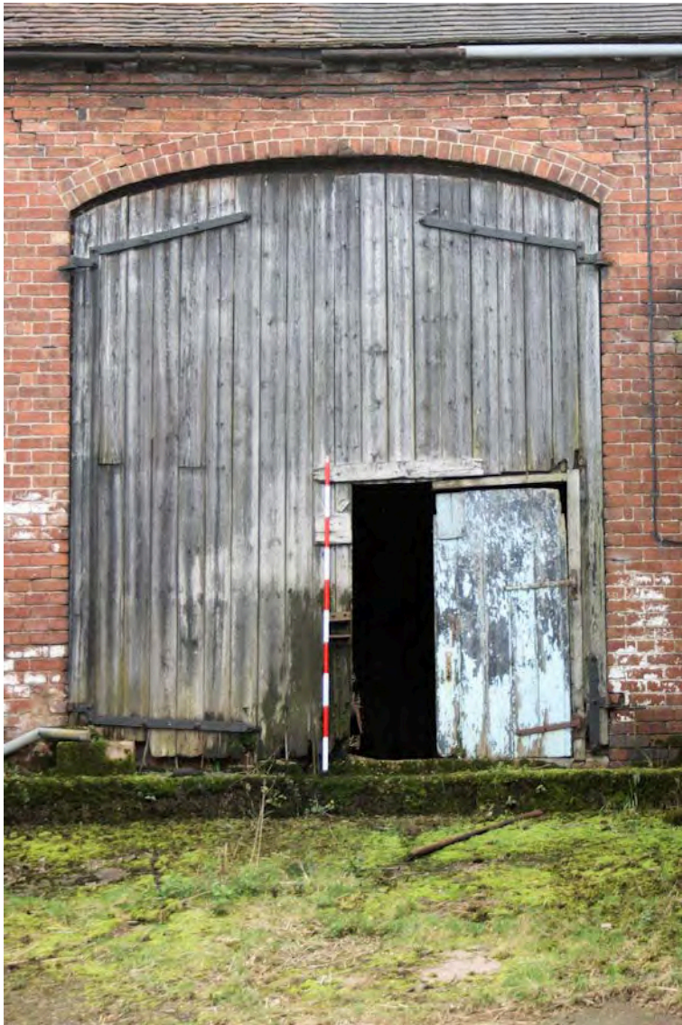
Plate 15 North west elevation of Building 6, including segmental arched opening
