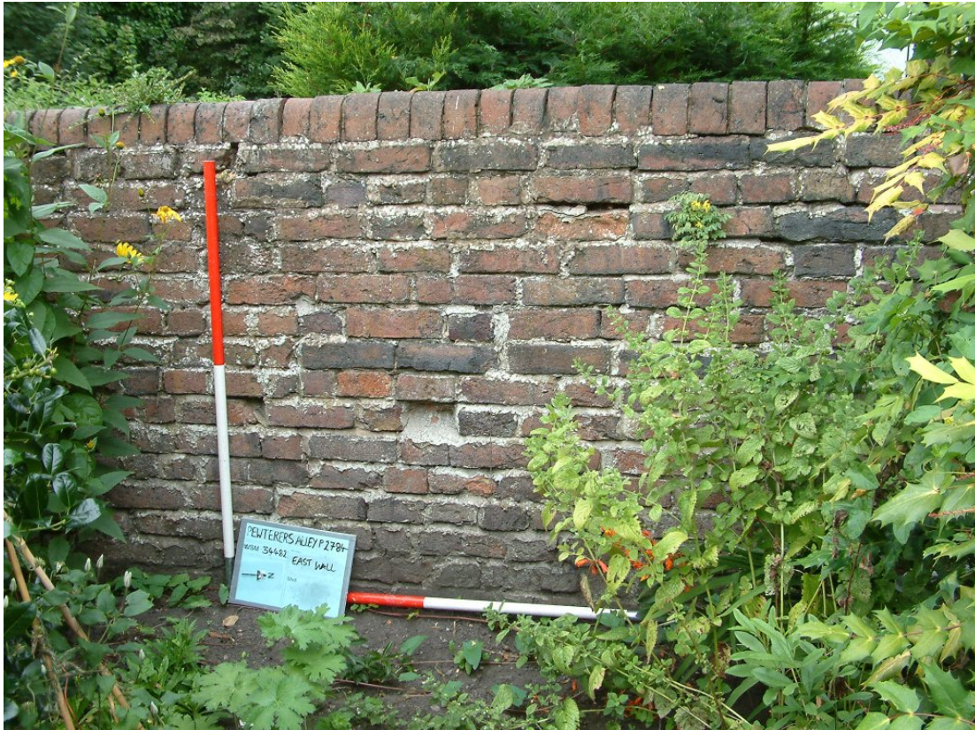
Plate 15 General shot of wall (see Figure 3 for location).
