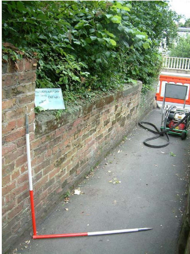
Plate 5 General shot of wall (see Figure 3 for location).
