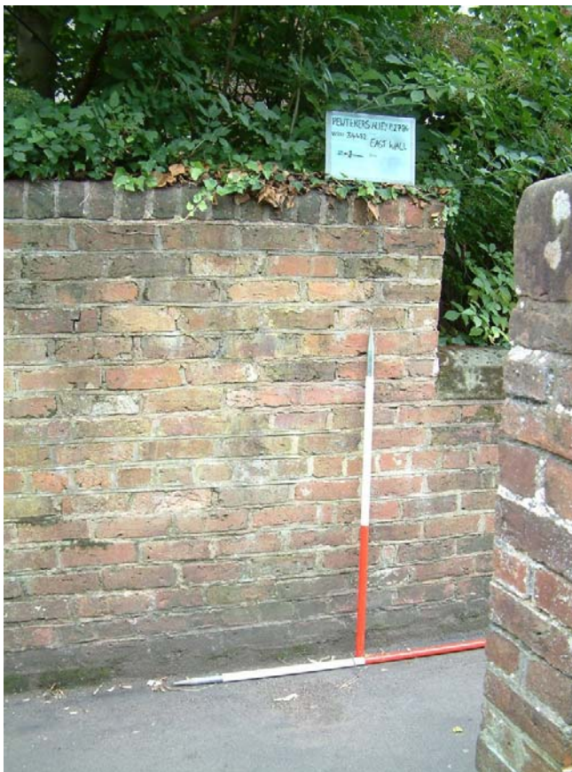
Plate 6 General shot of wall (see Figure 3 for location).
