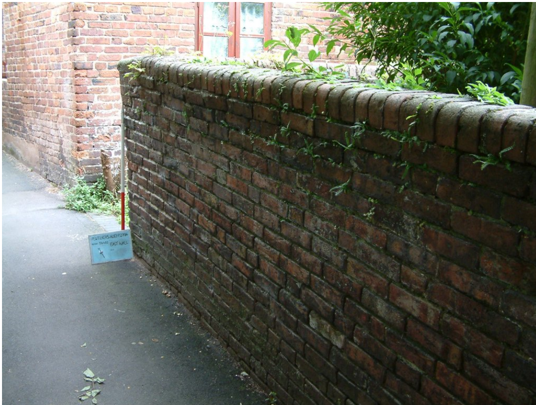
Plate 11 General shot of wall (see Figure 3 for location).
