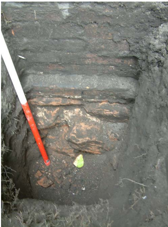
Plate 18 Sandstone foundation or early stone wall footings in test pit 2, facing north.
