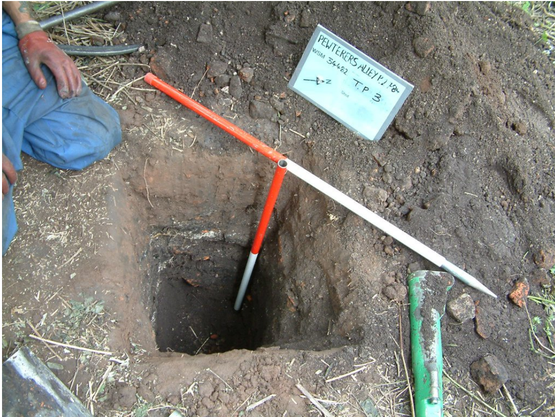
Plate 19 General shot of test pit 3, facing north west.
