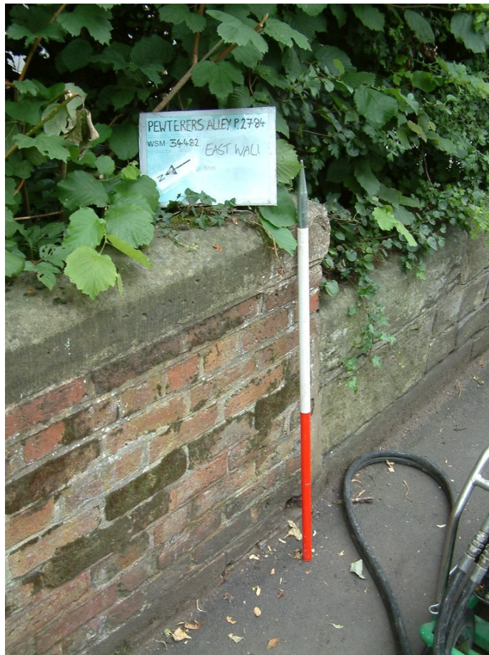
Plate 2 General shot of wall (see Figure 3 for location).
