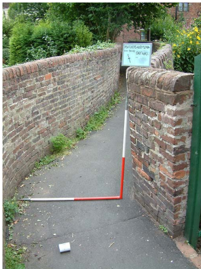
Plate 8 General shot of wall (see Figure 3 for location).
