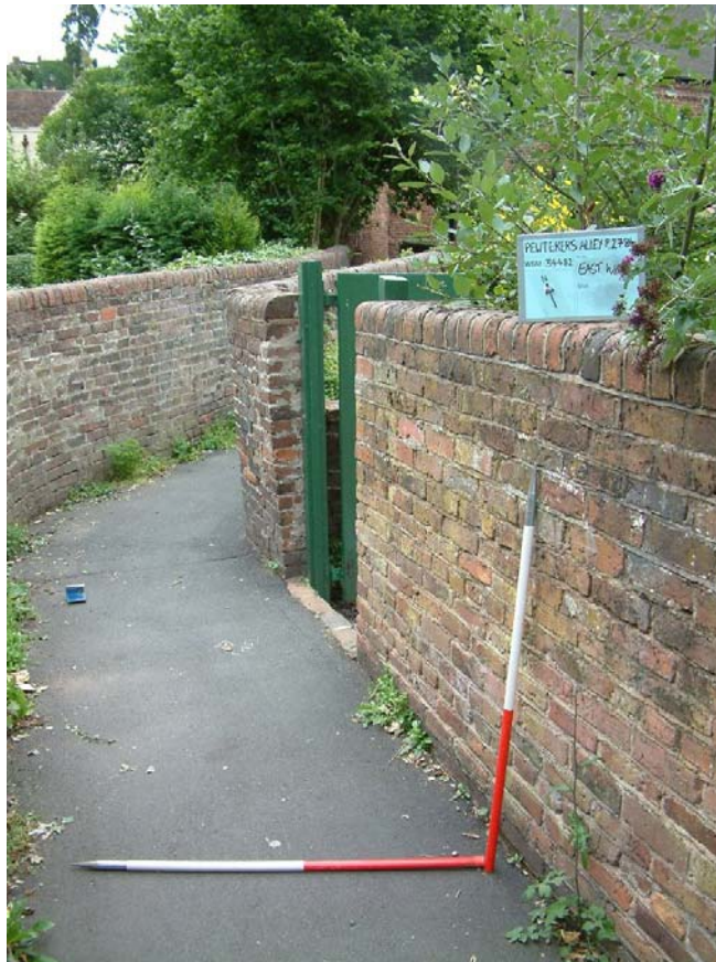
Plate 7 General shot of wall (see Figure 3 for location).
