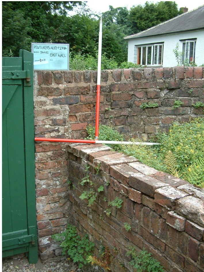
Plate 13 General shot of wall (see Figure 3 for location).
