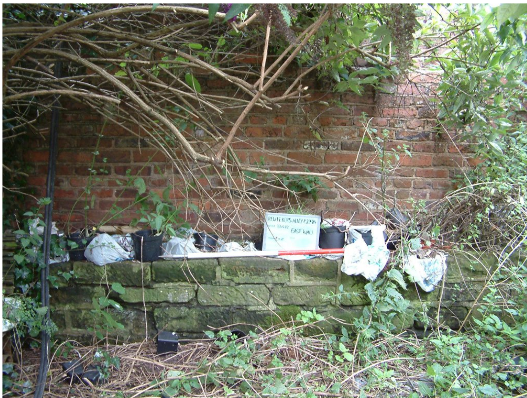
Plate 4 General shot of wall (see Figure 3 for location).
