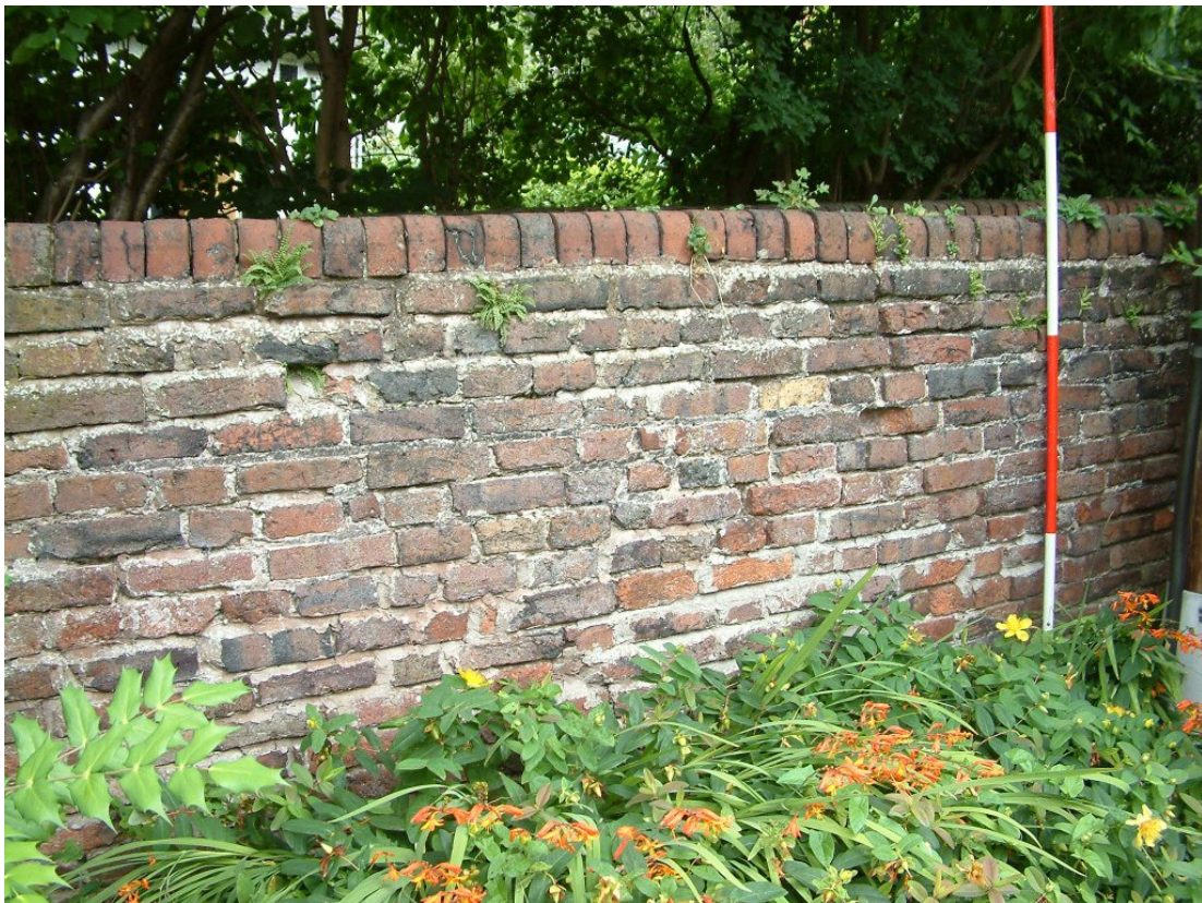
Plate 16 General shot of wall (see Figure 3 for location).
