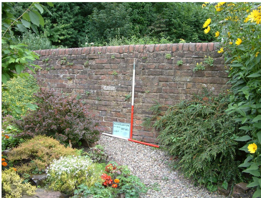
Plate 14 General shot of wall (see Figure 3 for location).
