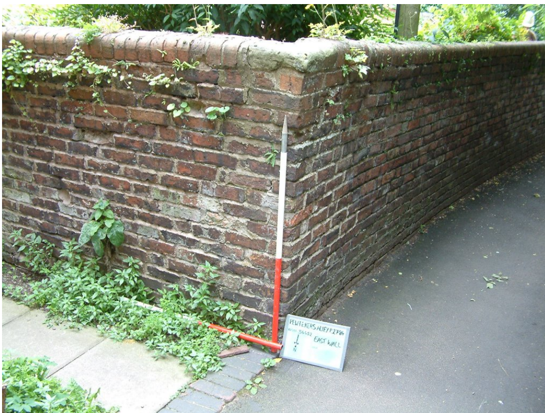
Plate 12 General shot of wall (see Figure 3 for location).
