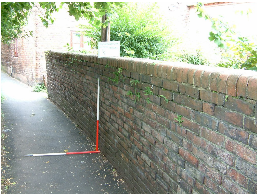
Plate 10 General shot of wall (see Figure 3 for location).
