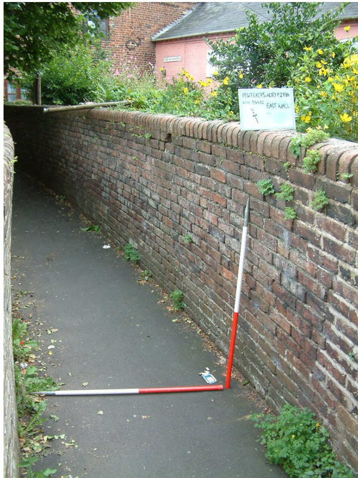
Plate 9 General shot of wall (see Figure 3 for location).
