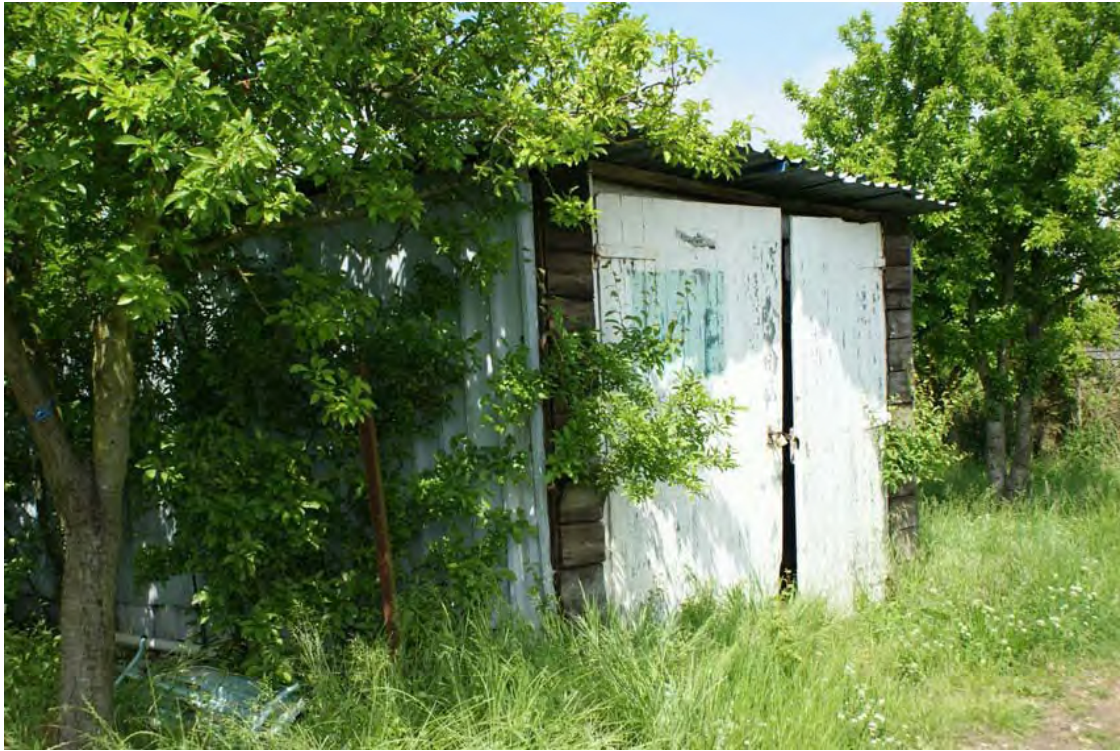
Plate 7: One of the wooden sheds
