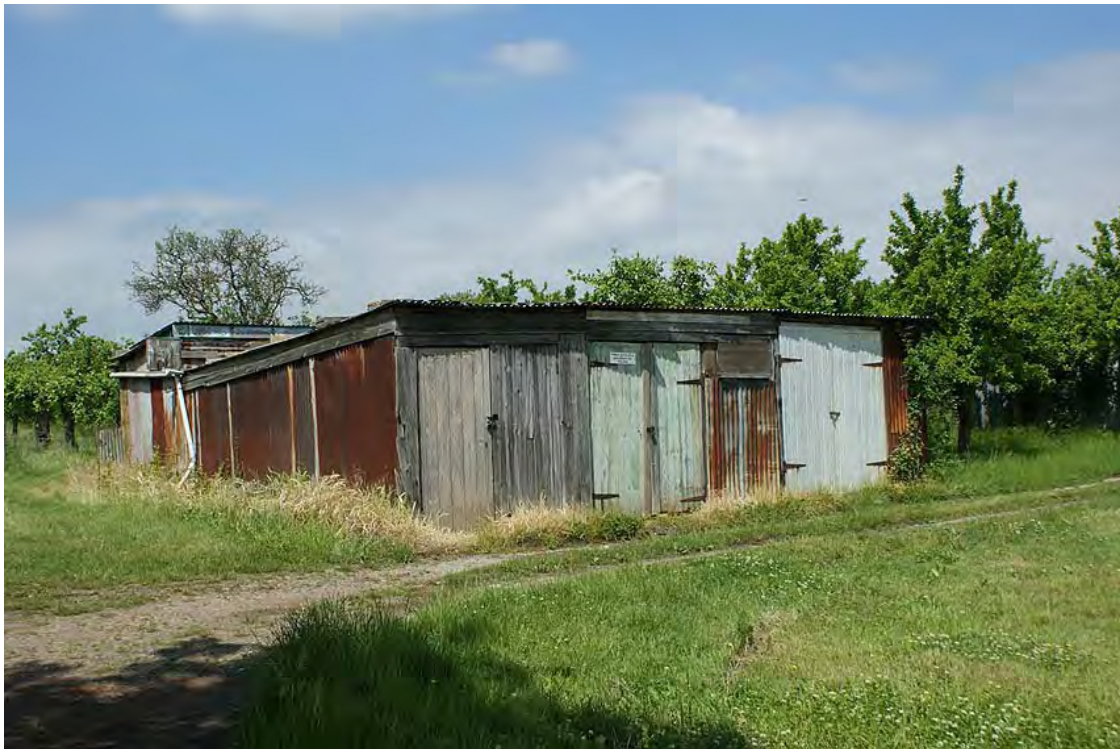
Plate 6: One of the tin sheds
