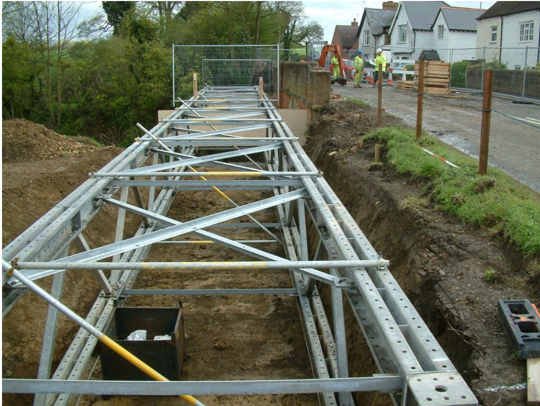
Plate 1: Trench 1 facing north-east
