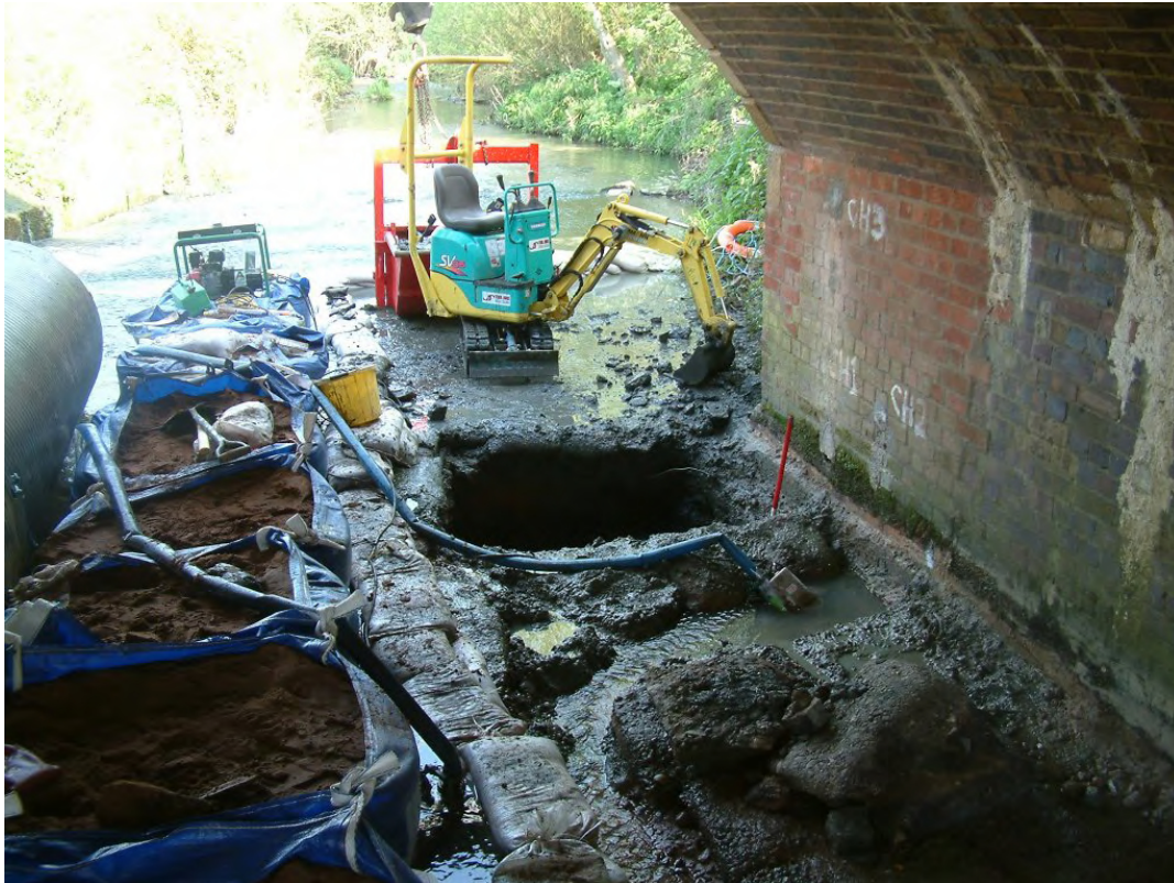
Plate 3: Trench 2 beneath east abutment
