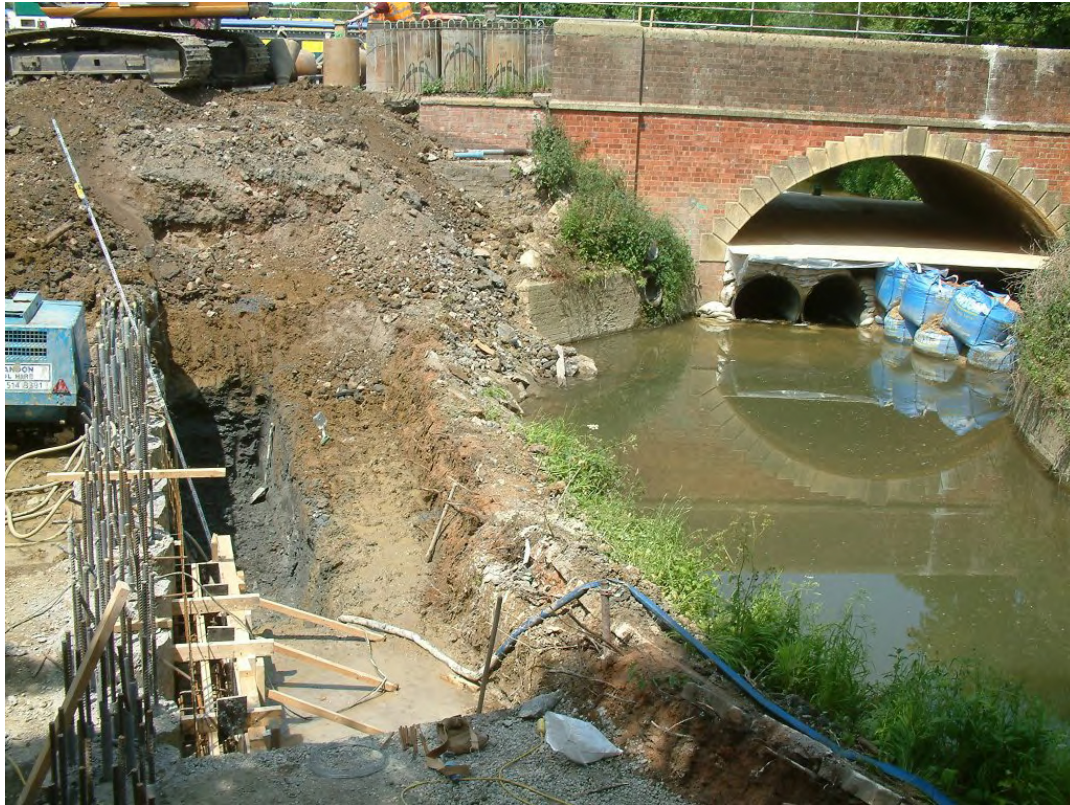
Plate 7: Trench 4 showing deep excavations and road bridge
