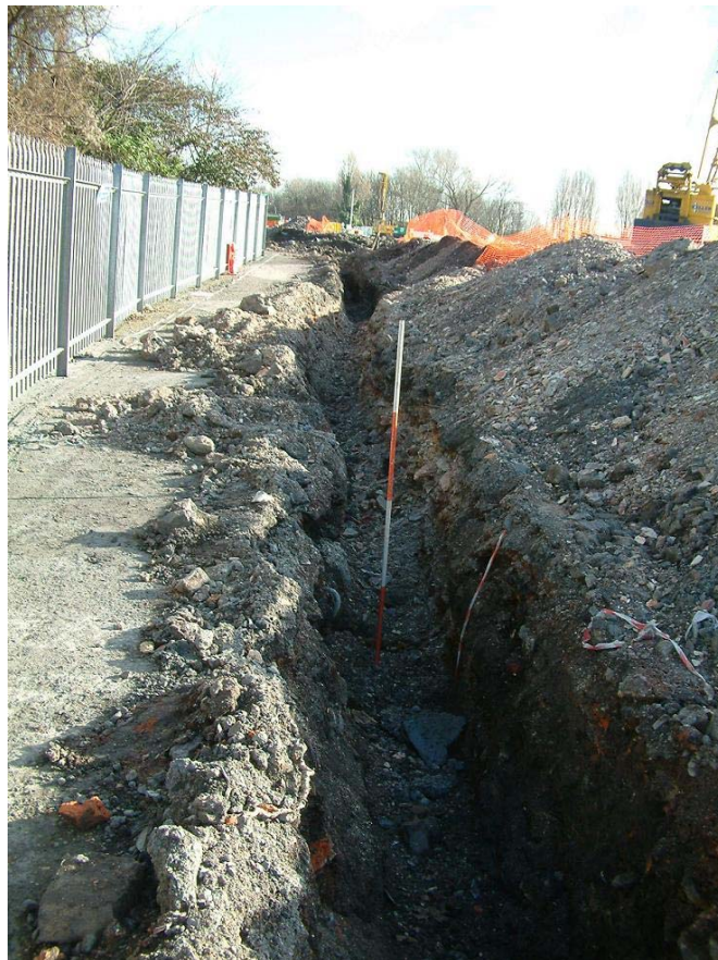
Plate 4. Trench 2 general view east, from west end
