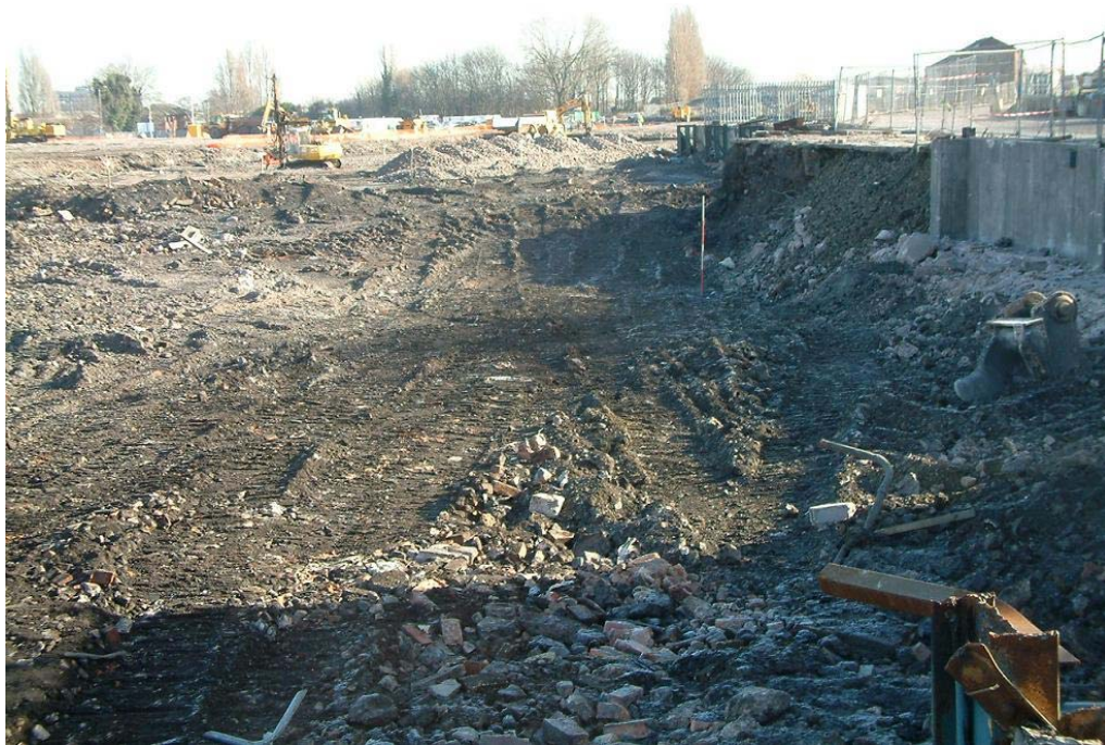
Plate 3. Area 1 south side, view east from south-west corner
