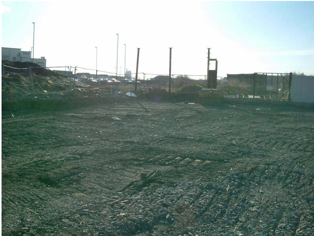
Plate 1. Area 1 view into south-east corner
