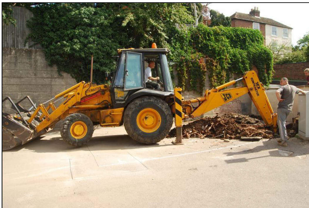
Plate 1 Trench 1 in progress, looking north
