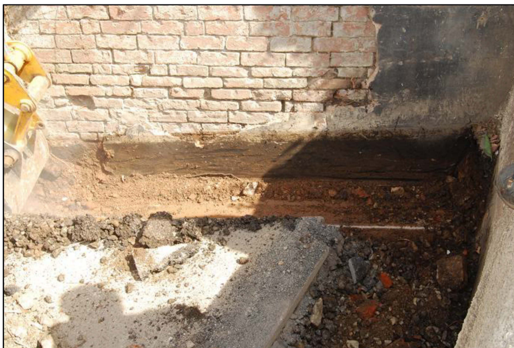
Plate 2 Trench 1 during excavation, showing the perimeter wall 101, looking north-east
