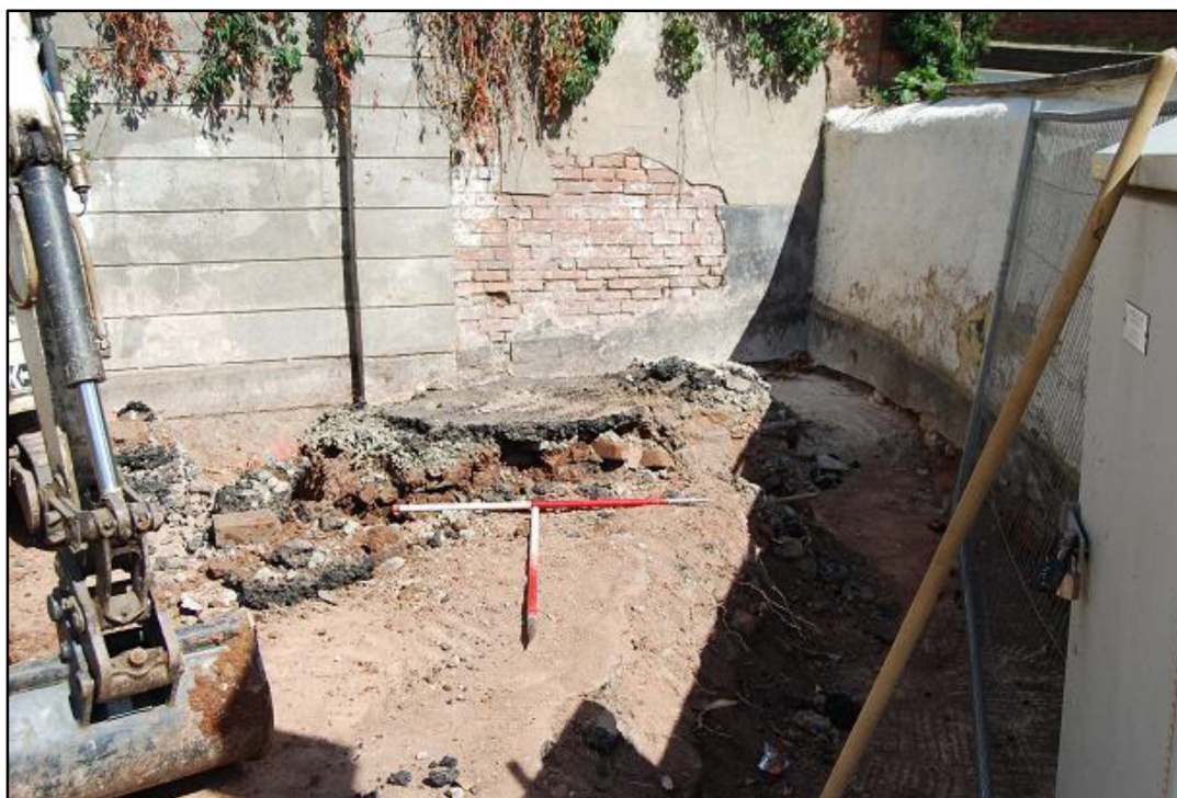
Plate 10 General view of Trench 2 after excavation, looking north-east
