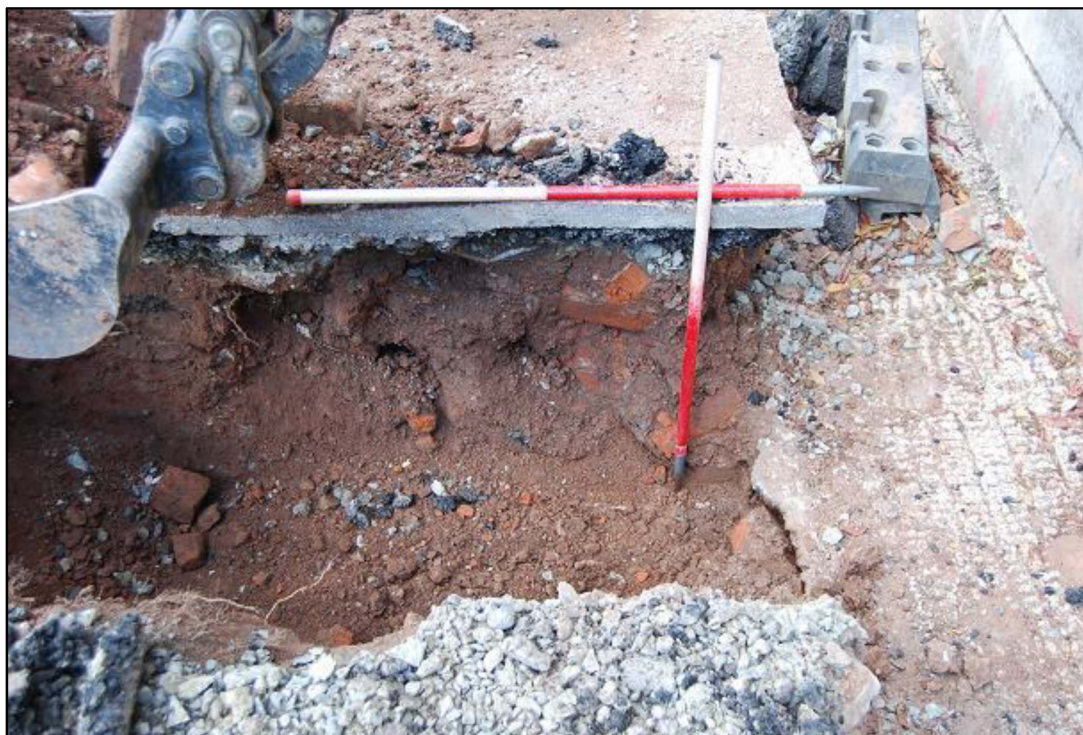
Plate 7 East facing section of Trench 2, showing modern surface, 201, backfilled material, 203, and natural marl, 204, at the base
