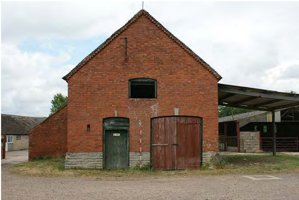
Plate 18: Different doors on brick extension south elevation
