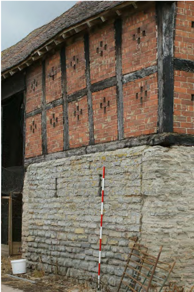
Plate 4: Northern most bay of barn from north east
