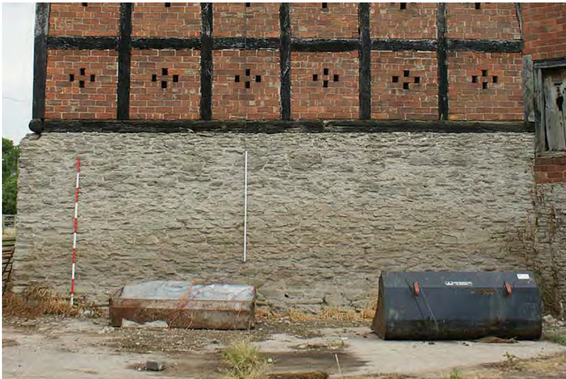
Plate 14: Phase 2 wall built to north of original barn
