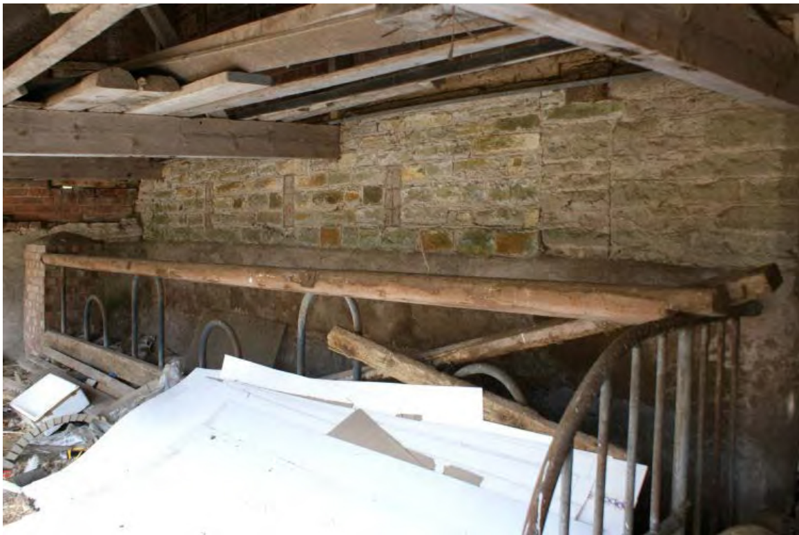
Plate 28: Concrete and aluminium feeding trough in lean-to shelter
