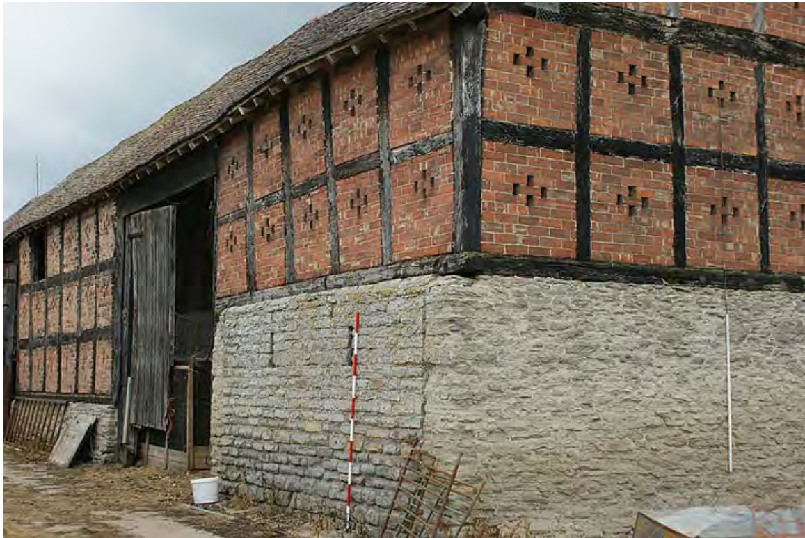
Plate 15: Phase three extension from the north east
