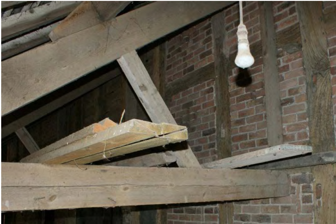
Plate 25: One of the lean-to half-trusses
