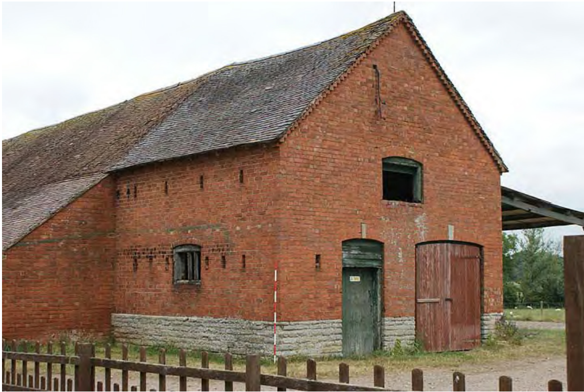
Plate 5: South extension of barn from south west
