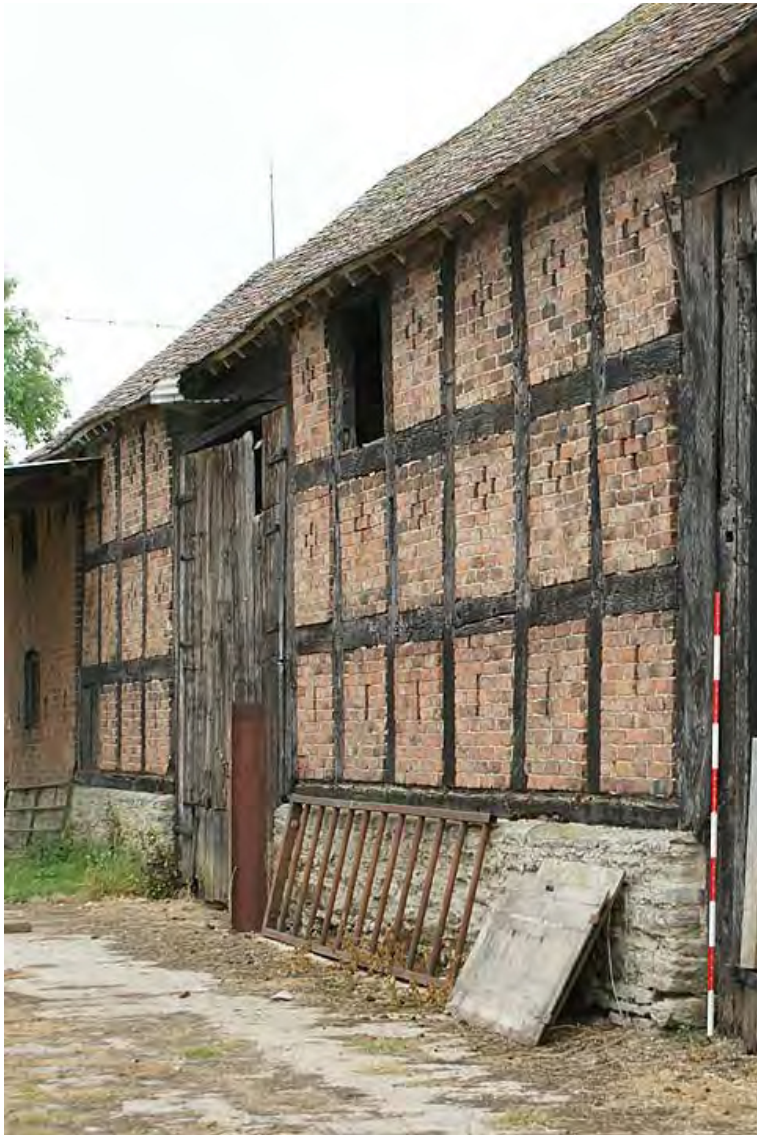
Plate 2: Central bays from the north east
