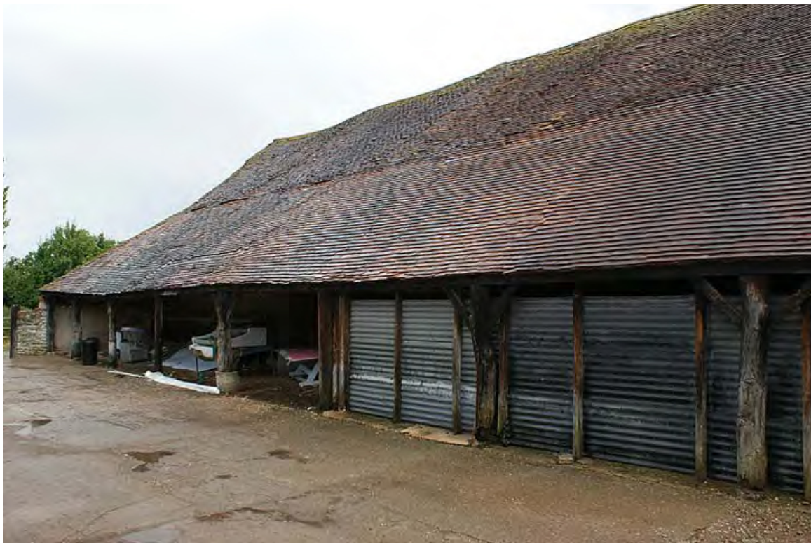
Plate 6: West elevation of barn, lean-to extension from south west
