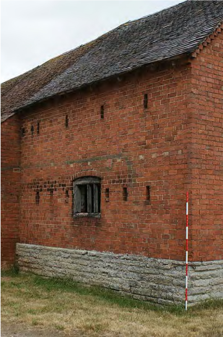
Plate 20: Ventilation holes on stable
