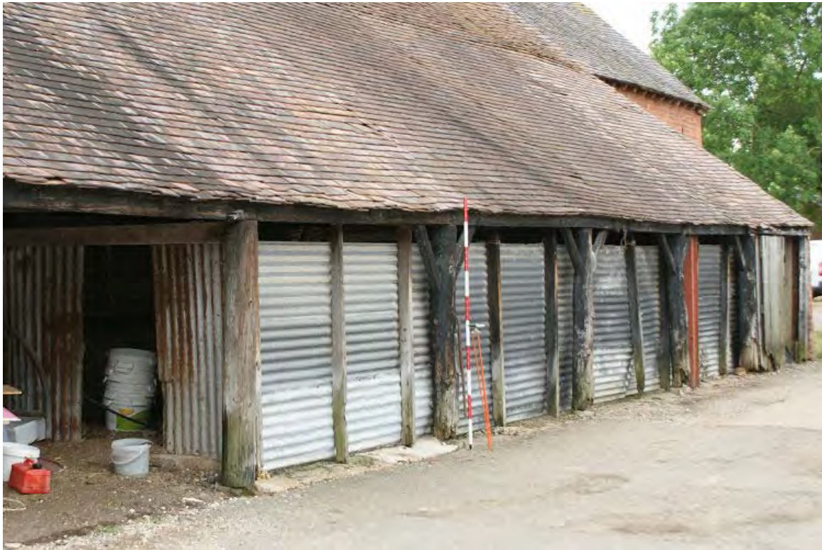
Plate 27: Corrugated infill to part of lean-to shelter
