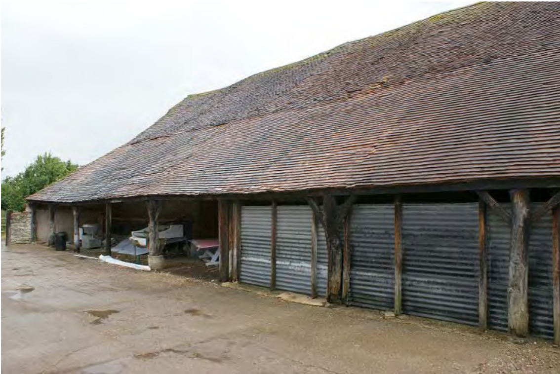
Plate 23: Lean-to against west elevation of barn
