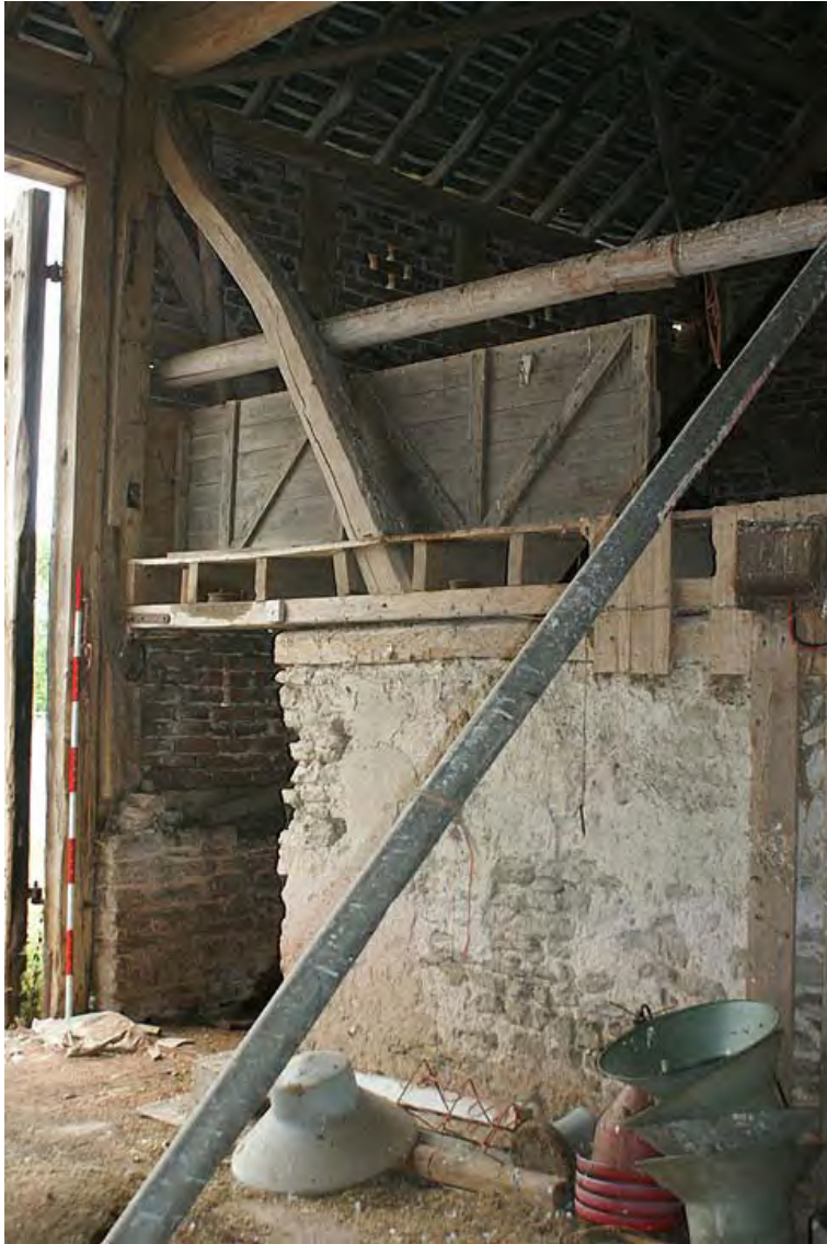
Plate 12: South lias stone wall built in phase 2 within phase 1 barn
