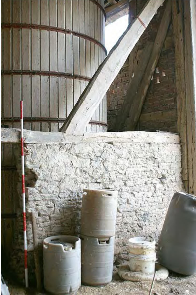
Plate 11: North lias stone wall built in phase 2 within phase 1 barn
