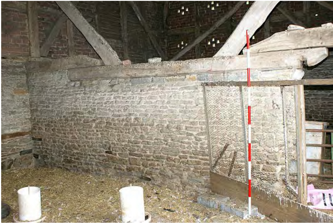
Plate 13: Phase 2 wall built to north of original barn
