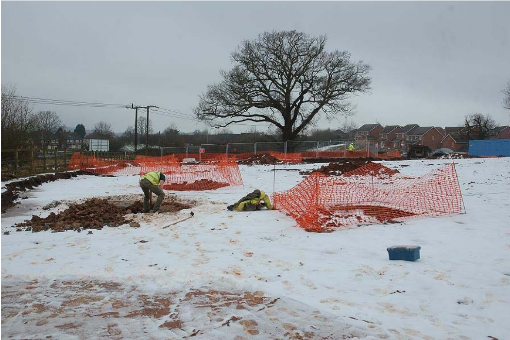
Plate 1: general site conditions facing west
