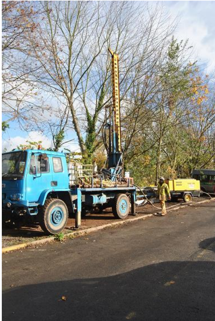
Plate 4 Sinking of Rotary Hole 2, looking north-west
