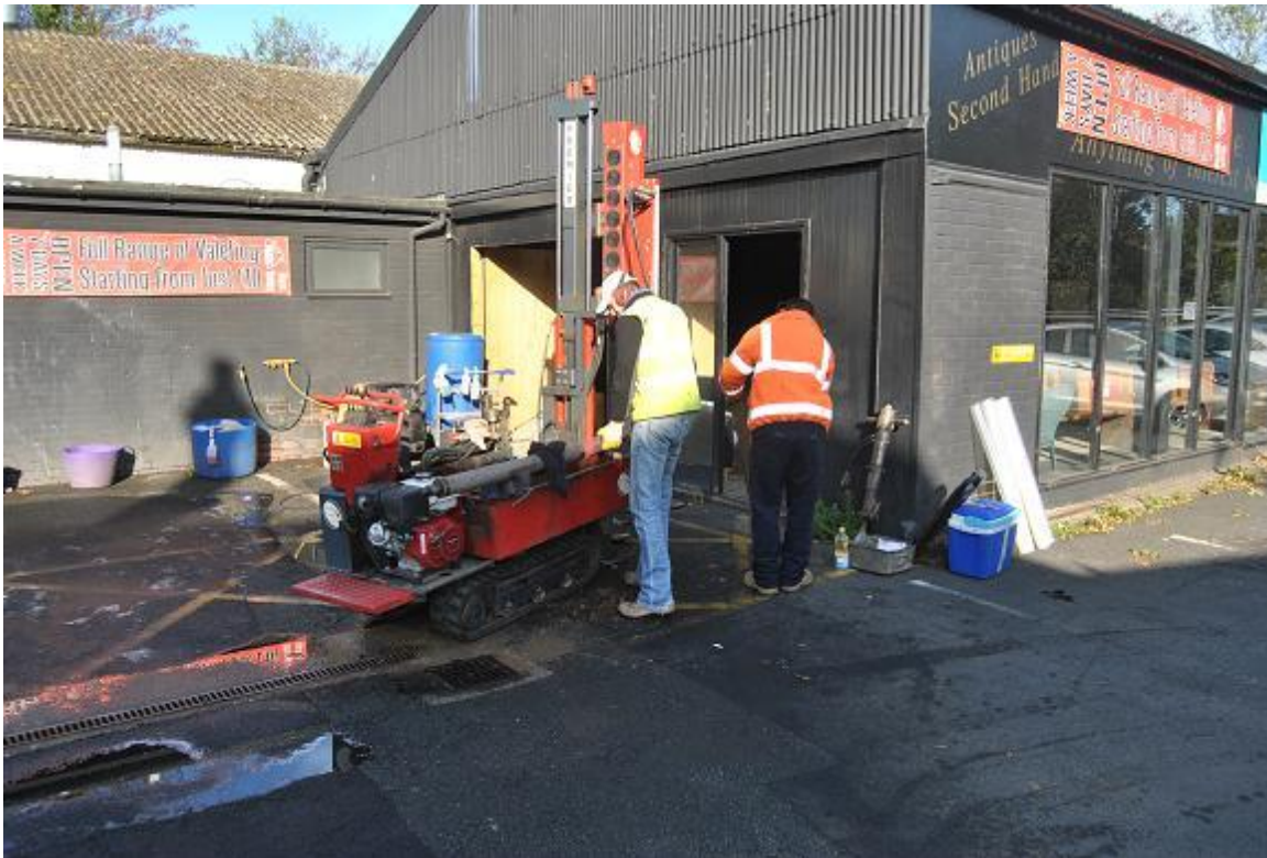
Plate 1 Sinking of Window Sample 4, looking north-west
