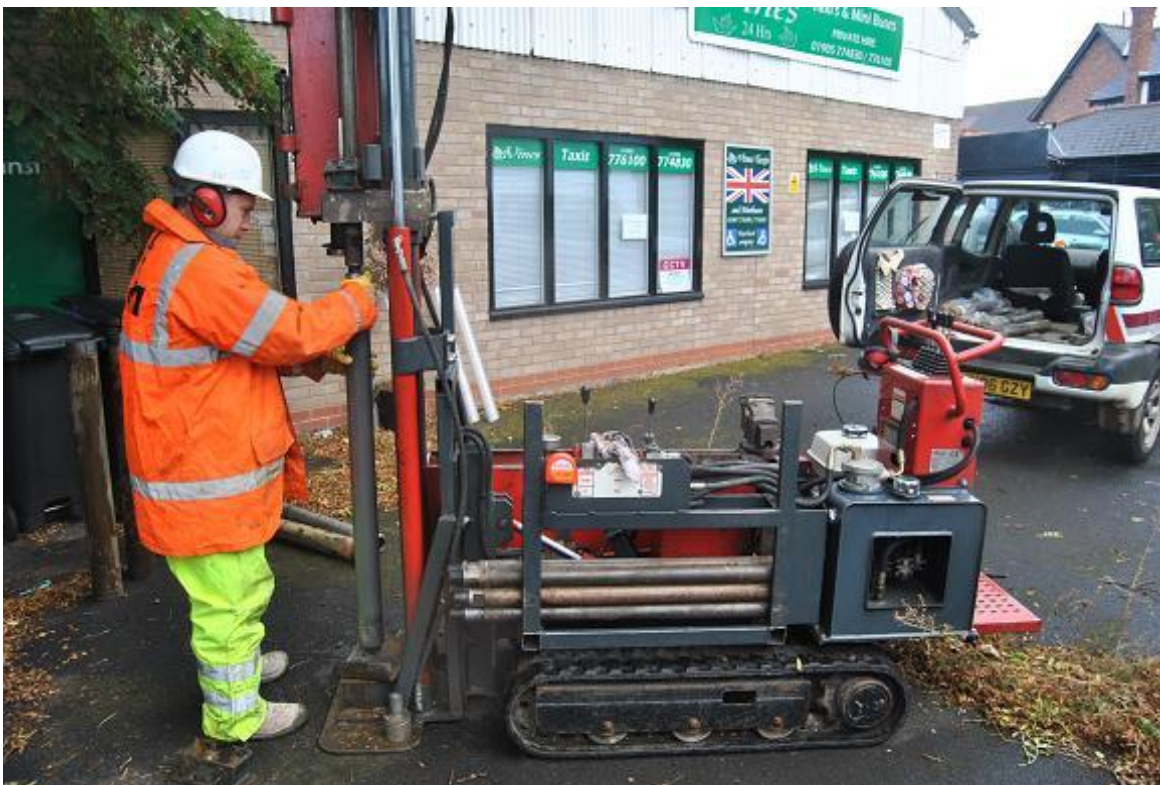
Plate 2 Sinking of Window Sample 6, looking north-east
