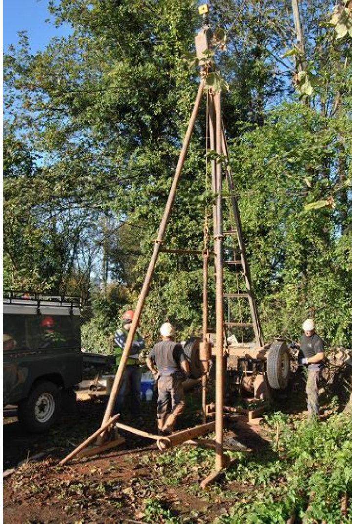
Plate 3 Sinking of Borehole 1, looking south-east
