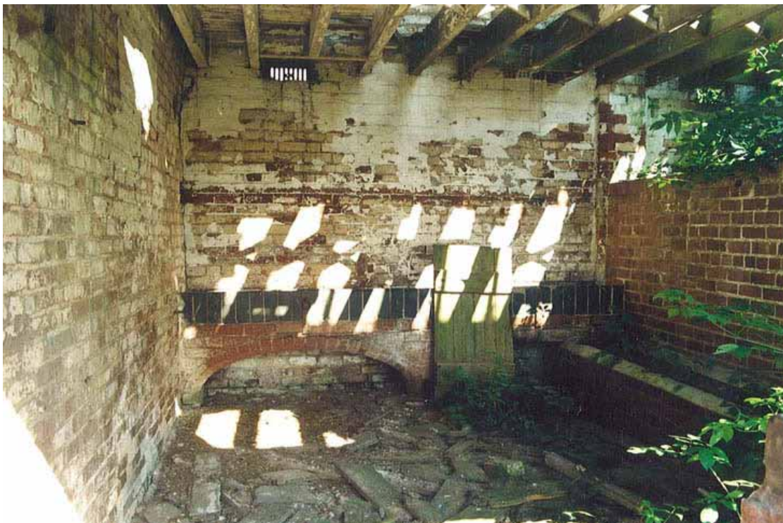
Plate 4. Phase 2, building 1; stable interior from the south west
