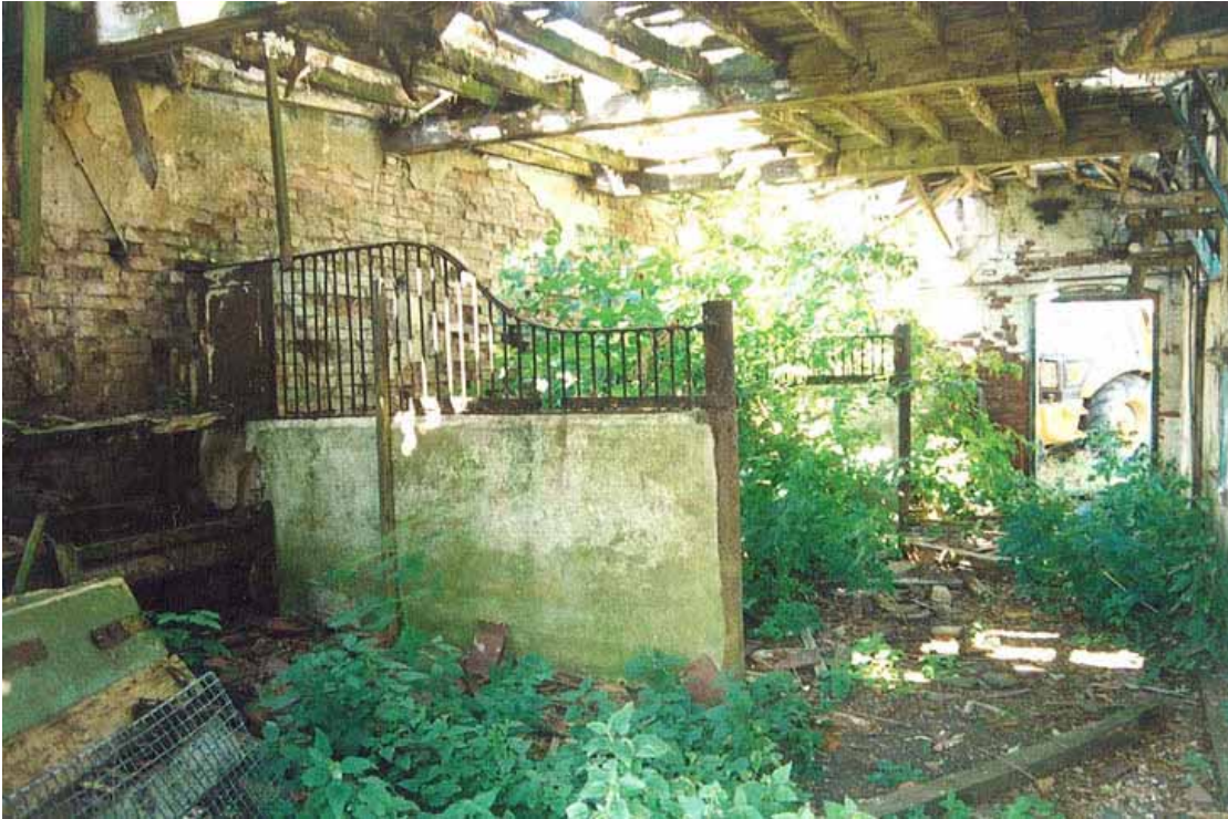
Plate 7. Phase 2, building 2; stable interior from the north-east
