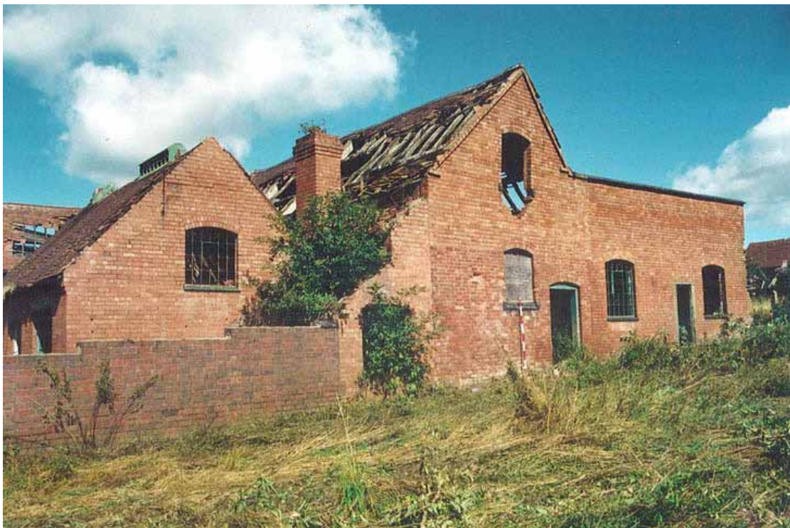
Plate 6. Phase 2, building 2 from the south
