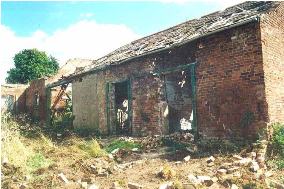
Plate 11. Phase 3, building 1; cart sheds from the west
