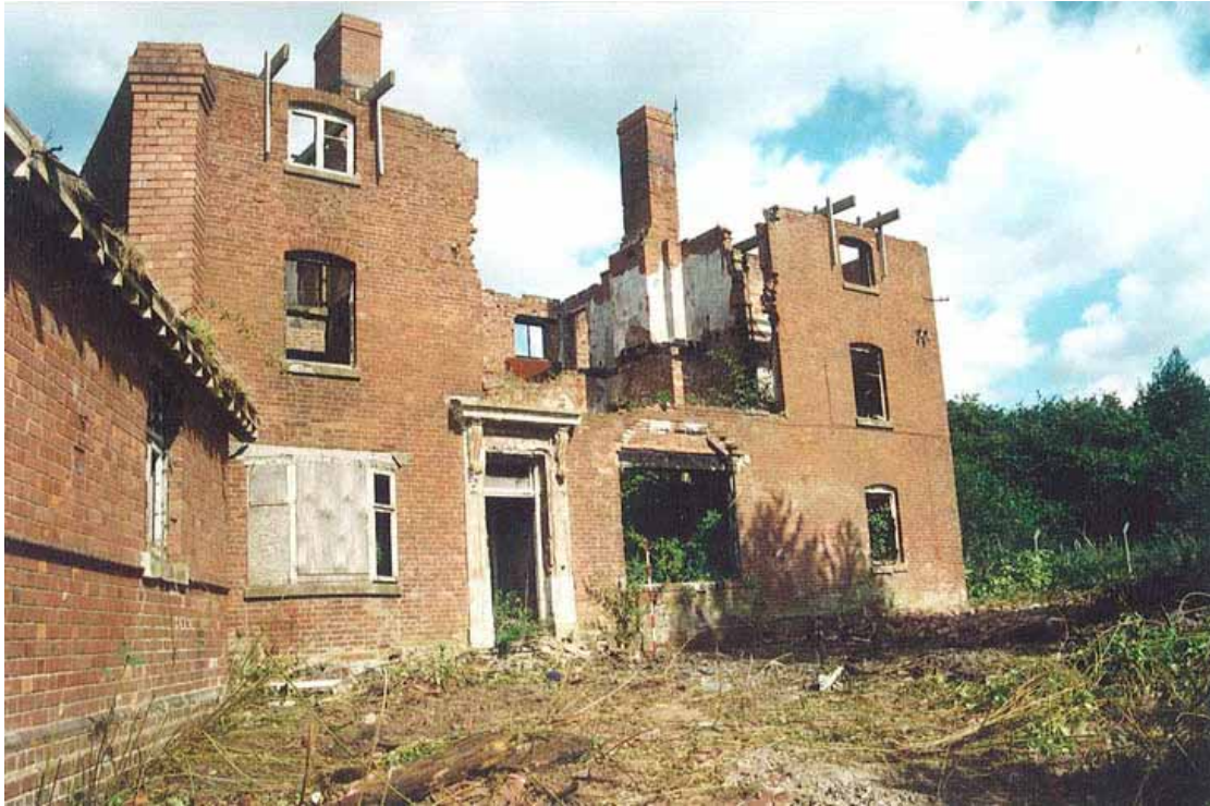
Plate 1. Phase 1, late 18 th century farmhouse from the south-west
