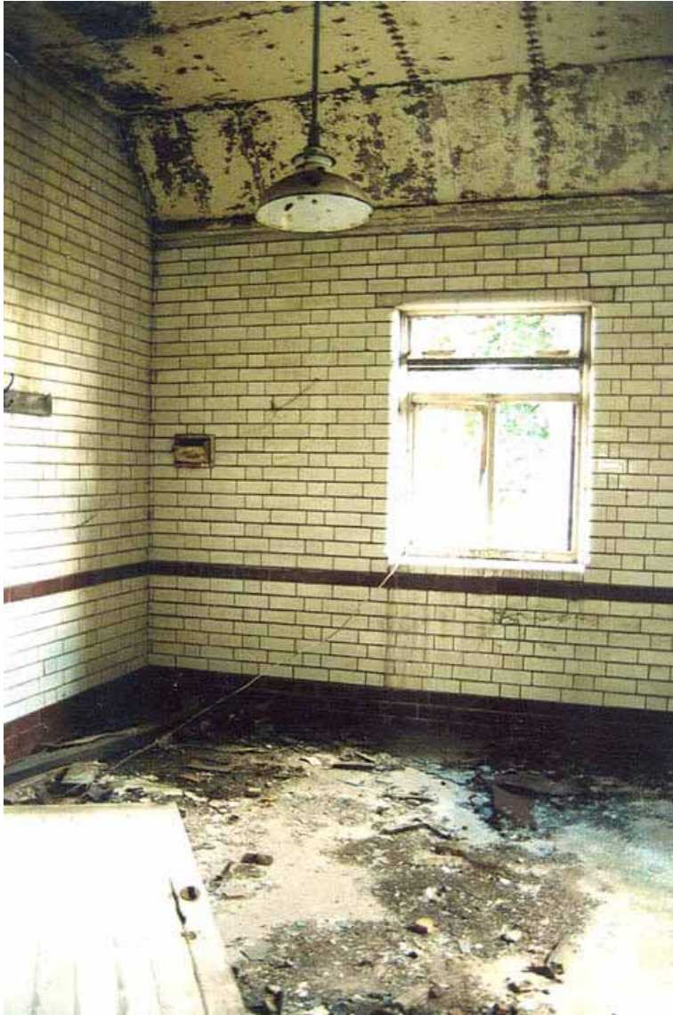
Plate 17. Phase 4, building 7; interior of the dairy, showing glazed bricks
