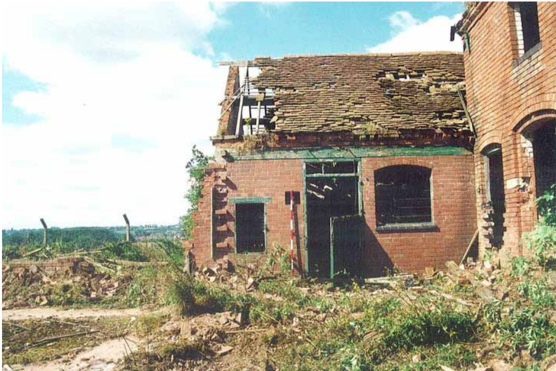
Plate 9. Phase 3, building 1; stable from the south-east
