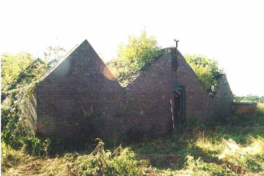
Plate 13. Phase 3, building 4; cow byre from the north
