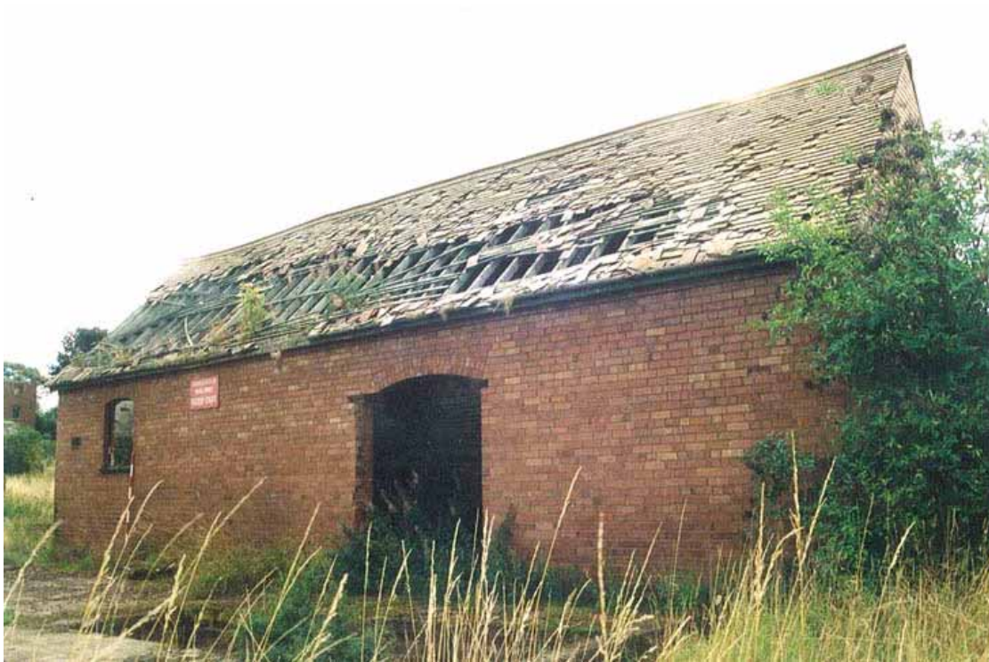
Plate 5. Phase 2, building 3 from the west
