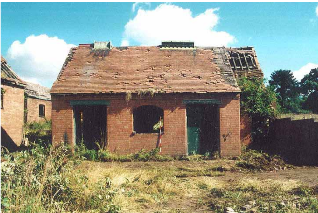
Plate 8. Phase 2, building 2; kiln from the south-west showing louvers on ridge line
