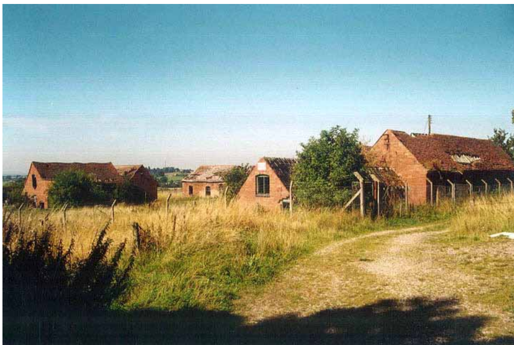
Barnsley Hall Farm buildings in 2001, from the north-east
