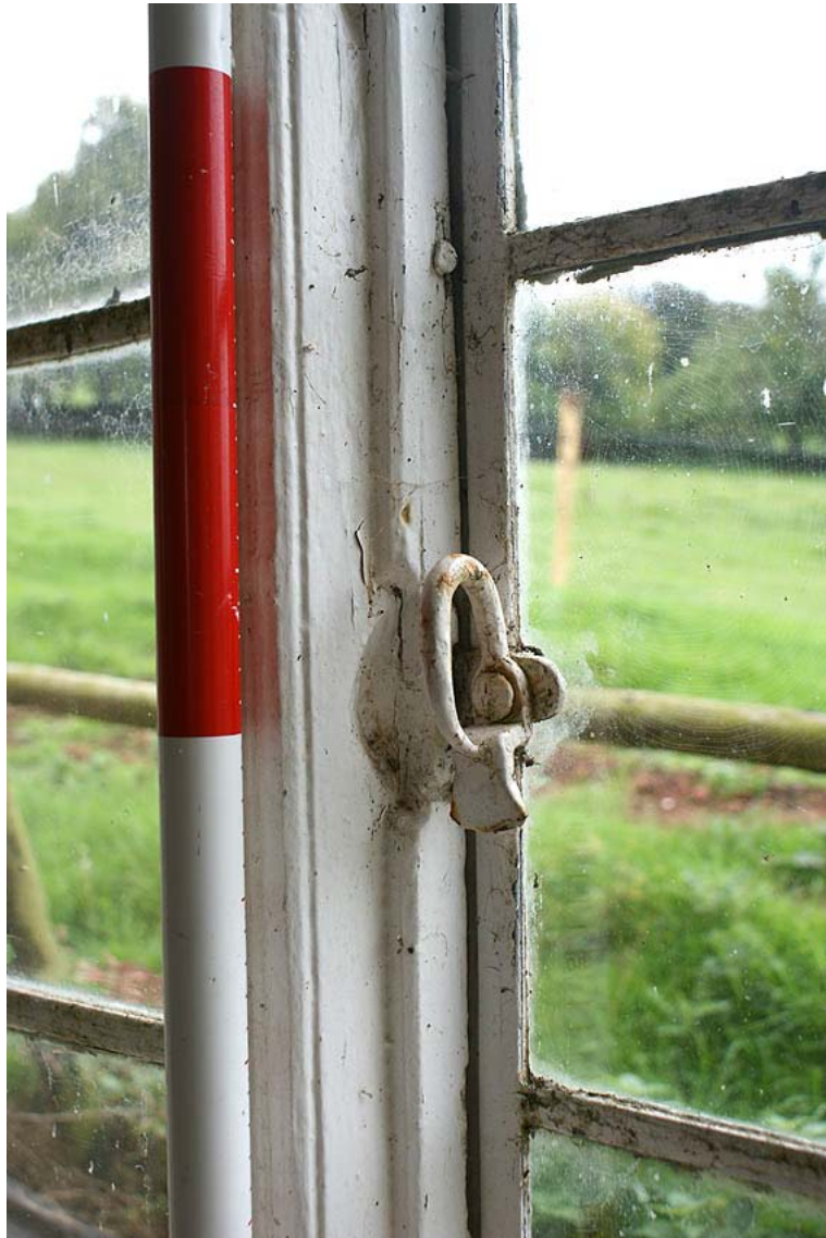
Plate 6: Turnbuckle catch
