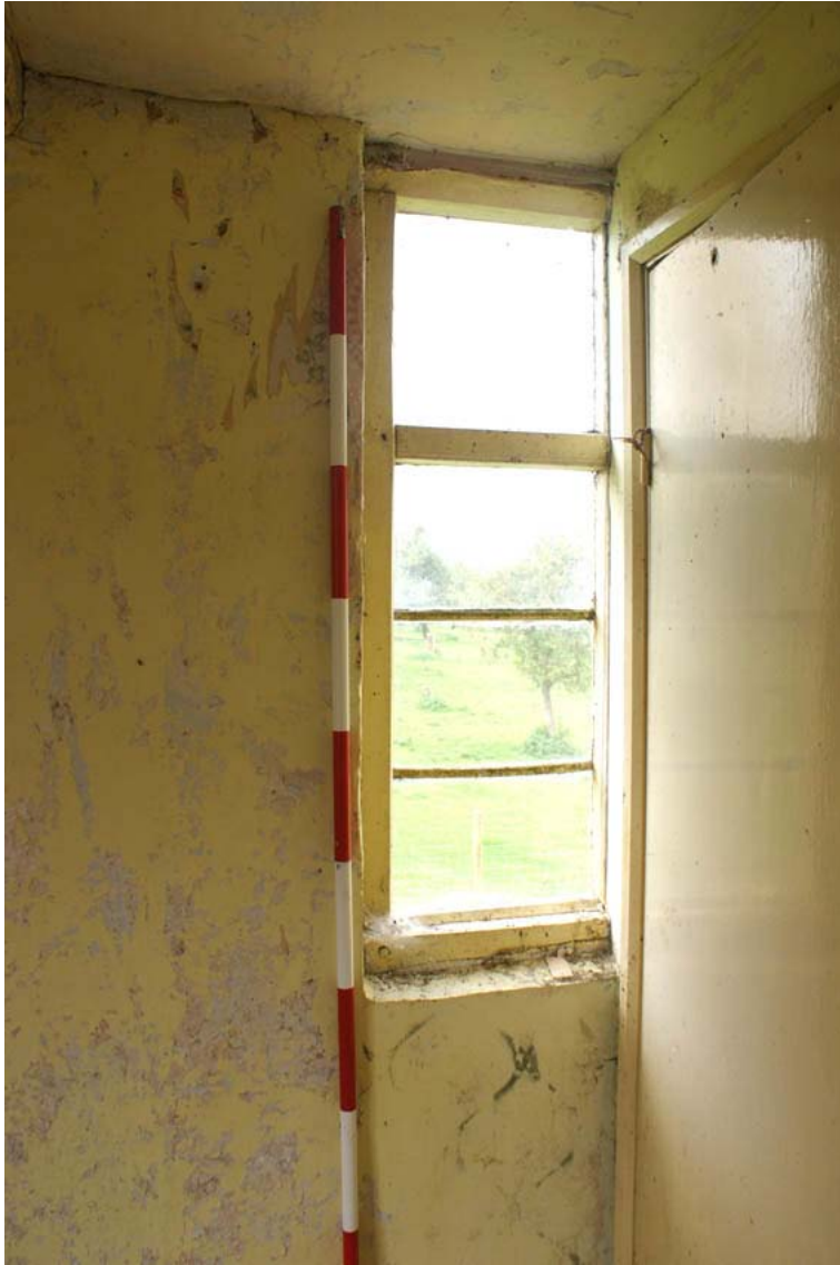
Plate 22: First floor window divided by partition
