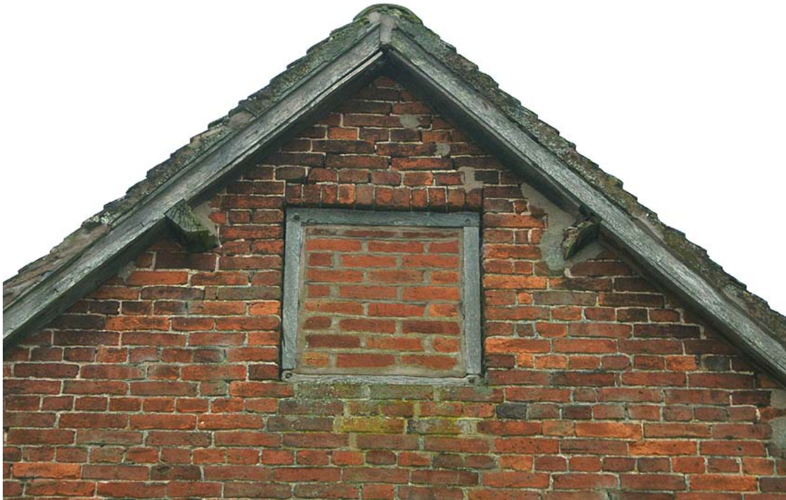
Plate 24: Blocked roof space window
