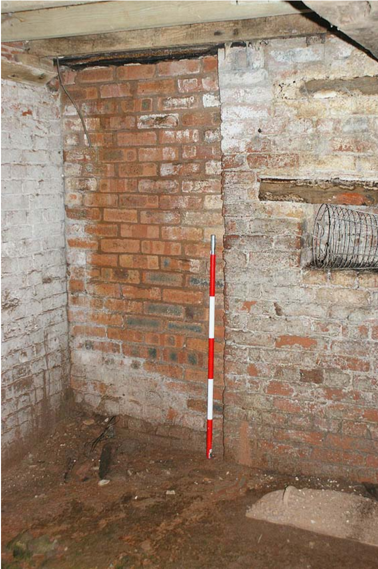
Plate 26: Blocked opening in cellar, former position of cellar access
