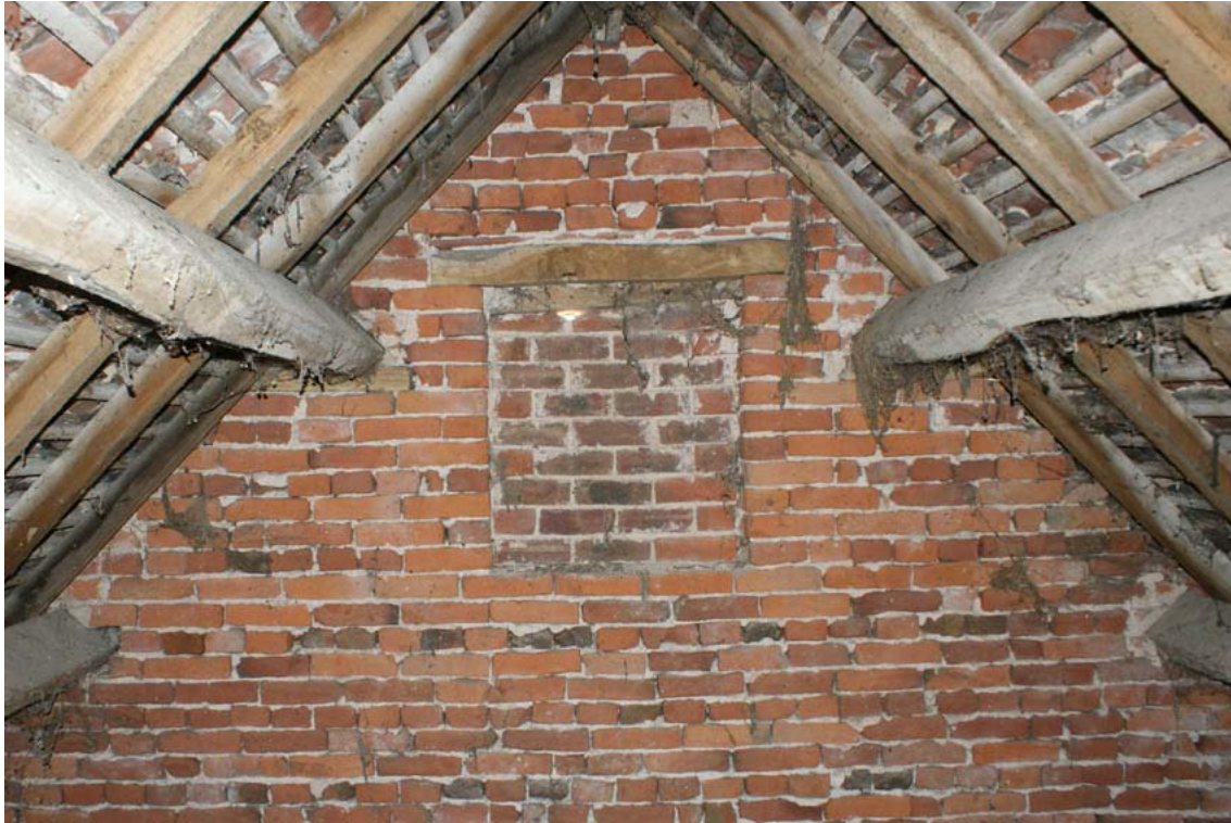
Plate 16: Blocked roof space window on south elevation
