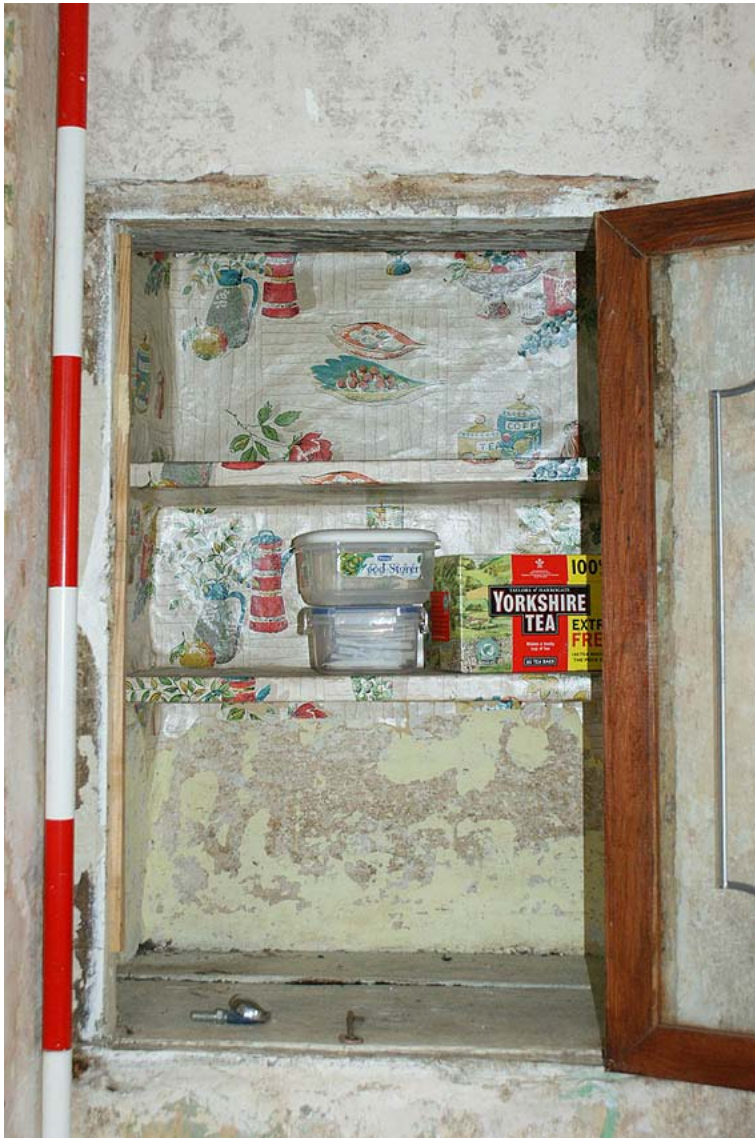
Plate 18: Small cupboard beside fireplace, possible bread oven
