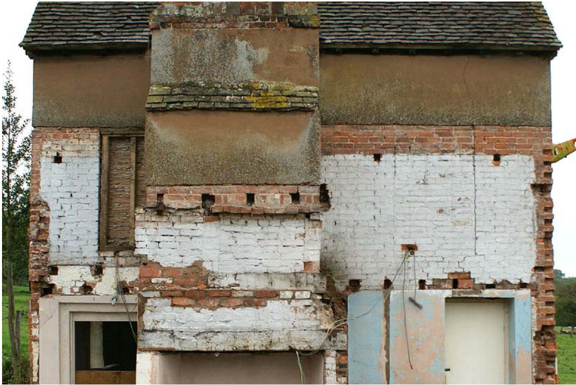
Plate 14: Blocked taking-in doors on first floor of cottage, east elevation
