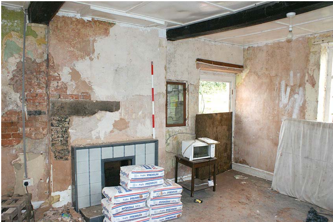
Plate 12: Ground floor interior showing chimney breast, from the north west
