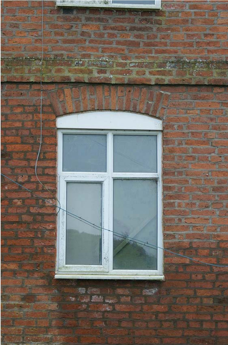
Plate 28: Modern glazing on north elevation of cottage
