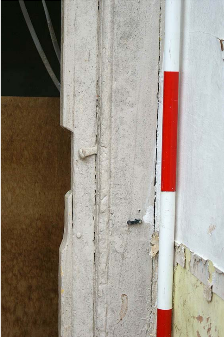
Plate 10: Bead moulding around original door
