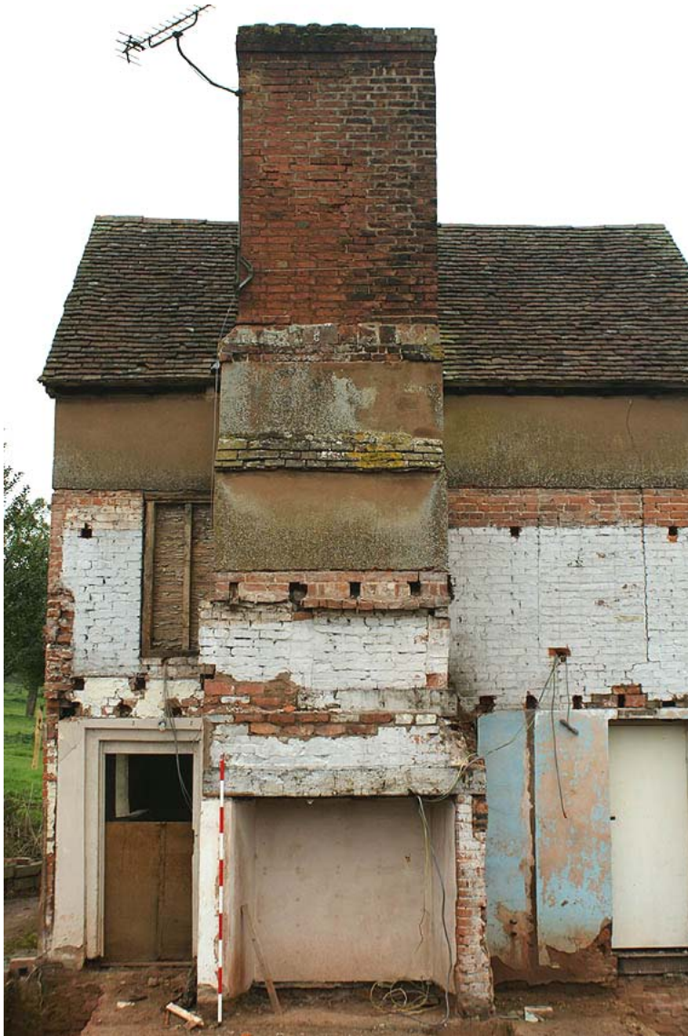
Plate 3: Chimney stack on east elevation
