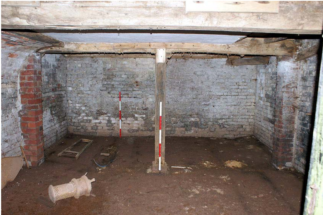
Plate 11: Cellar interior showing positions of drains in dips in floor
