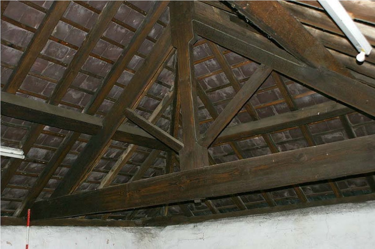
Plate 22: King post truss of the stable roof
