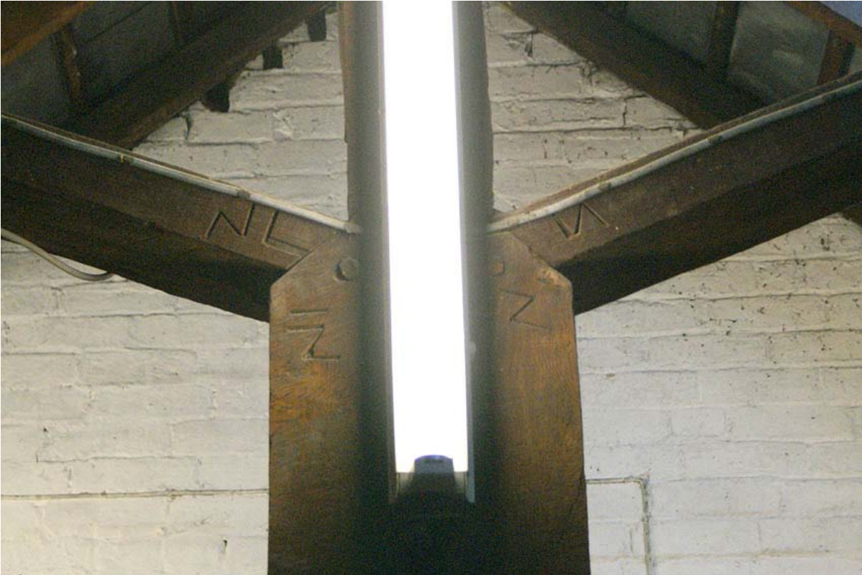
Plate 29: Example of carpenter's marks in the warehouse
