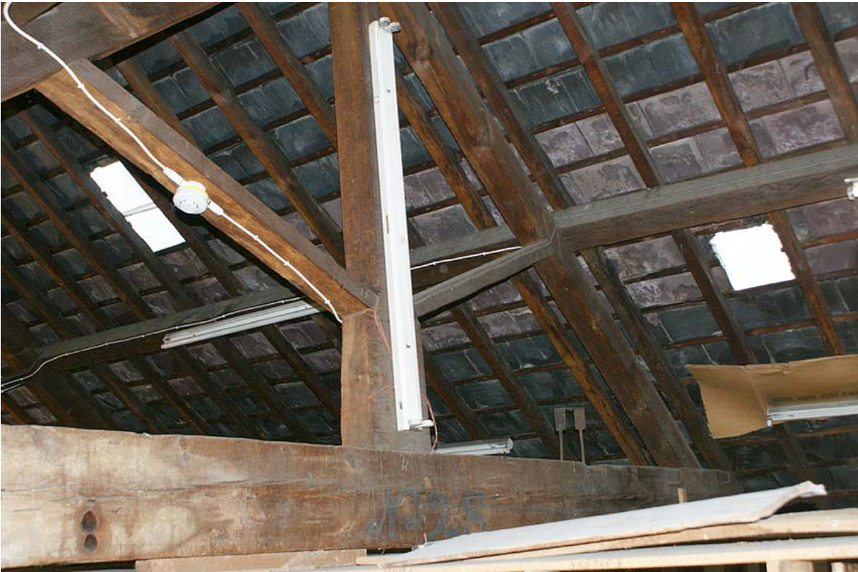
Plate 26: King post truss of the warehouse roof
