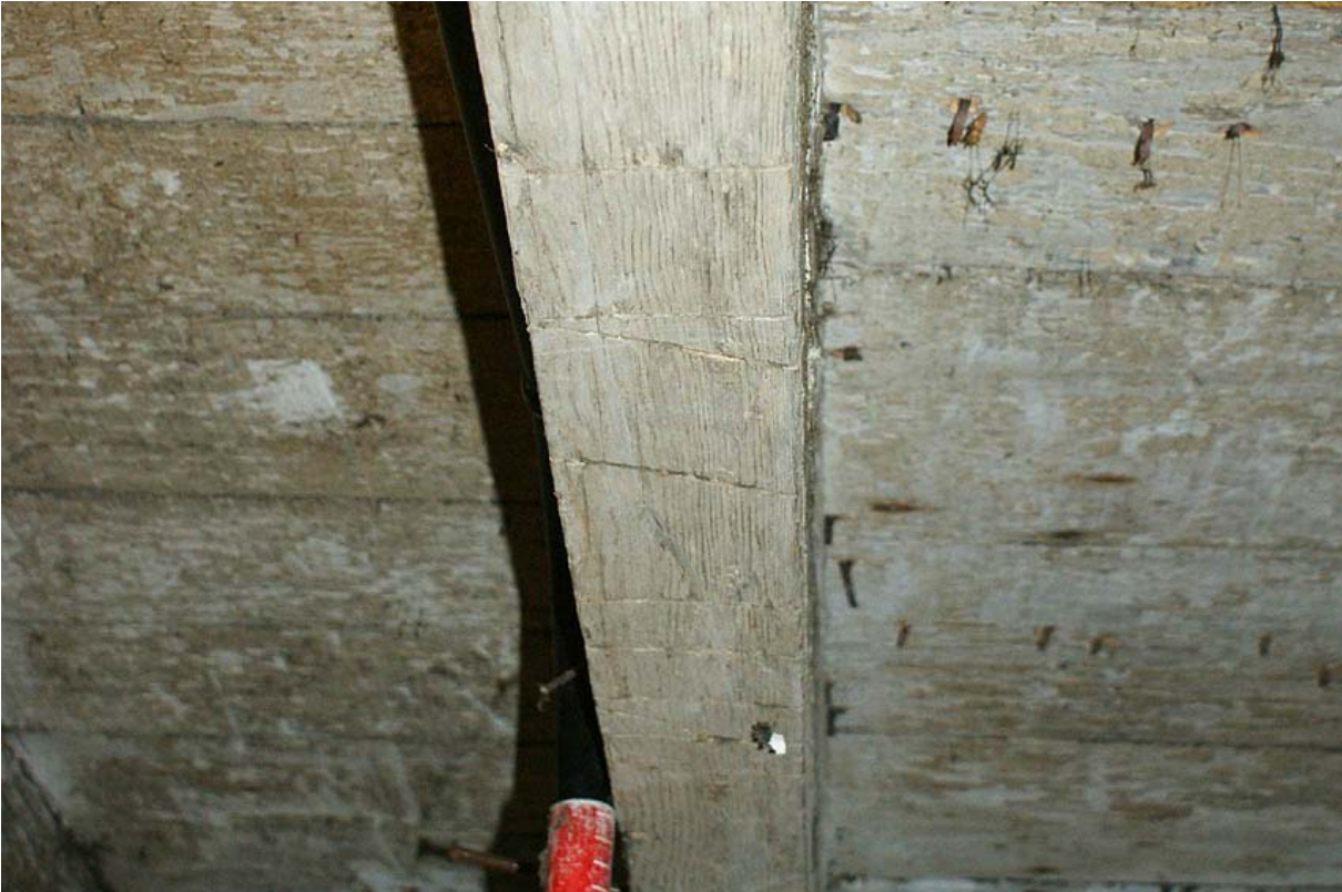
Plate 37: Baltic timber marks on cellar ceiling joist
