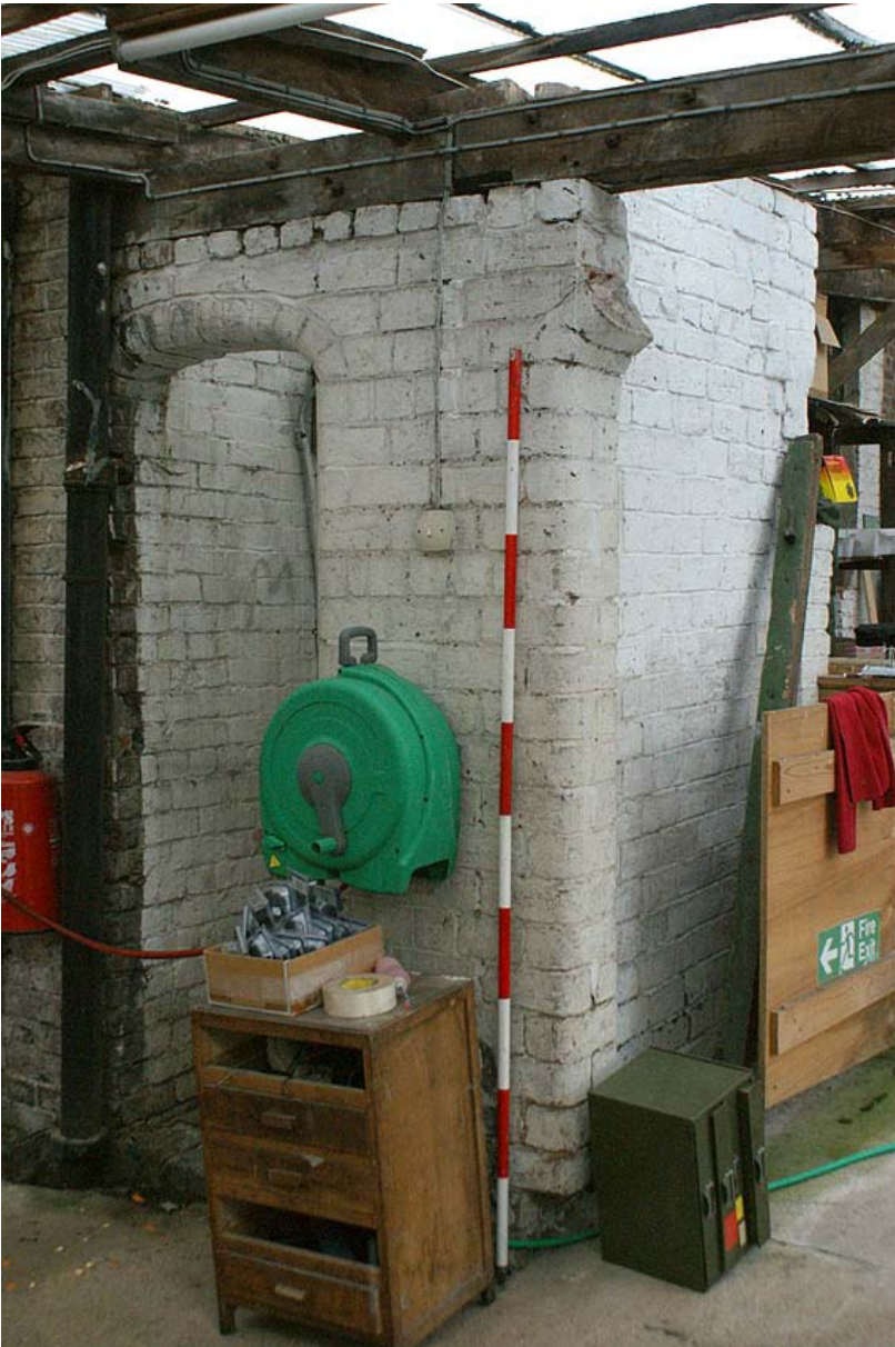
Plate 30: Arch springer adjacent to toilet extension from the south
