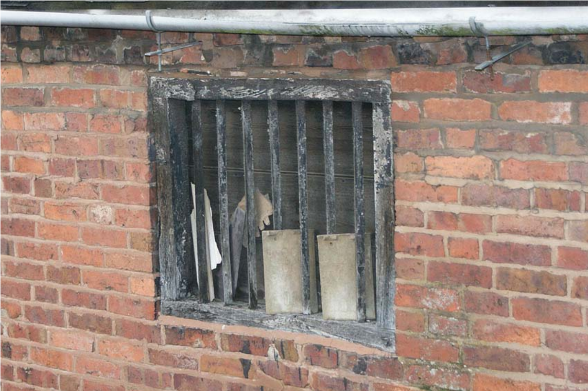
Plate 16: First floor window of the warehouse
