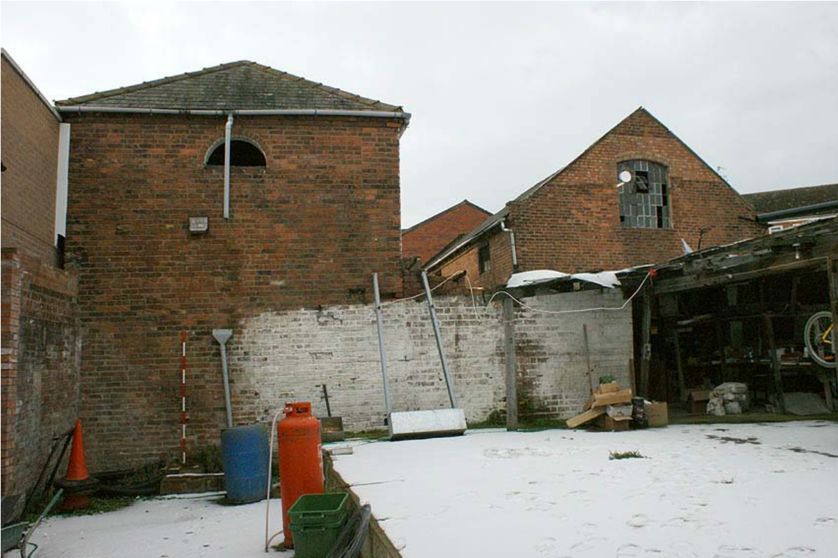
Plate 1: The buildings from the east
