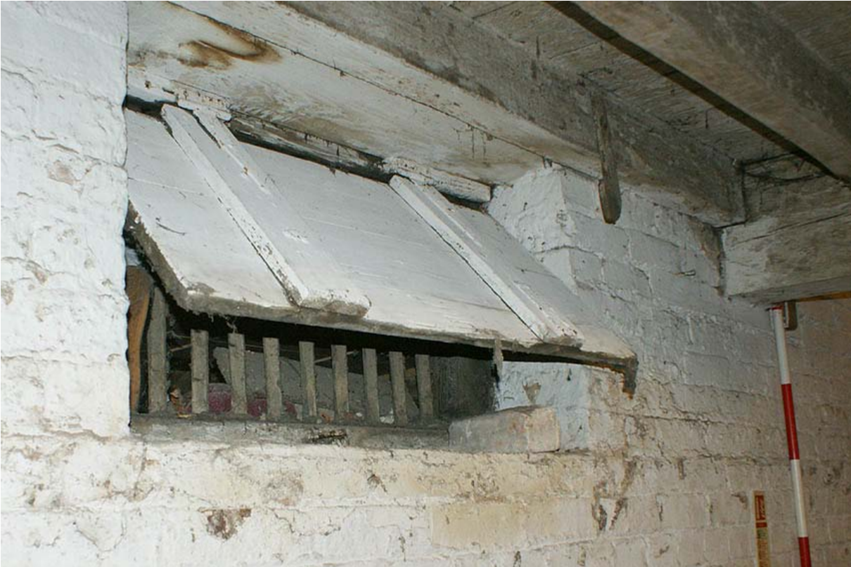
Plate 27: Warehouse cellar window from the interior showing shutter and bars
