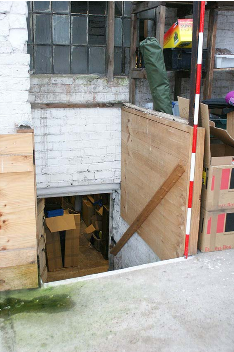
Plate 20: Exterior cellar stairs from the south east
