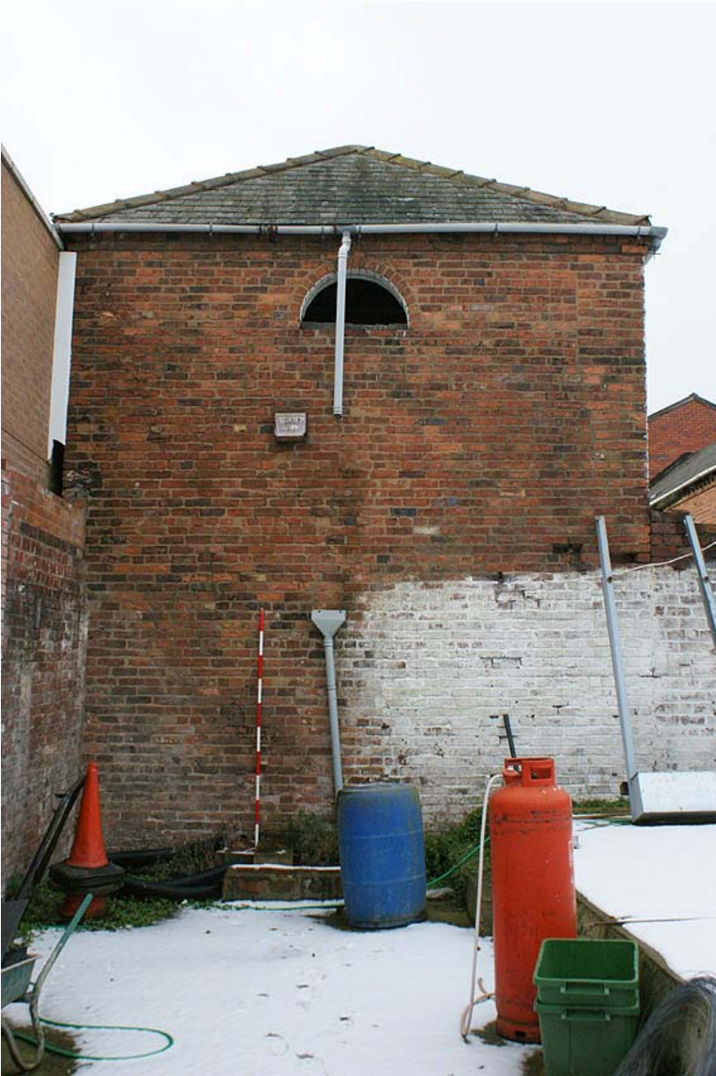
Plate 7: South east gable of the stable from the south east
