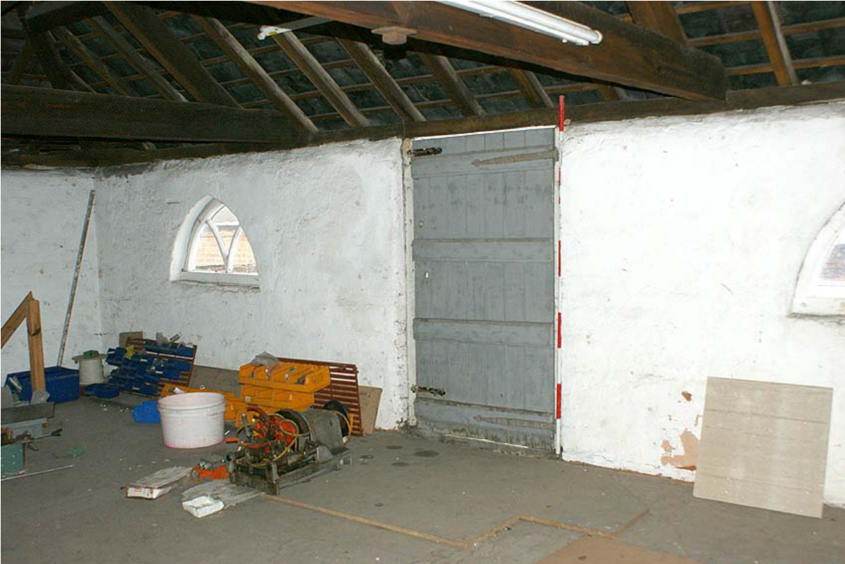
Plate 6: 1 st floor door and window of the stable
