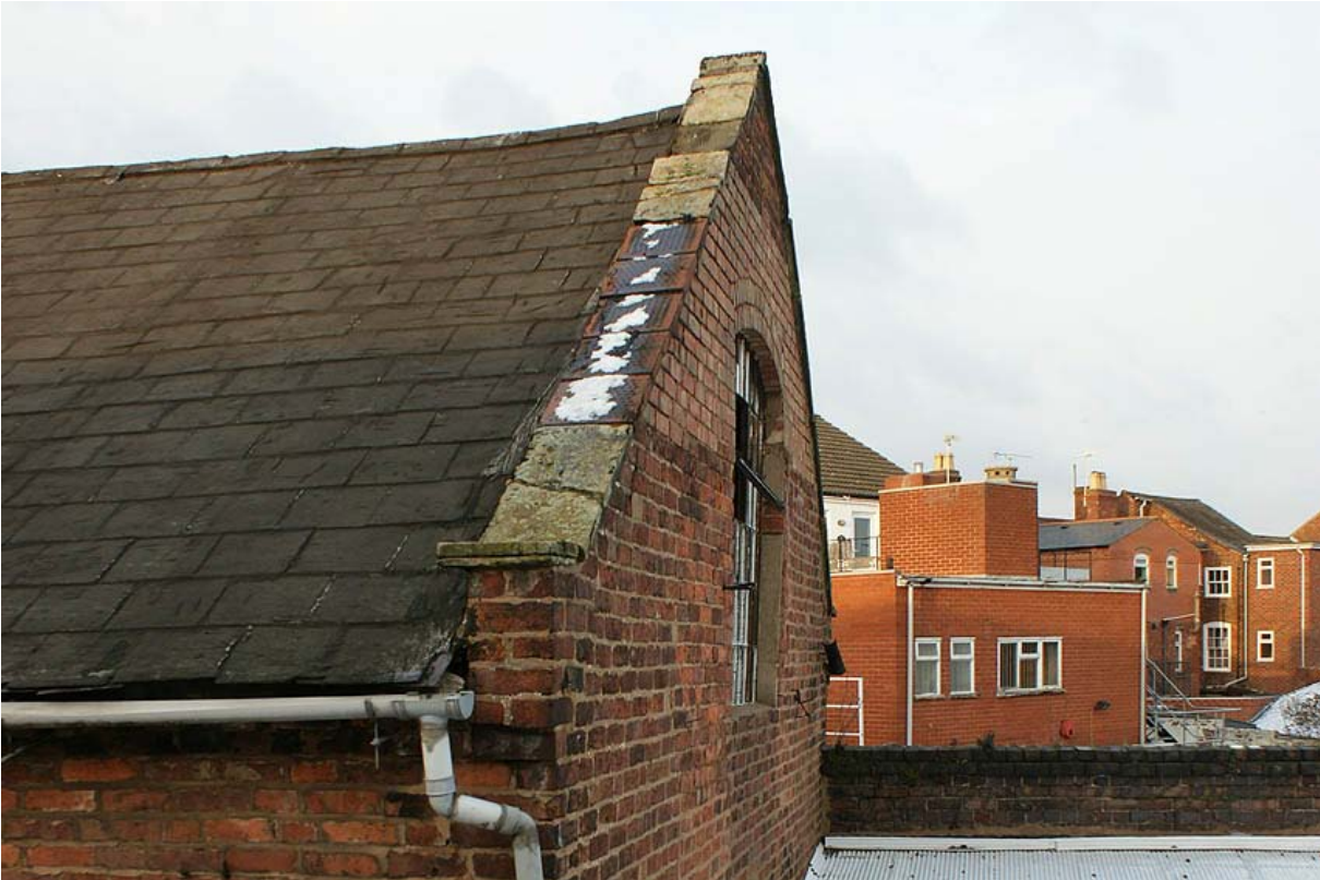
Plate 25: Warehouse south east gable from the south showing the parapet
