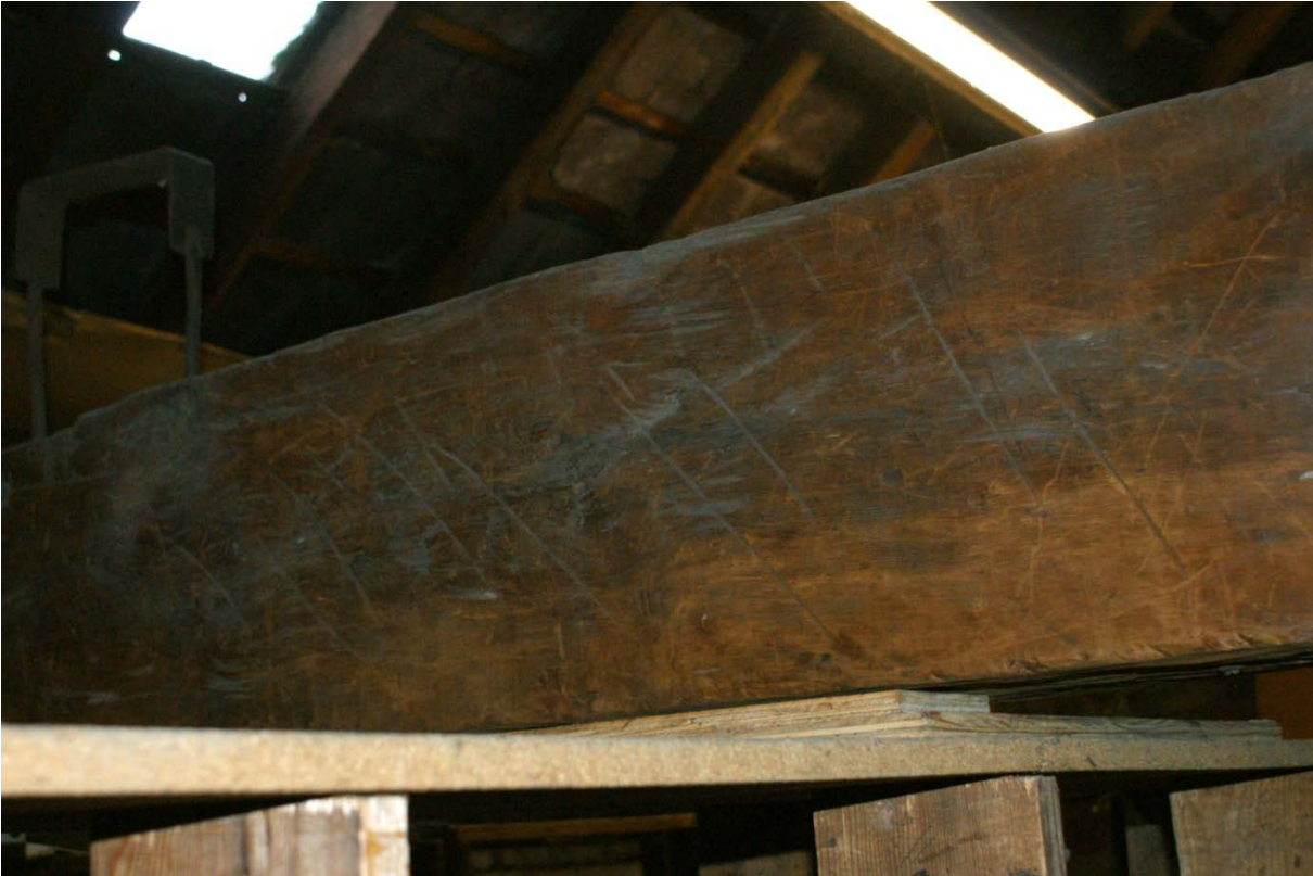
Plate 36: Baltic timber marks on tie beam in warehouse
