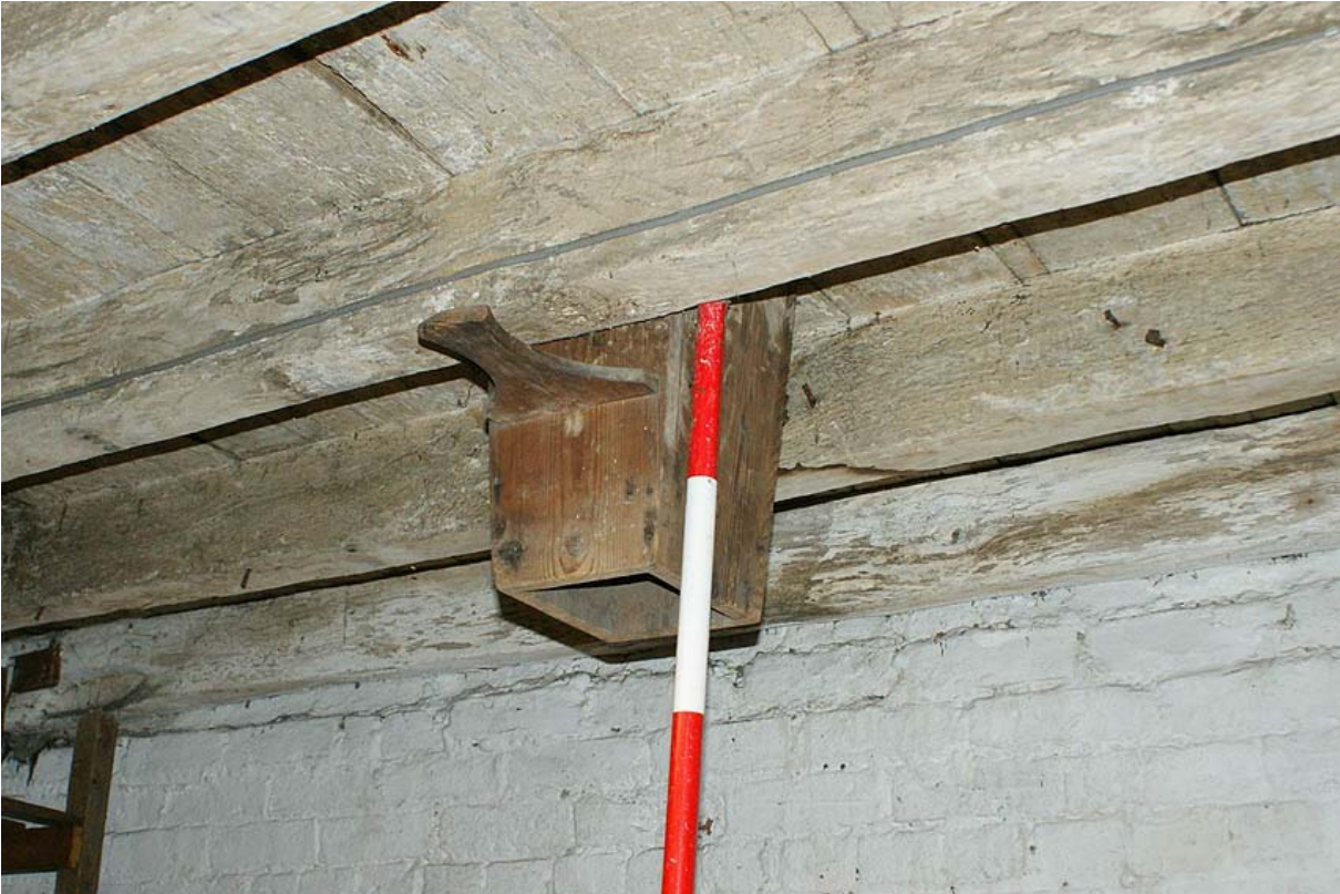
Plate 34: One of the grain chutes in the warehouse cellar ceiling
