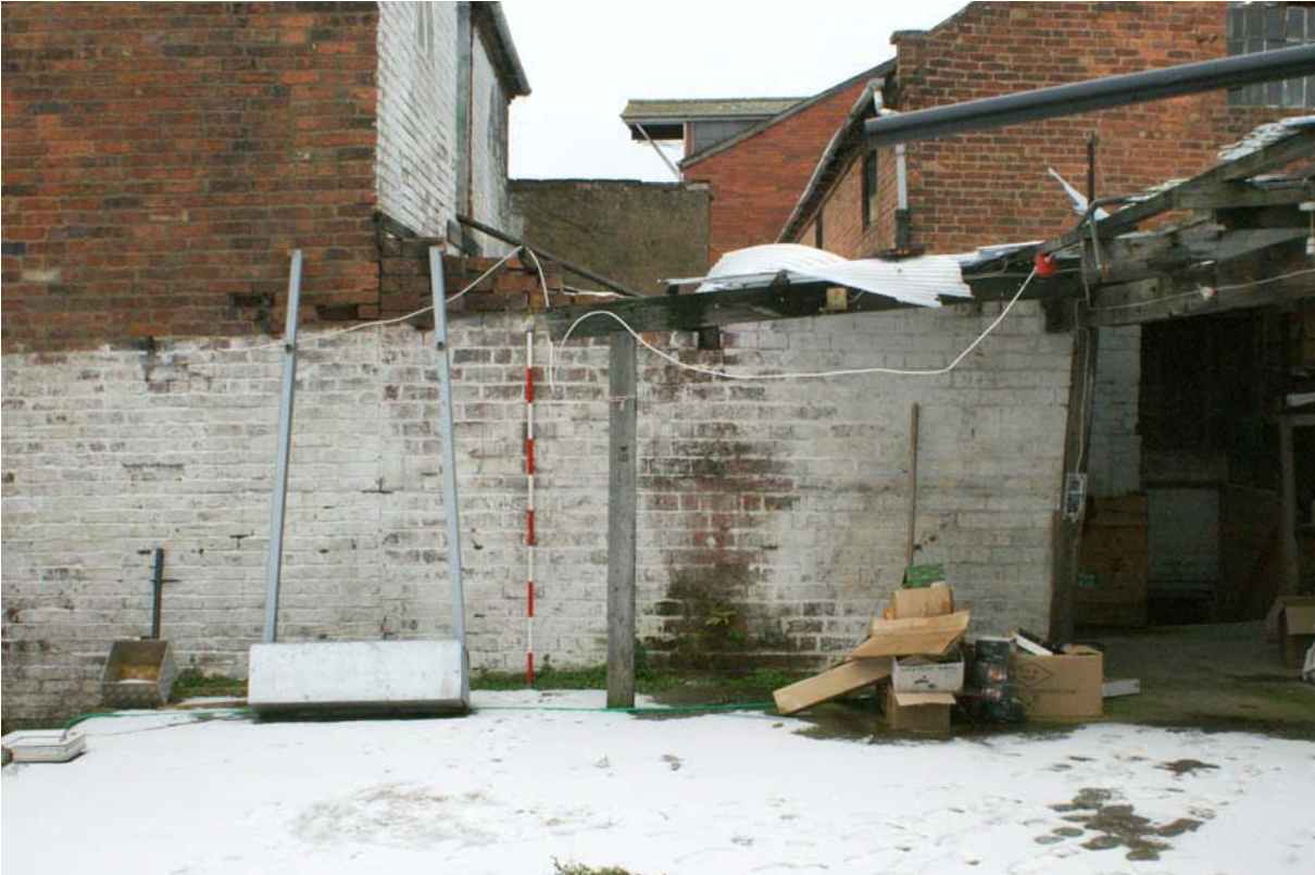
Plate 33: Return of wall to join onto gable of stable
