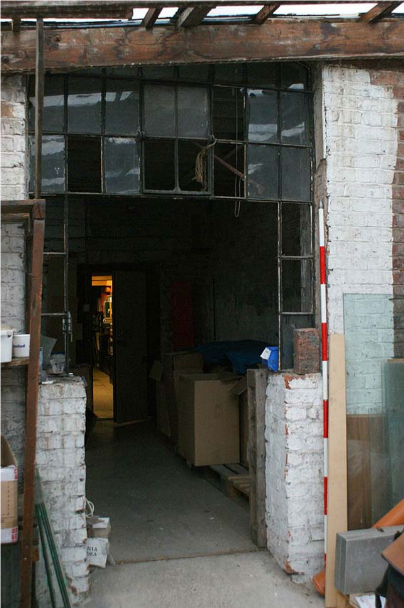
Plate 13: Warehouse iron frame window converted to a door
