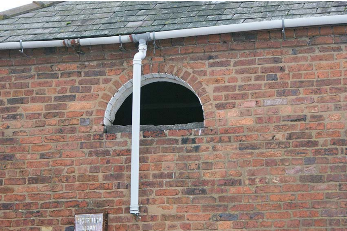
Plate 8: Semi-circular window in south east gable of stable
