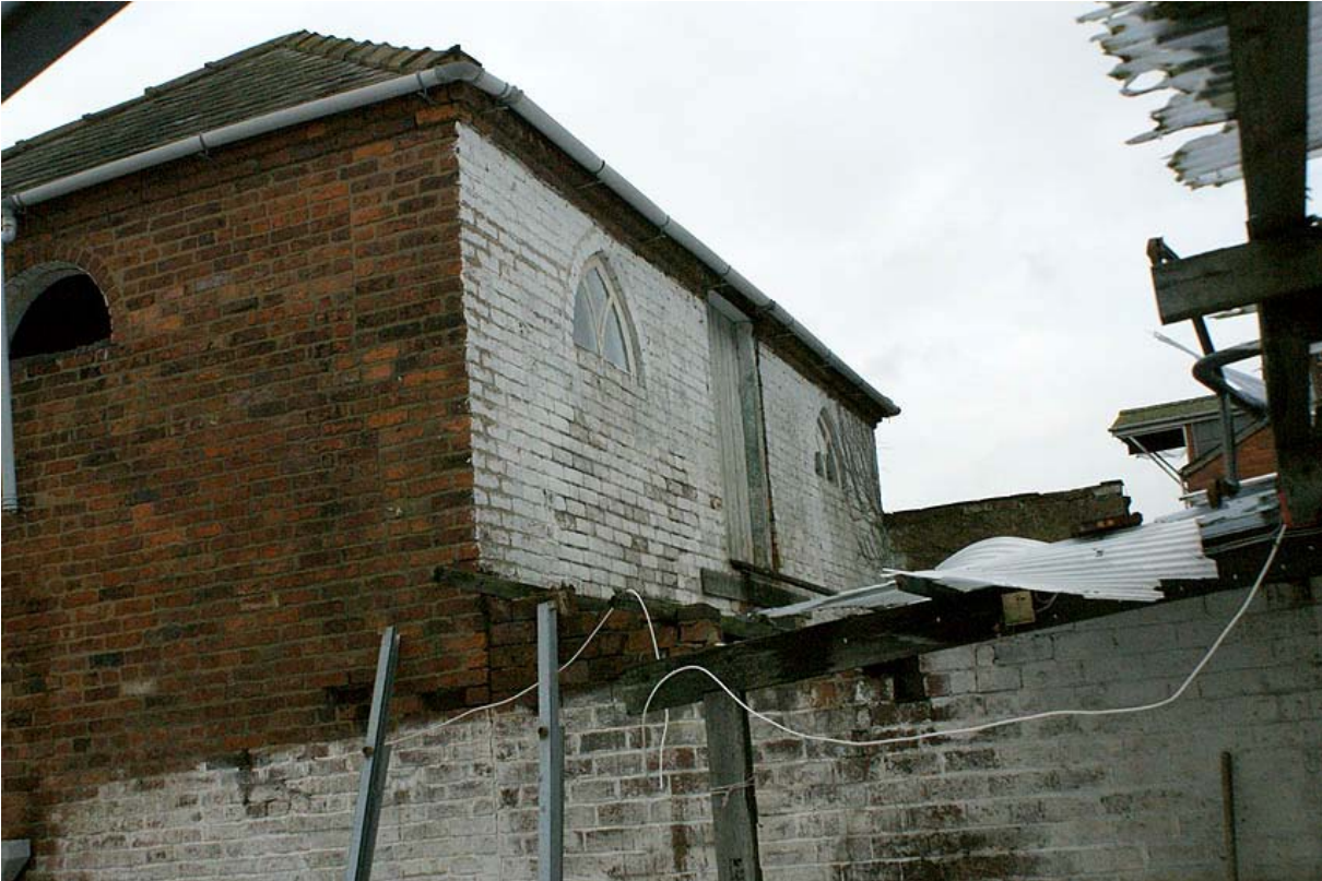
Plate 2: The stable from the north east
