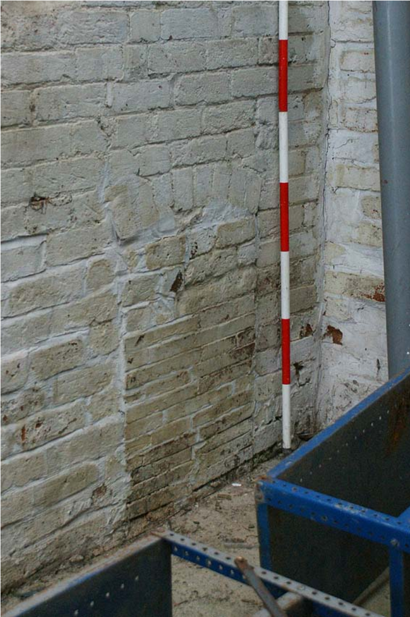
Plate 23: Small opening in north east elevation of the stable
