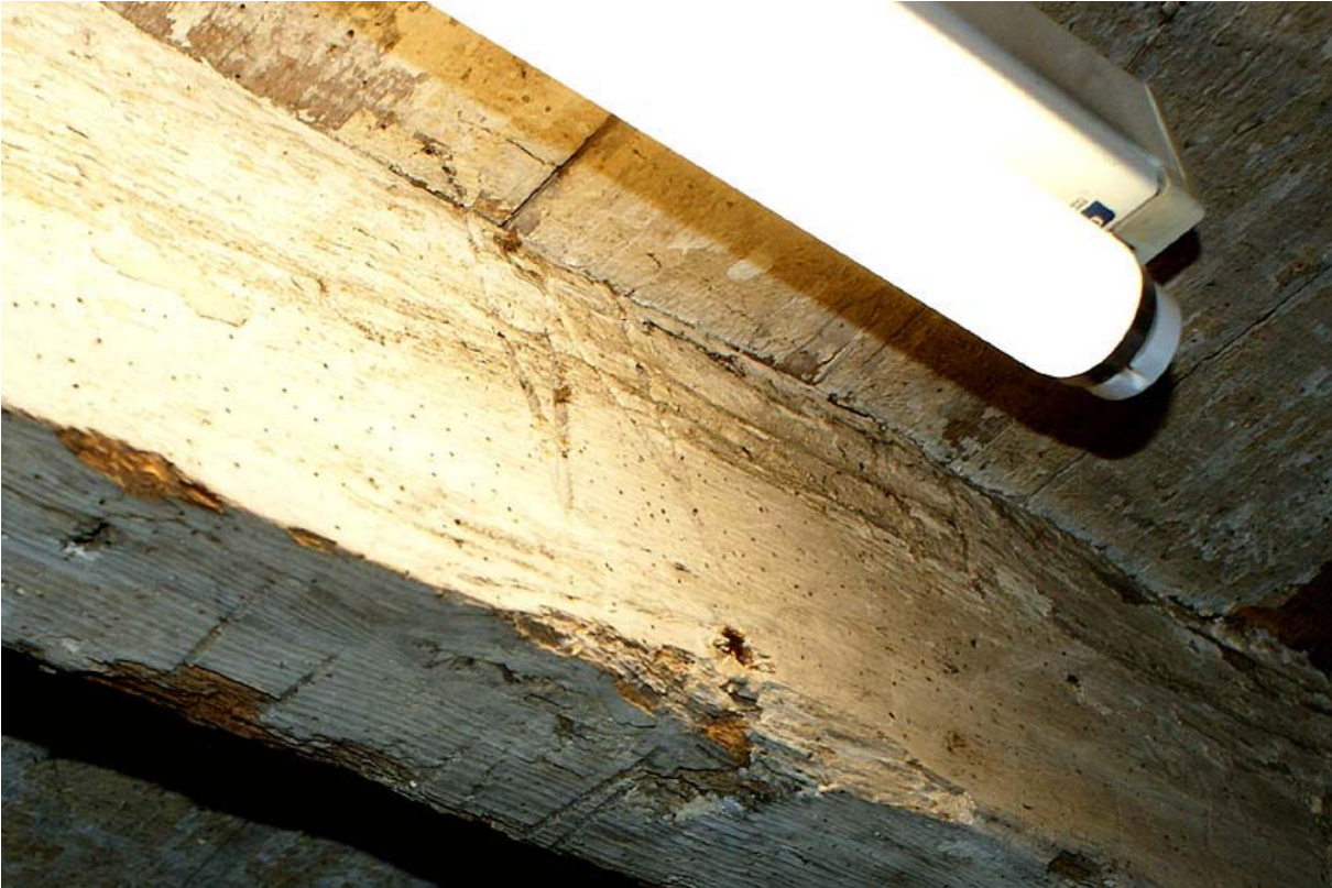
Plate 38: Possible apotropaic mark on cellar ceiling joist (with Baltic timber marks on below face of timber)
