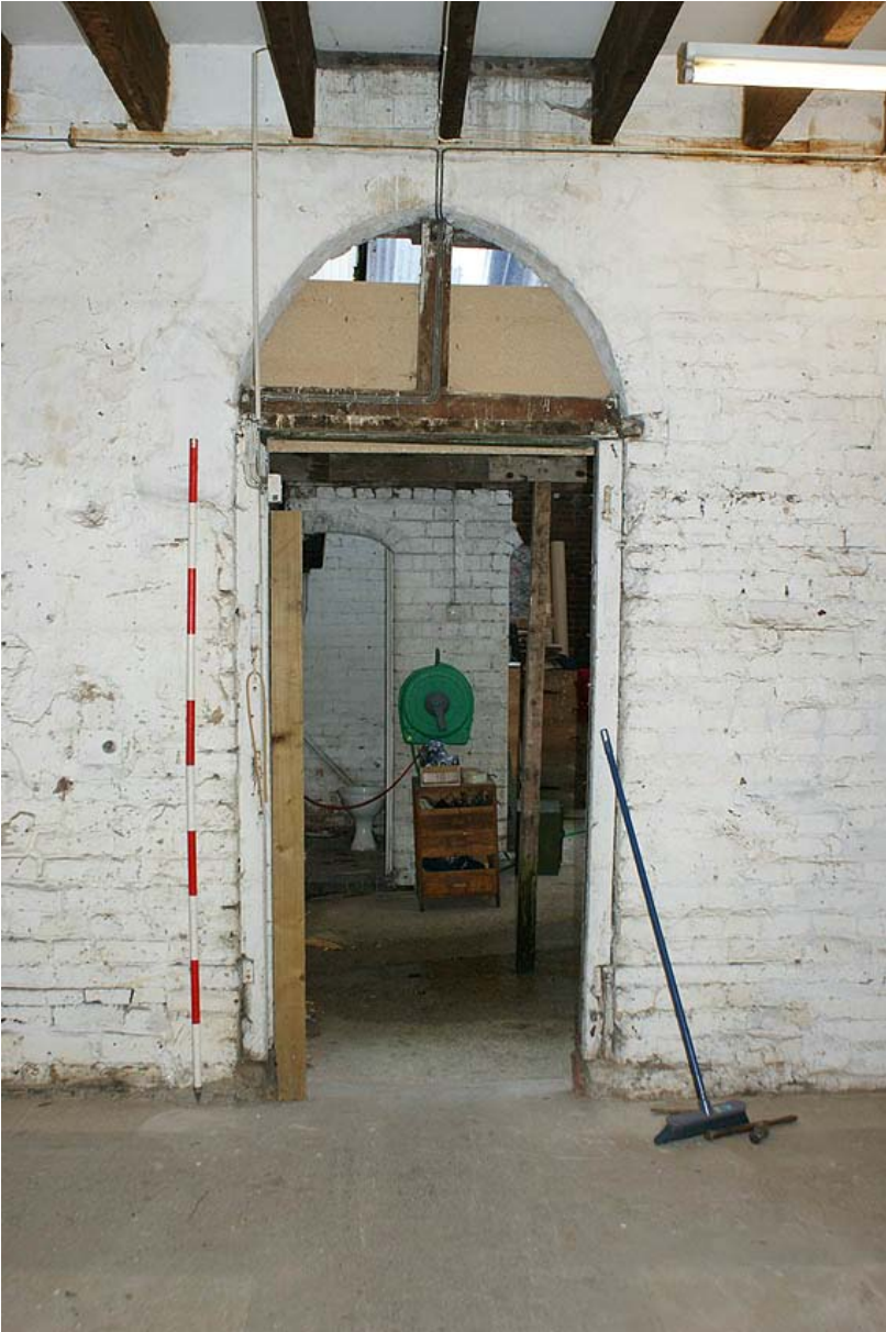
Plate 4: Ground floor door of the stable
