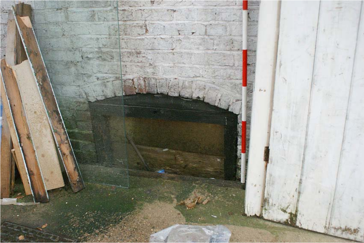
Plate 17: Cellar window of the warehouse
