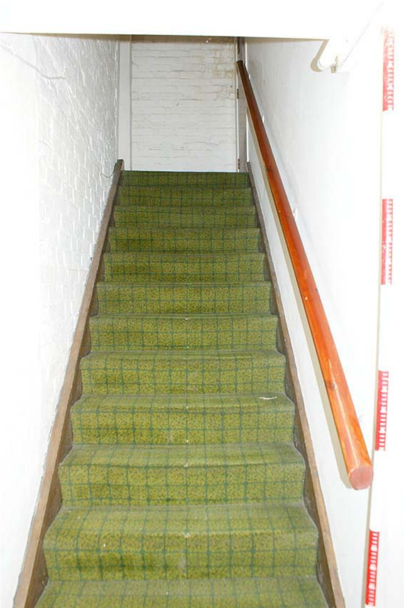
Plate 18: Warehouse ground to first floor stairs from the south west
