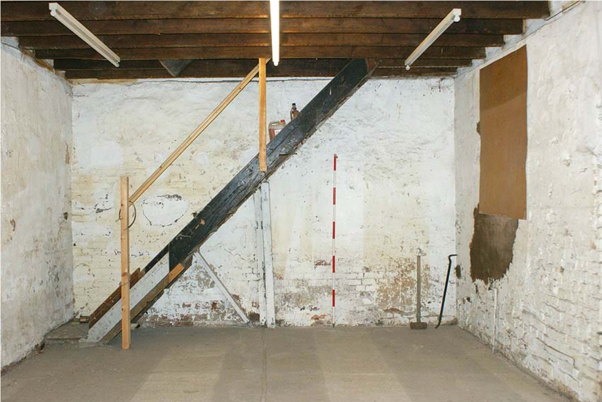
Plate 9: Interior of stable ground floor from the south east
