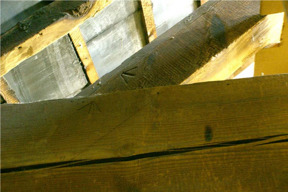
Plate 28: Example of carpenter's marks in the warehouse
