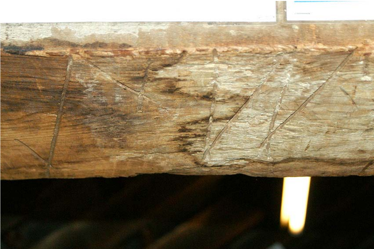
Plate 35: Baltic timber marks on tie beam in warehouse
