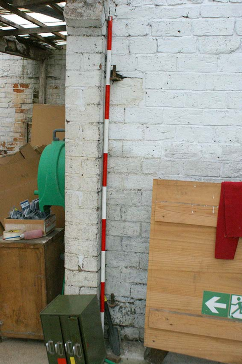
Plate 31: Hinge hooks behind jamb of arch springer from the east
