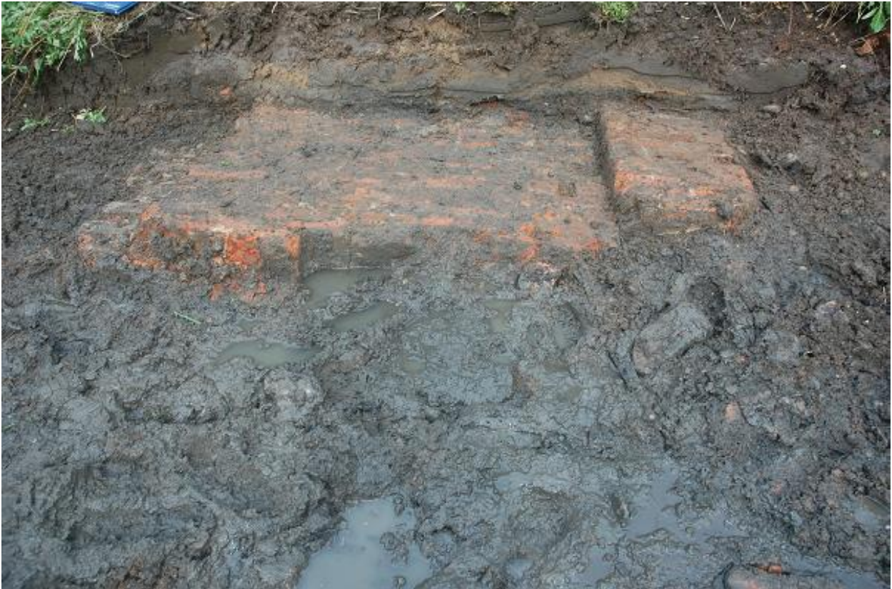
Plate 4 Collapsed wall (2004), looking north
