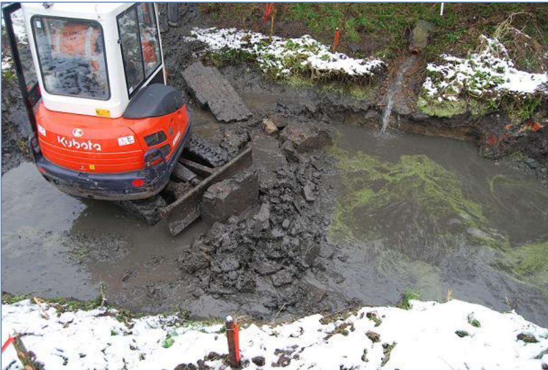
Plate 12 Removing the collapsed wall from the pond seen during the previous works, view north
