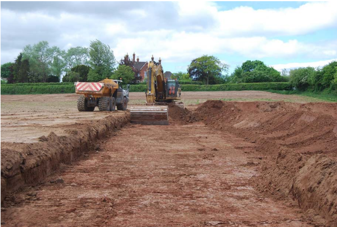
Plate 3: Stripping in Phase 2 (facing west)
