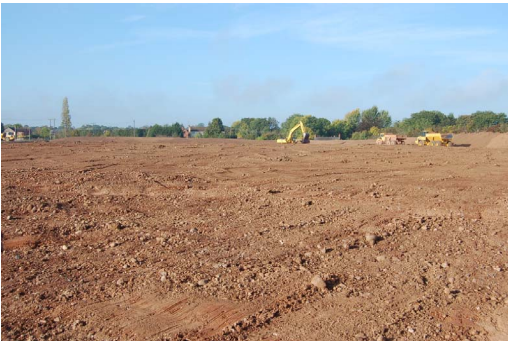
Plate 2: Phase 1 during excavation strip (facing south-west)
