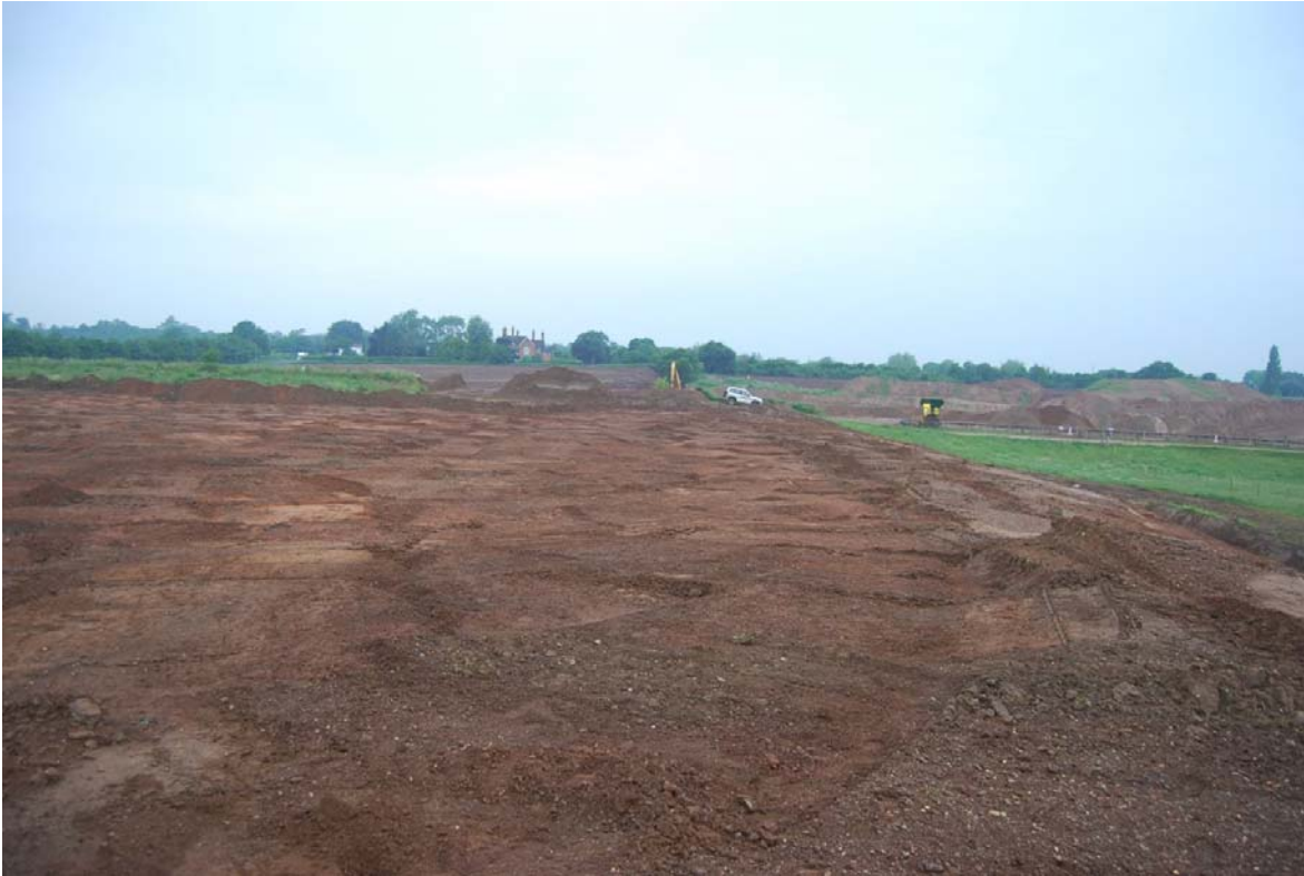
Plate 4: Stripping in Phase 3 (facing west)
