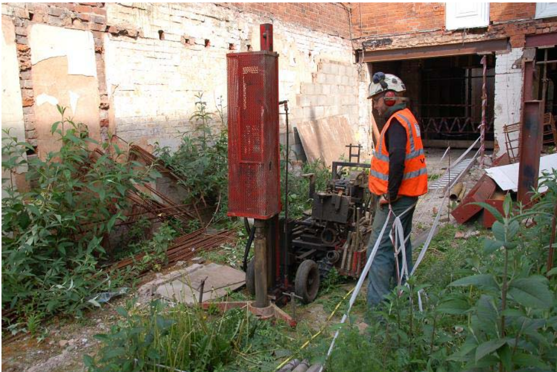
Plate 2 The percussive rig in use
