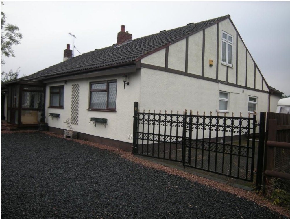
Plate 1, Bungalow at Little Acre, facing south-west
