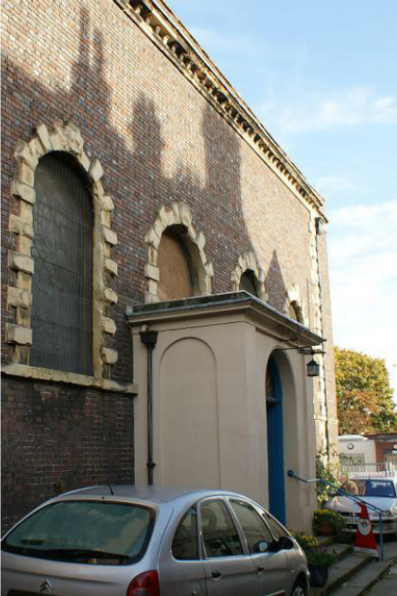
Plate 16: 1820s porch from the south west
