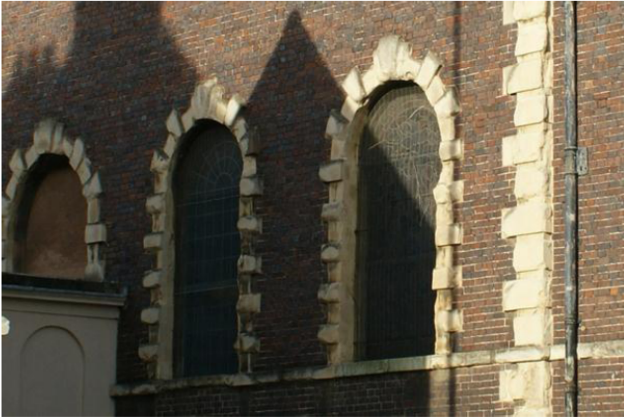
Plate 8: Semi-circular windows and surrounds, from the south east
