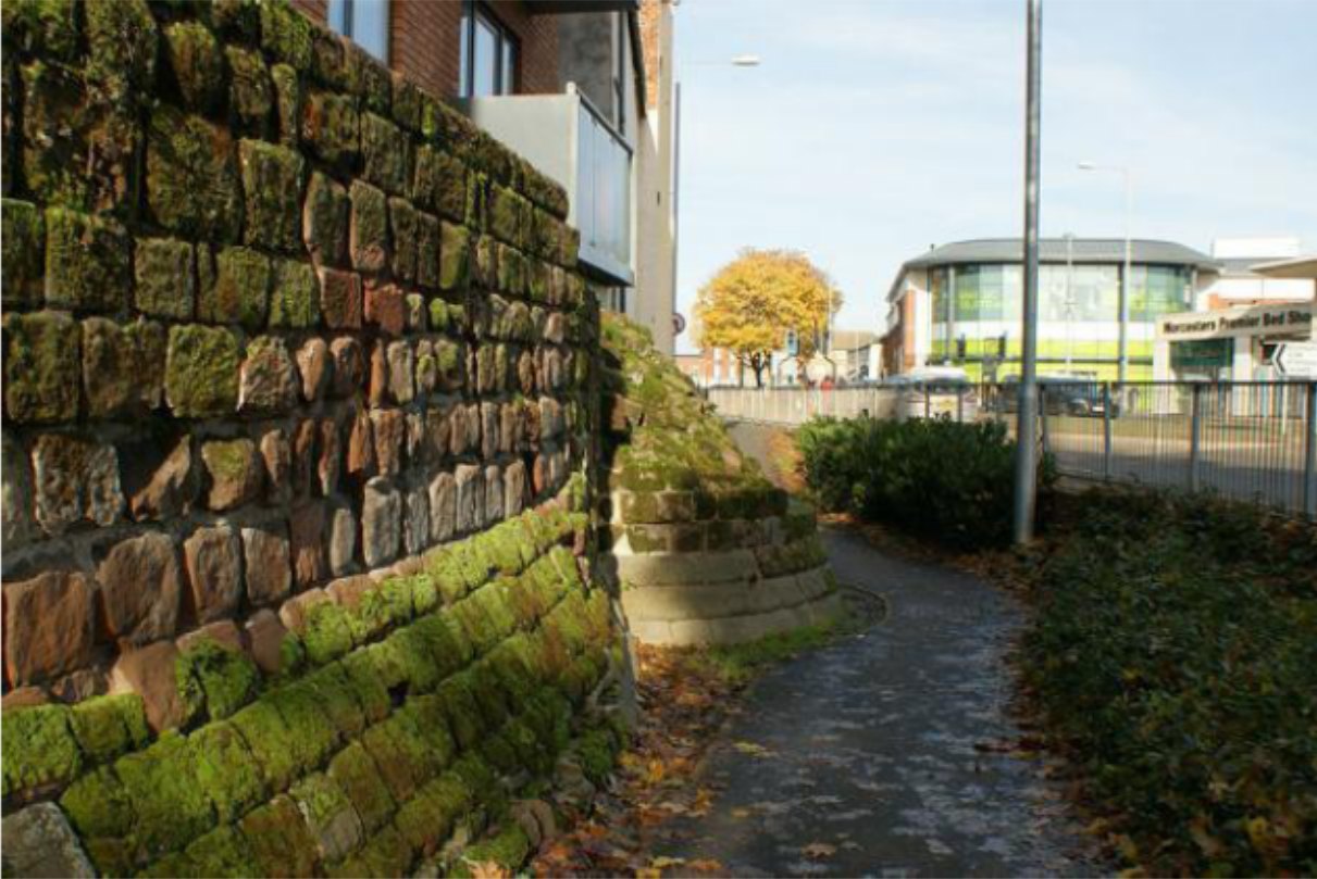
Plate 27: Listed City Wall and bastion from the south
