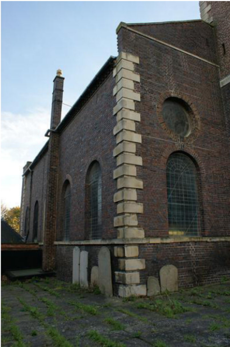
Plate 7: Stone quoins, from the north west
