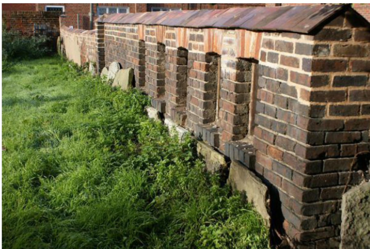
Plate 13: Churchyard walls, from the east
