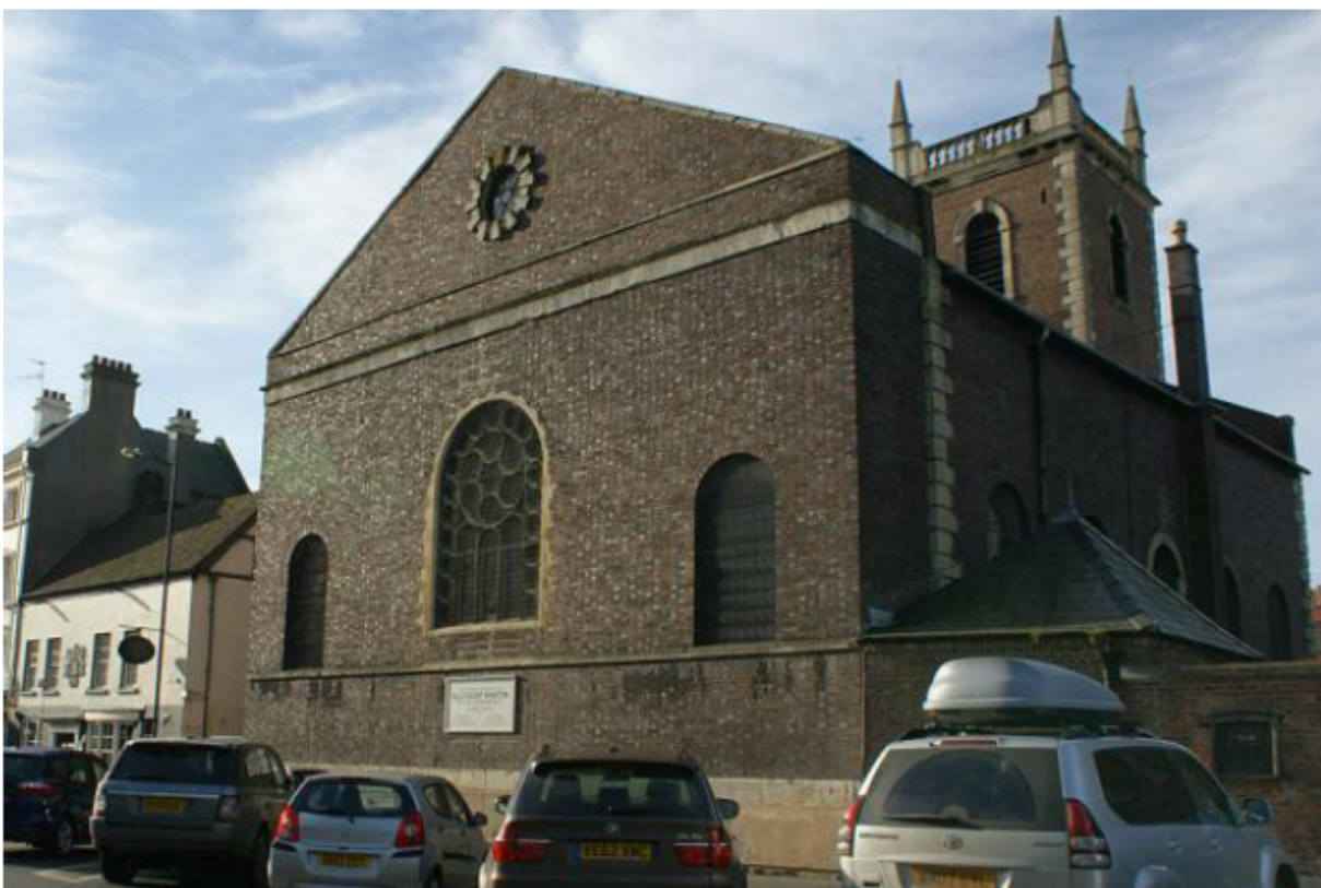
Plate 4: Old St Martin's Church showing brickwork
