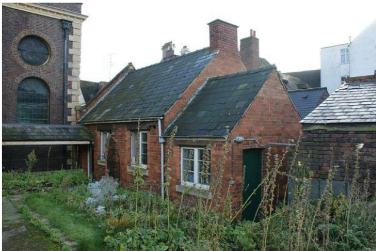
Plate 19: Parish rooms from the west
