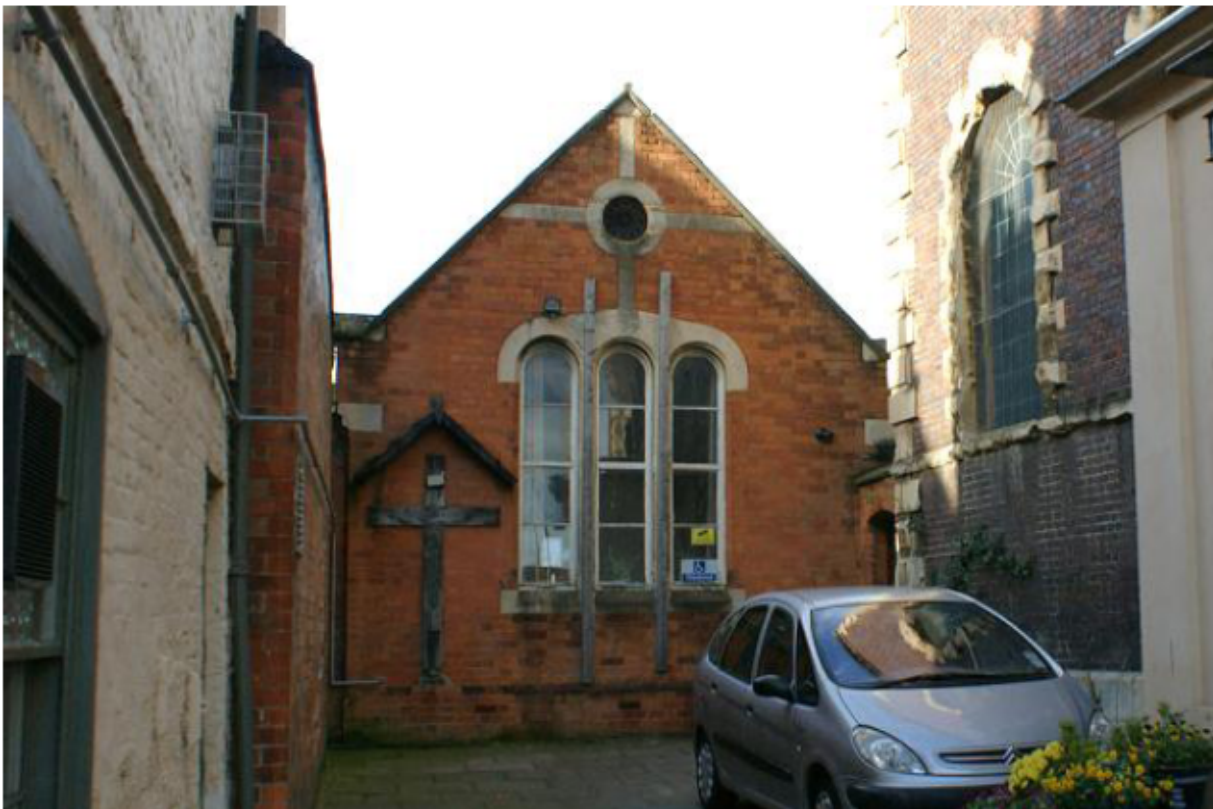
Plate 2: The parish rooms from the east
