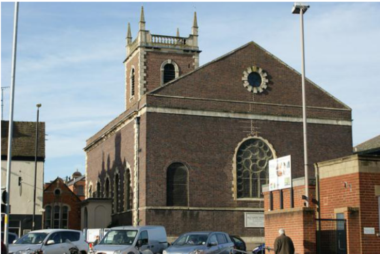
Plate 6: Old St Martin's Church showing five bays and tower
