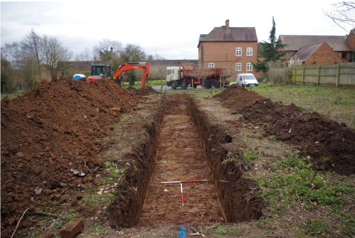
Plate 2: Natural deposits of weathered clayey mudstone were identified in Trench 1. Note the northern side elevation of the listed Grove Farm is clearly visible beyond the truck.
