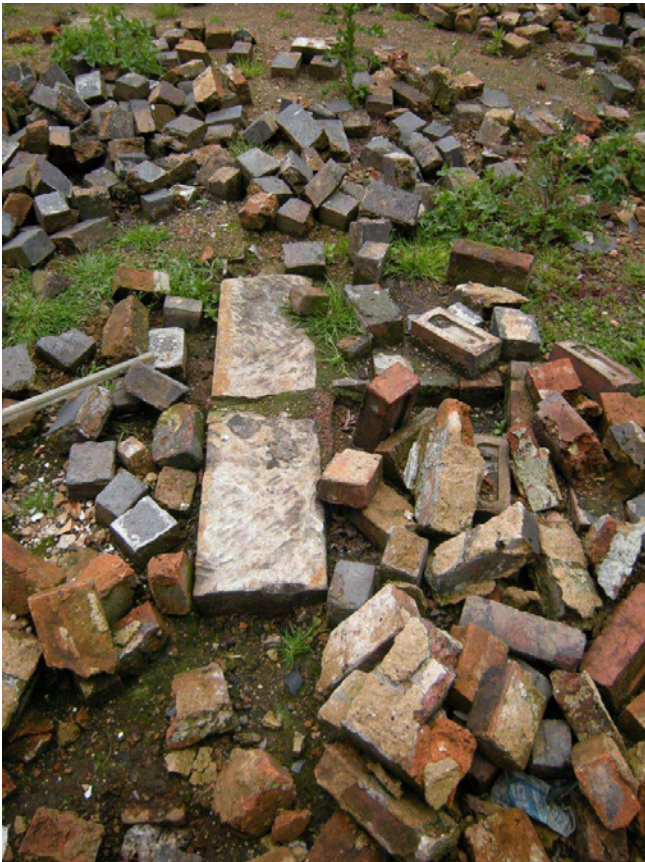
Plate 6 Wall footings from the east
