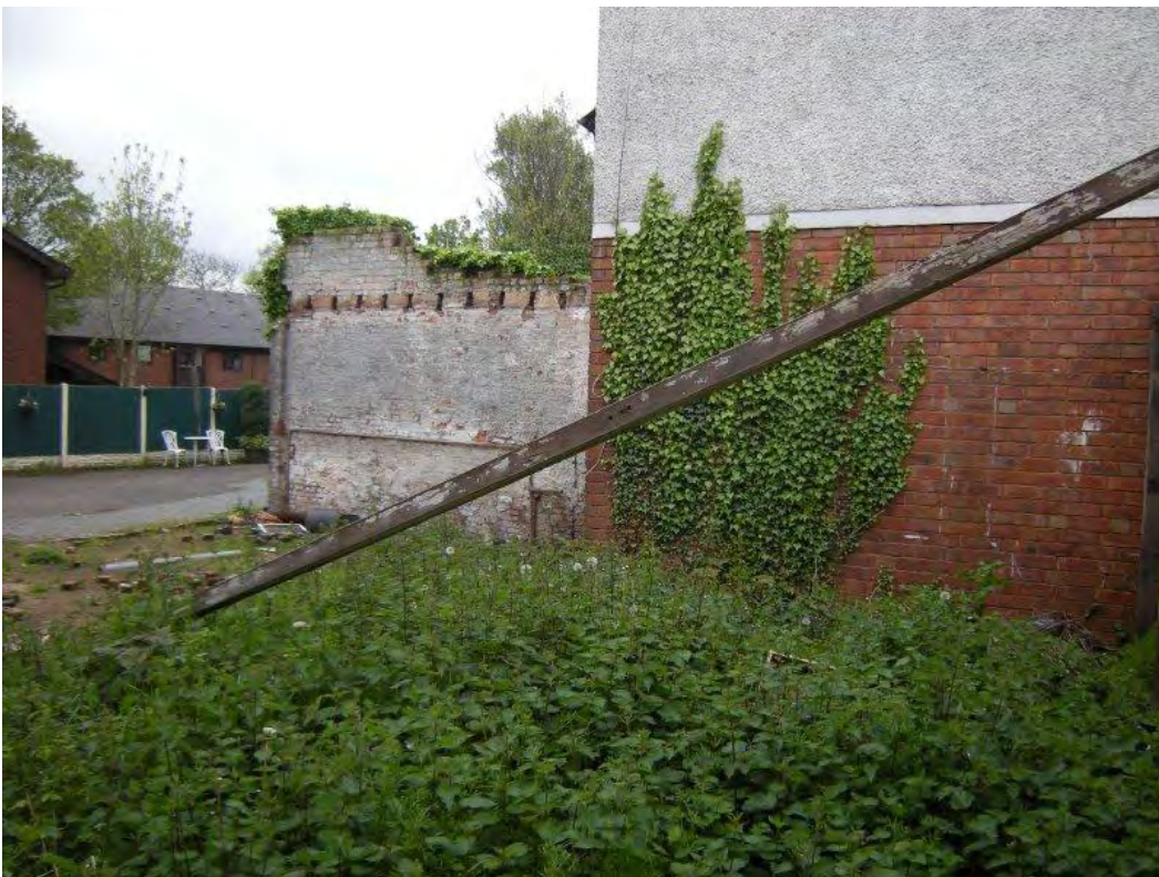
Plate 4 East facing wall of demolished buildings from the north-east
