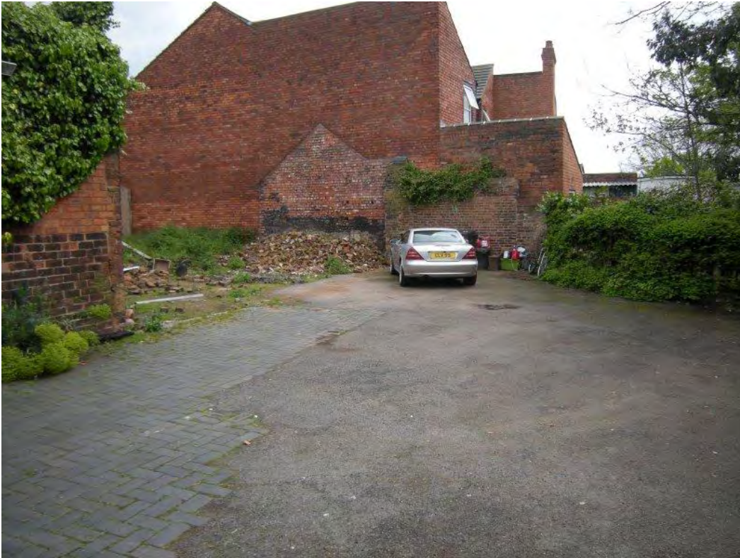
Plate 5 Relict outline of demolished building from the south-west showing brick west-facing inner wall.
