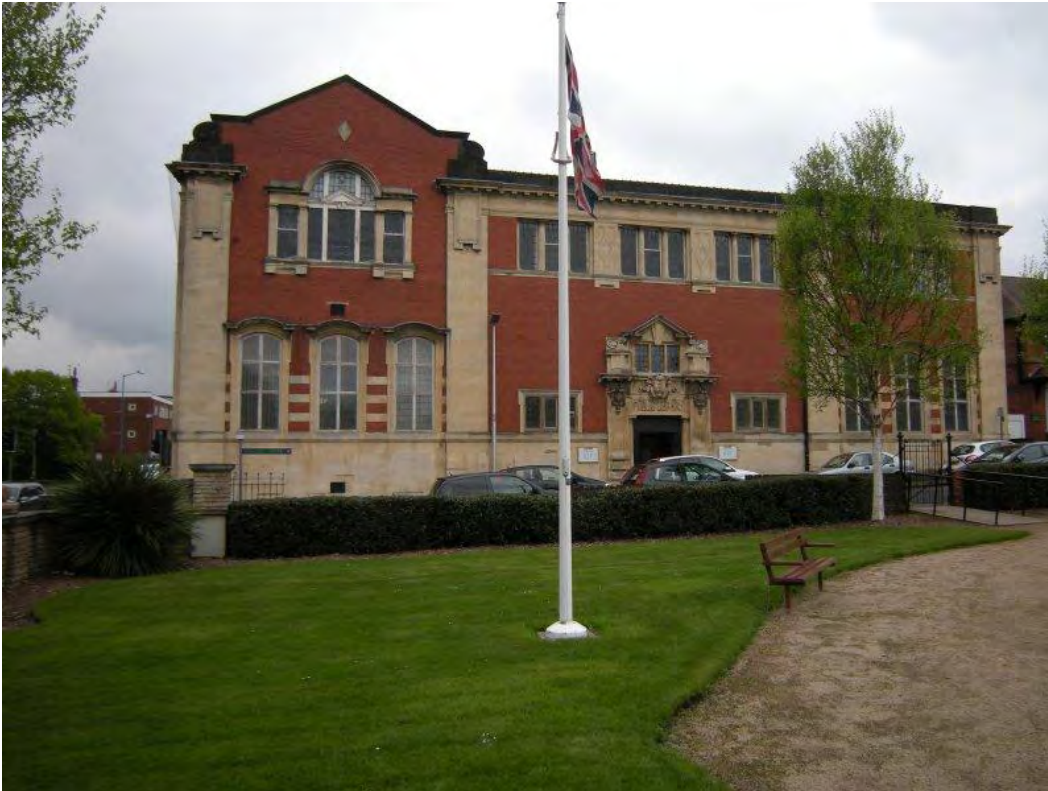
Plate 7 Wednesbury Public Library from the east
