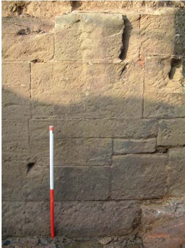
Plate 11: Detail of front face of 15 th century abutment (context 1606)
