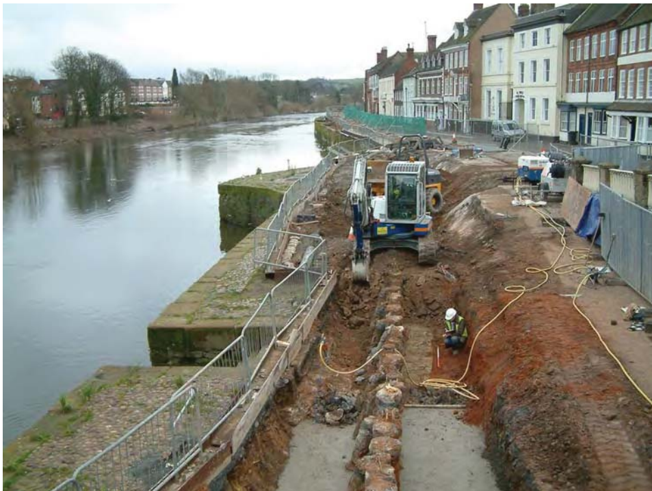
Plate 16: 17 th /18 th century wall in groundbeam trench near present bridge (context 2101)
