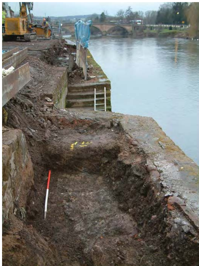
Plate 14: ?15 th century quay wall (context 7009)
