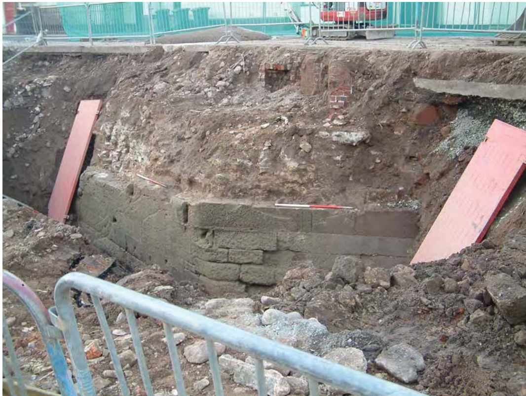
Plate 9: 15 th century bridge abutment, facing south-east
