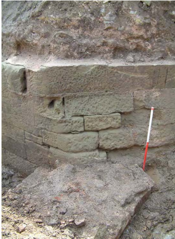
Plate 15: Wall abutting north west side of 15 th century bridge abutment (context 1607)
