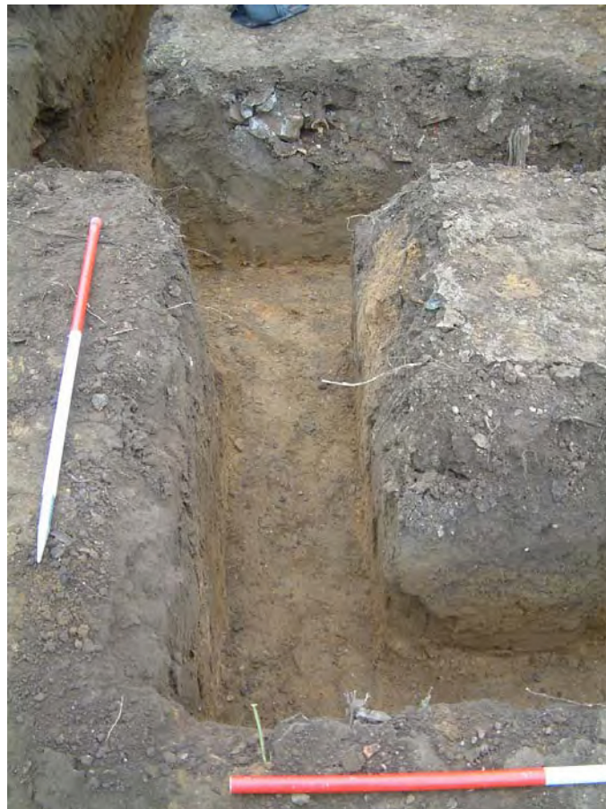
2. Sample of southern foundation trenches, view west
