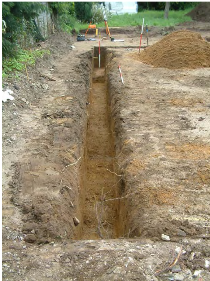
3. Eastern foundation trench, view south
