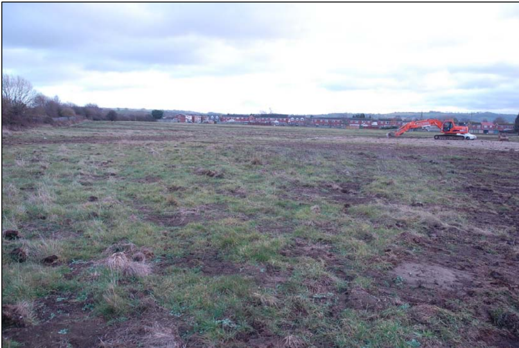
Plate 7: Backfilled trenches (Trenches 2, 3, and 4 facing south)
