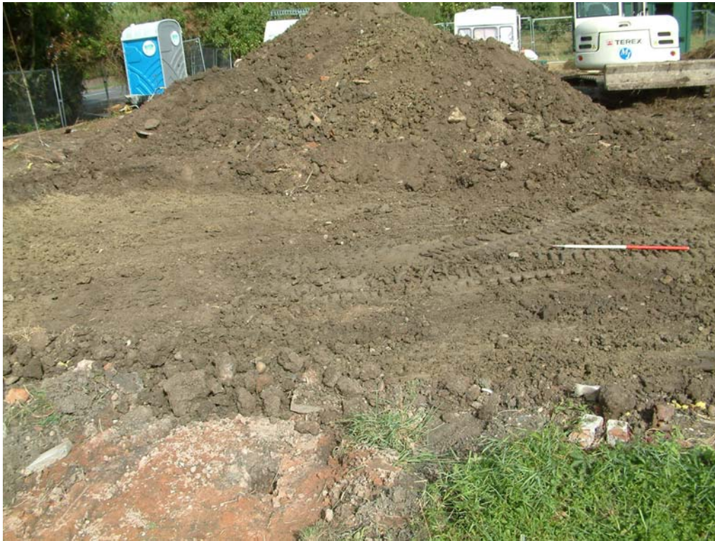
Plate 3, General view north of stripped area
