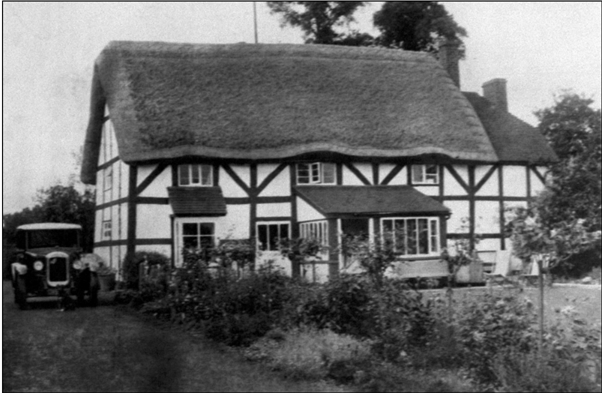
Figure 11: 1934 photograph showing cottage with sunroom and bay window extensions
