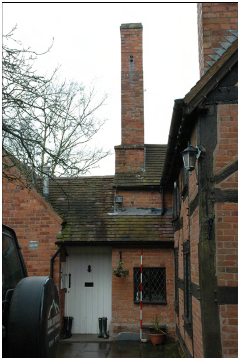
Figure 15: elevation of inglenook chimneystack enclosed by 1980s extension
