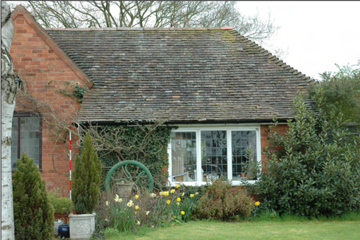
Figure 16: 1980s extension to rear of washhouse
