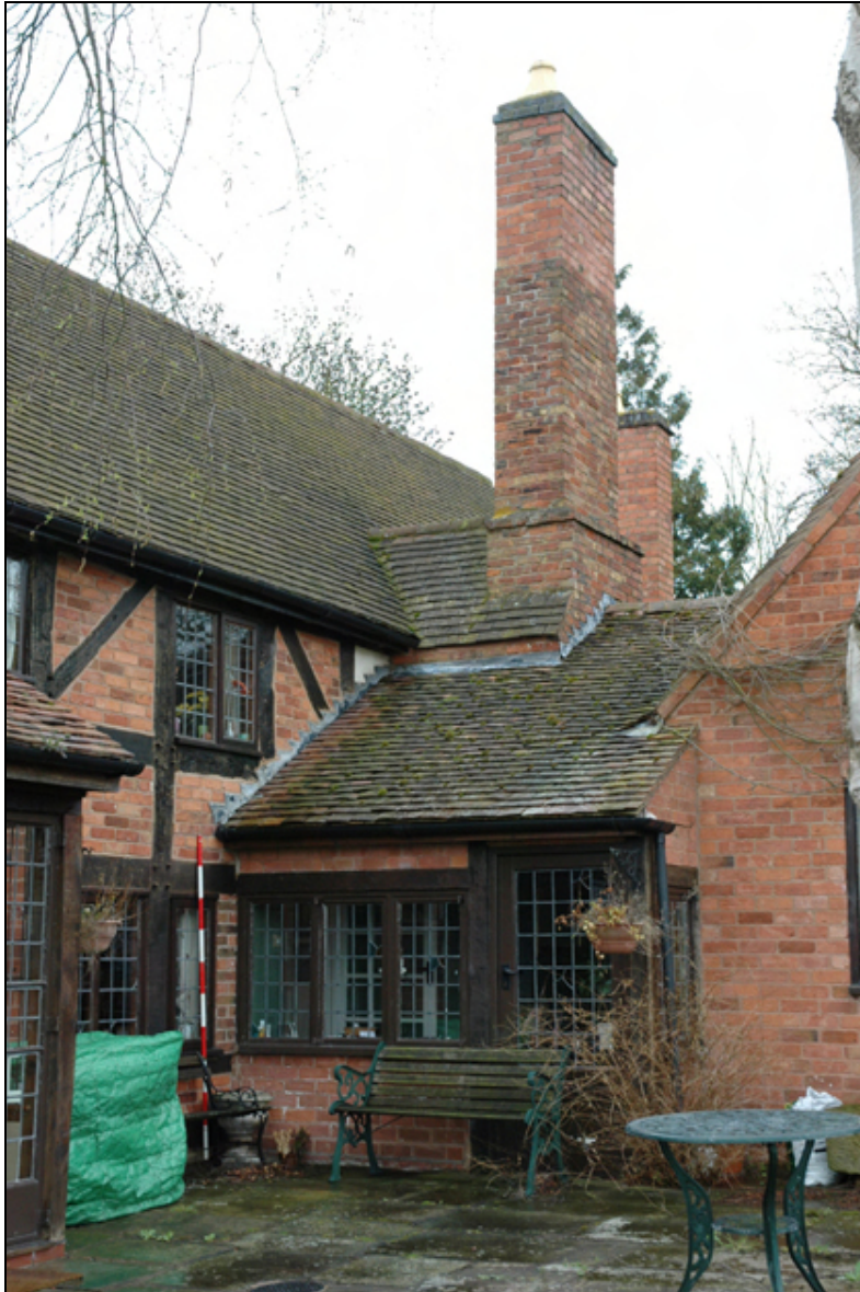
Figure 14: 1980s extension joining cottage to washhouse
