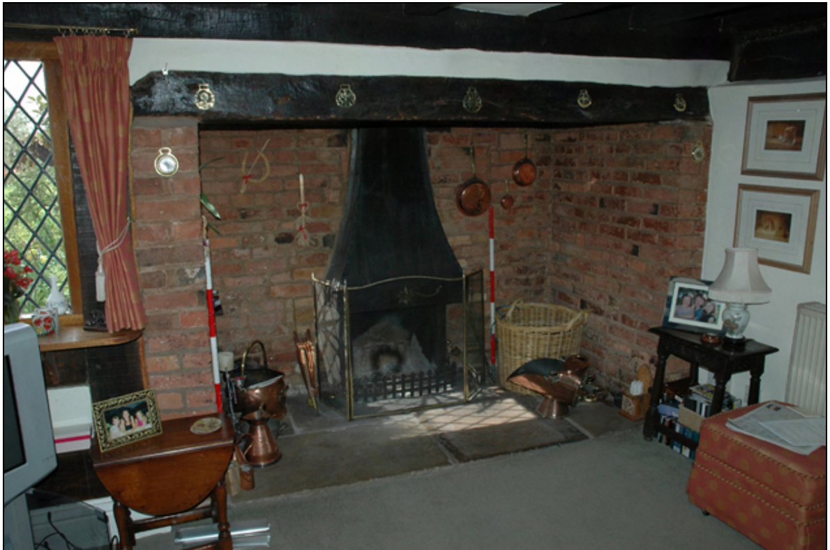
Figure 6: 1830s inglenook fireplace in main ground floor room of cottage
