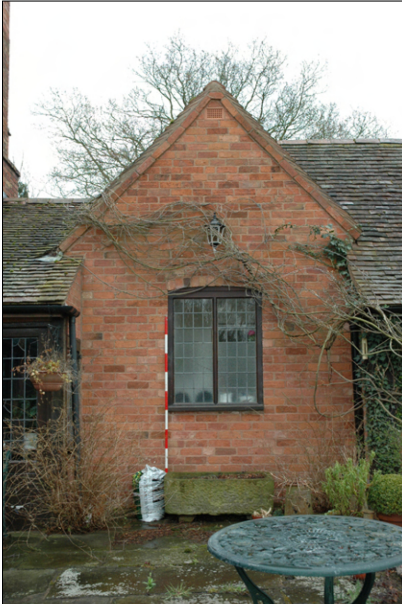
Figure 8: 1890s washhouse extension
