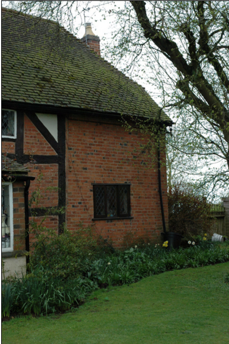
Figure 4: 1830s extension to cottage
