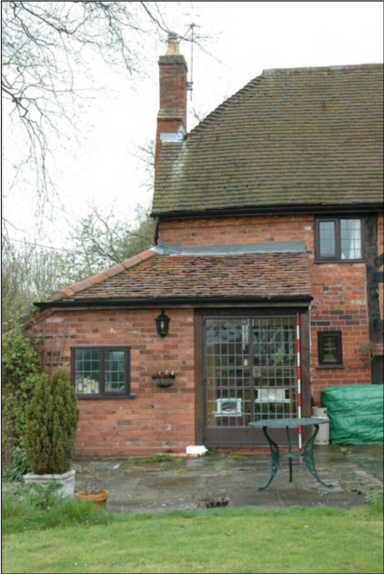
Figure 13: 1980s extension to west gable of cottage
