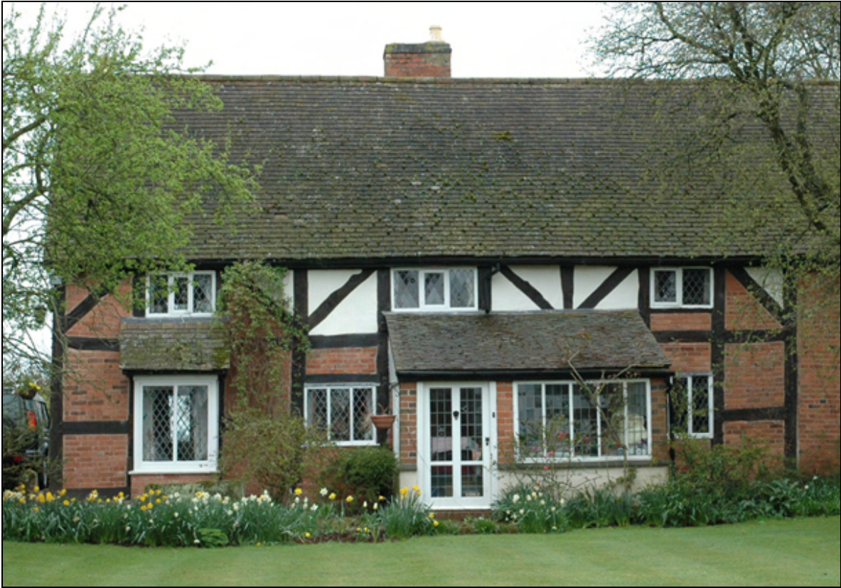
Figure 3: Three bay timber framed 17 th century cottage
