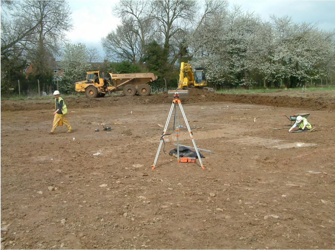
Plate 9. Work in progress, the site from the south east.
