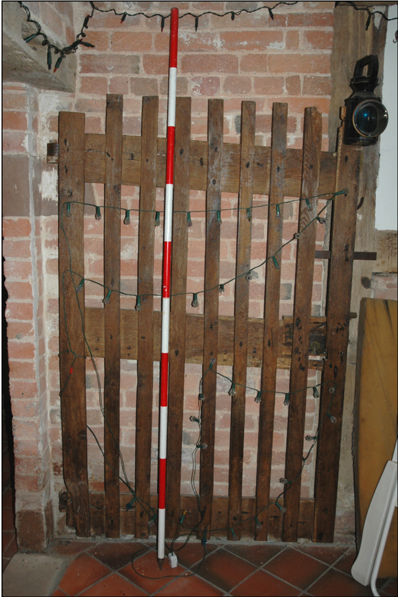
Figure 16: Gate at entrance to large cellar room
