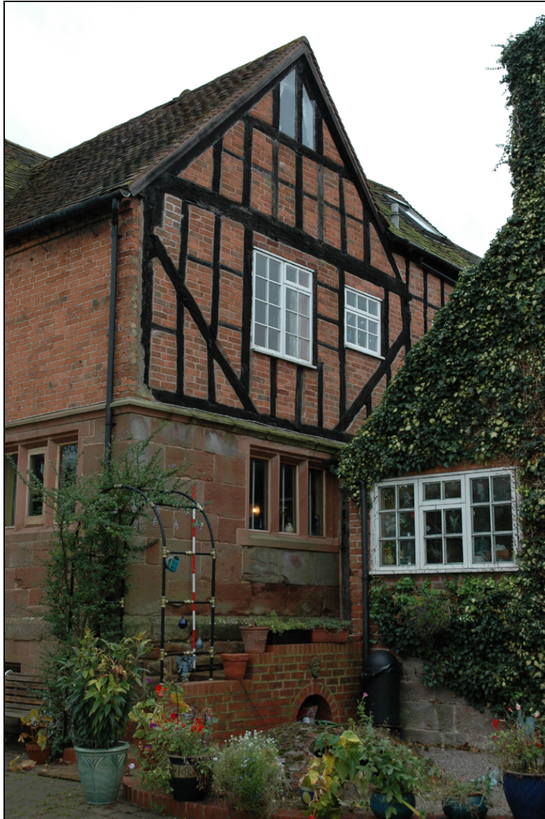
Figure 7: Ridgeway Court rear (north) elevation showing close studding
