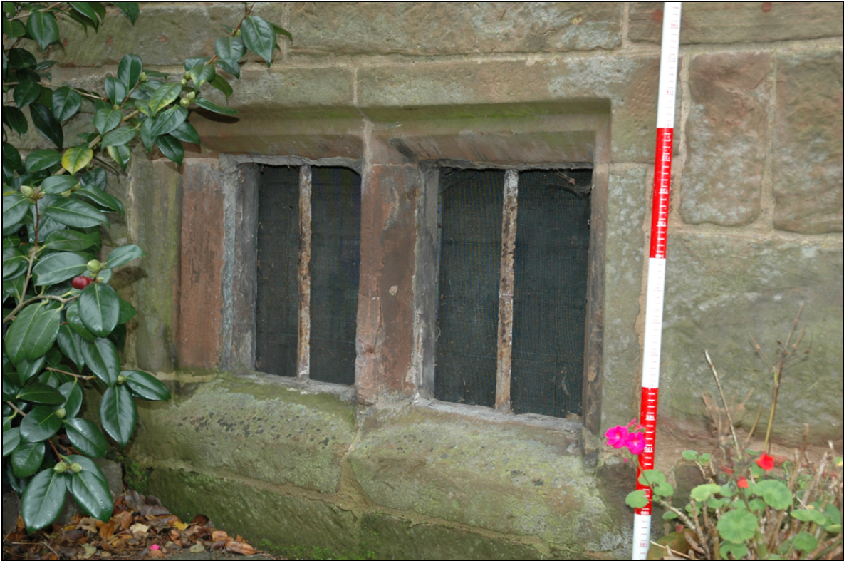
Figure 9: Sandstone, mullion window dating to 16 th century
