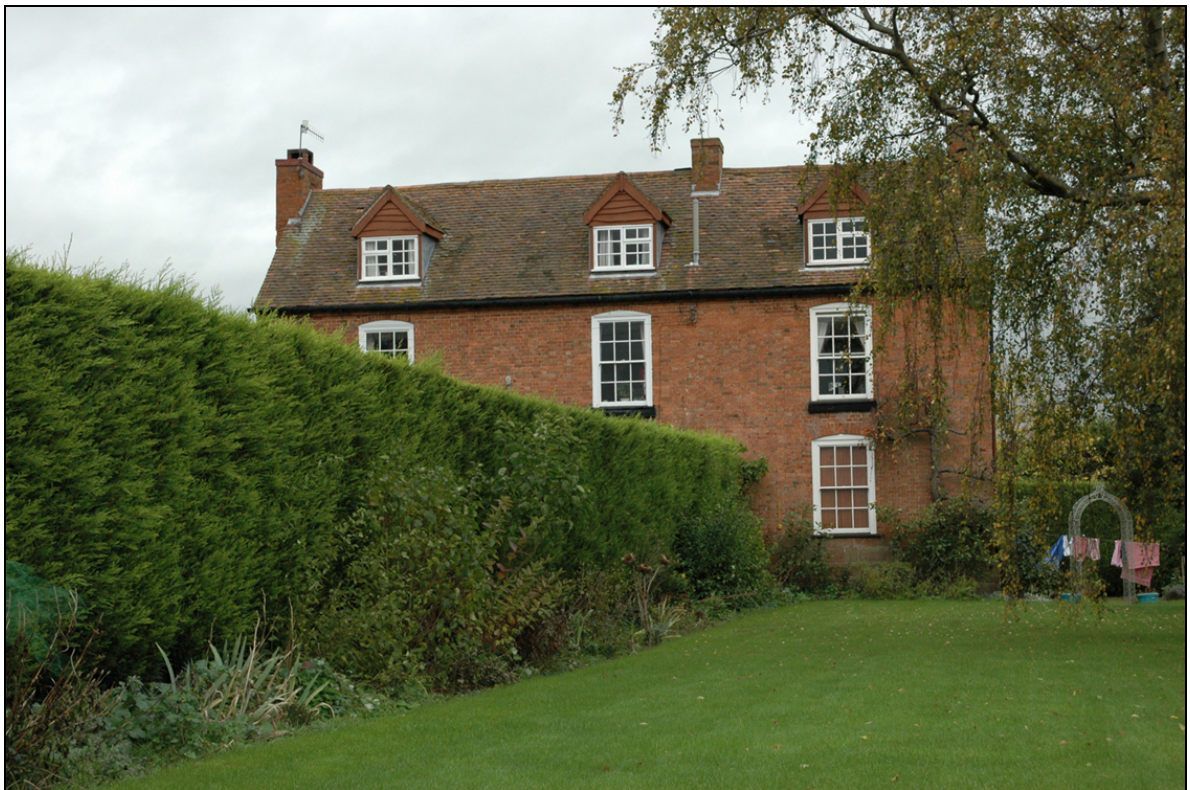
Figure 3: Frontage (south), of Ridgeway Court showing division of house
