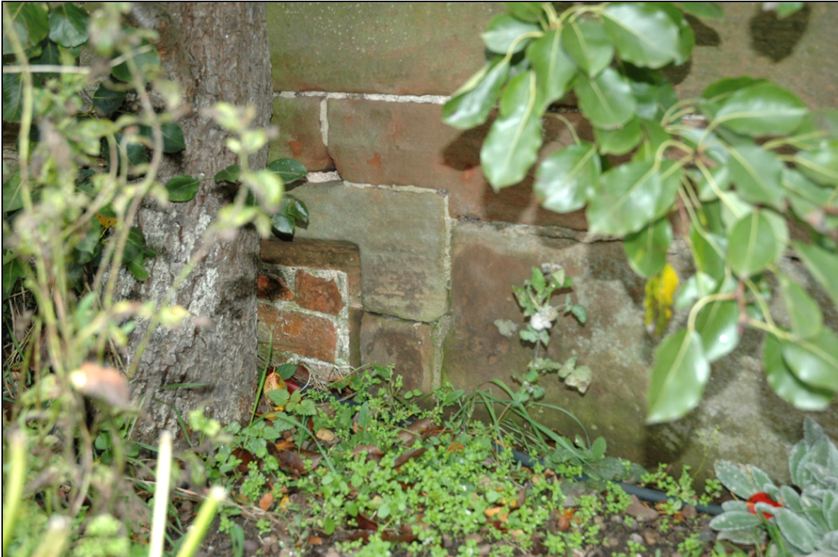
Figure 14: Blocked window on the south elevation
