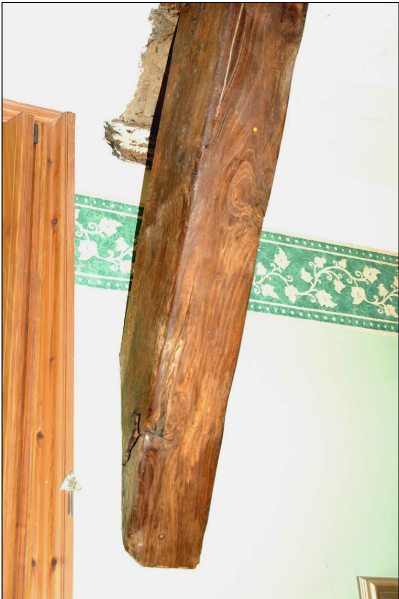
Figure 12: Beam cut off when south wall replaced
