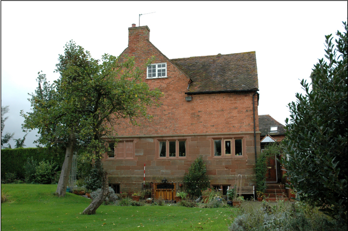
Figure 8: East elevation of Ridgeway Court showing sandstone walls
