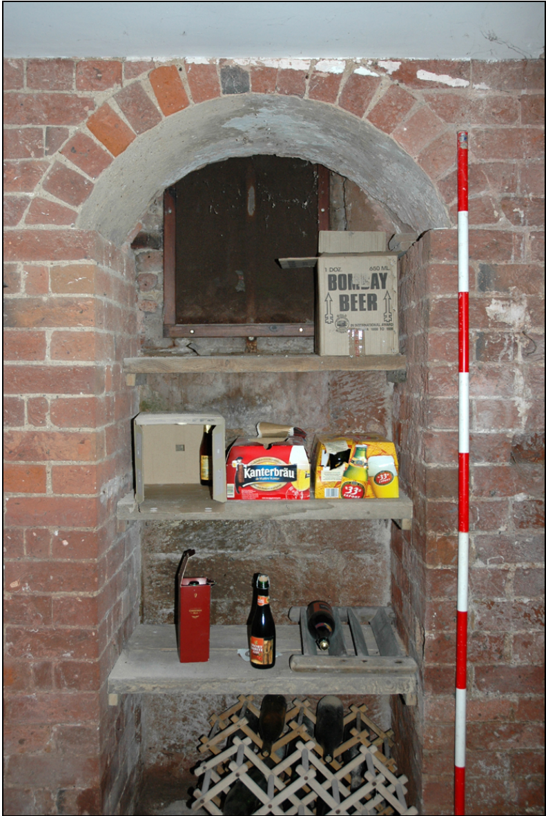
Figure 18: Fireplace in dairy in cellar
