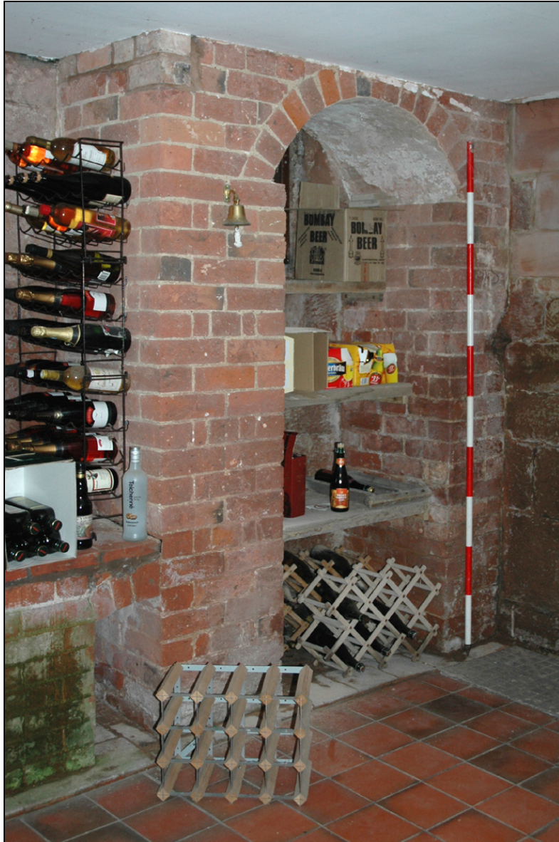
Figure 19: Dairy fireplace showing where it has caused the removal of the dairy cold shelf (bottom left)
