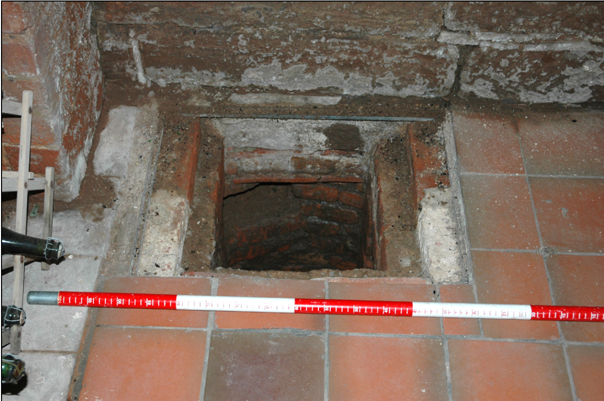
Figure 17: Water sump in dairy in cellar
