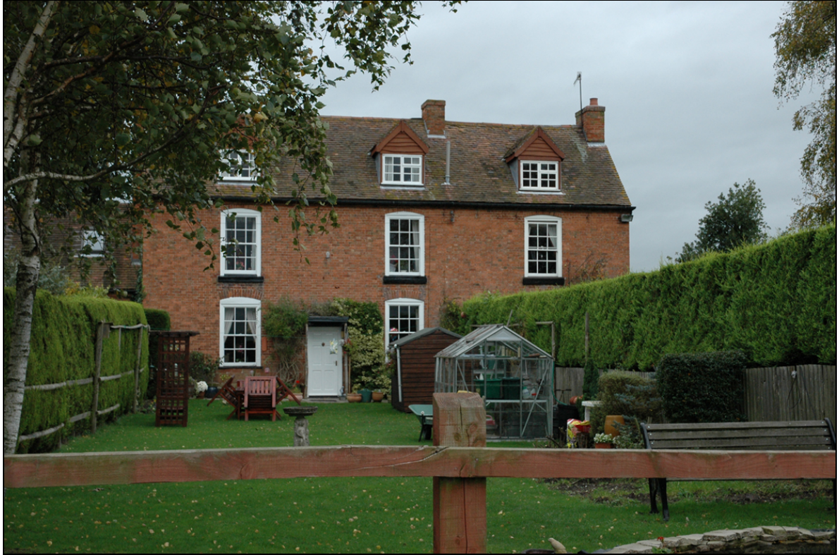
Figure 2: Frontage (south), of Ridgeway Court showing division of house
