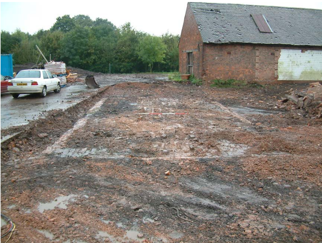
Plate 2: General overview of Area 2 and foundations of structure 2007, facing west
