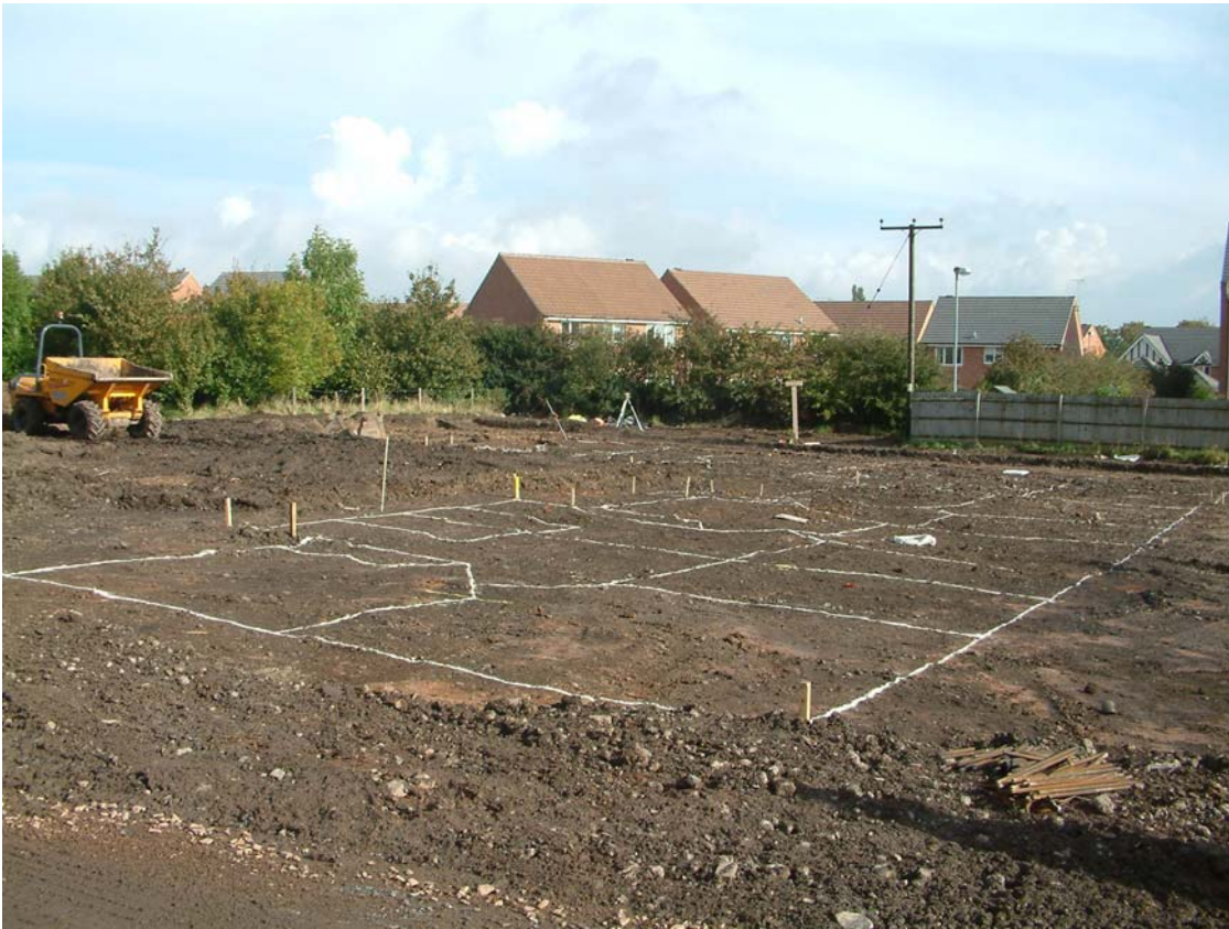
Plate 1: General overview of Area 1, prior to excavation, facing north-east
