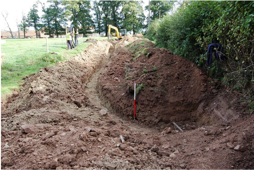
Plate 1: North West section of excavated pipe trench, showing original sewer pipe.
