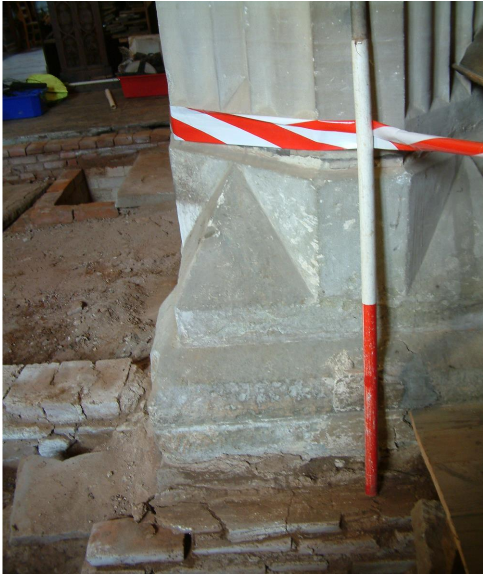
Plate 10: Base of nave column with possible earlier wall foundation at lower left corner (Facing south)
