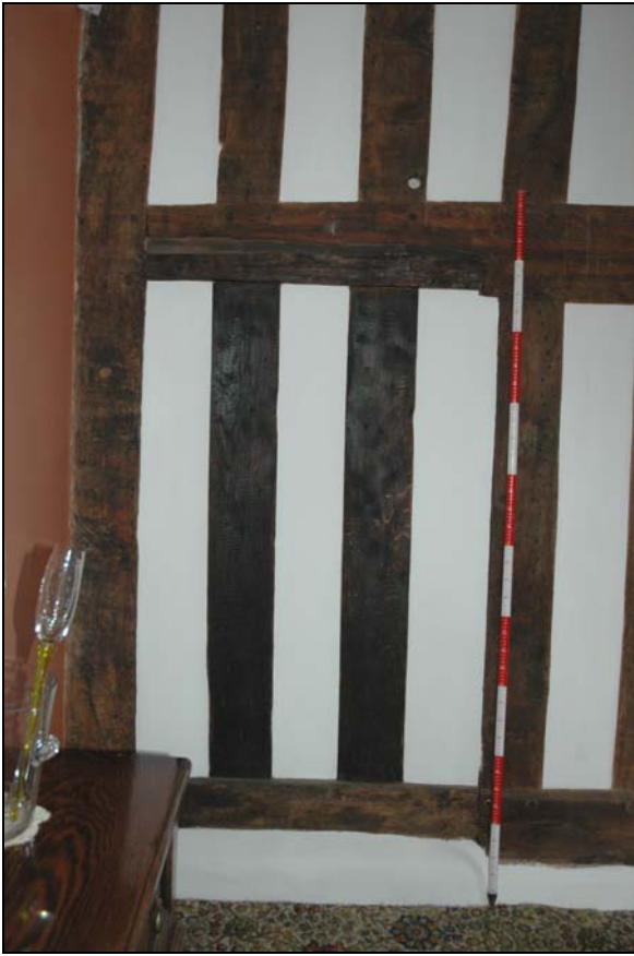
Figure 11: Former doorway now incorporated into the current dining room of the phase 3 building
