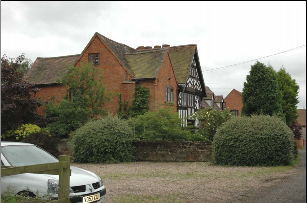
Figure 13: Different roof styles of the brick built north range phases 3 (gable) and 4 (left and right ridges)
