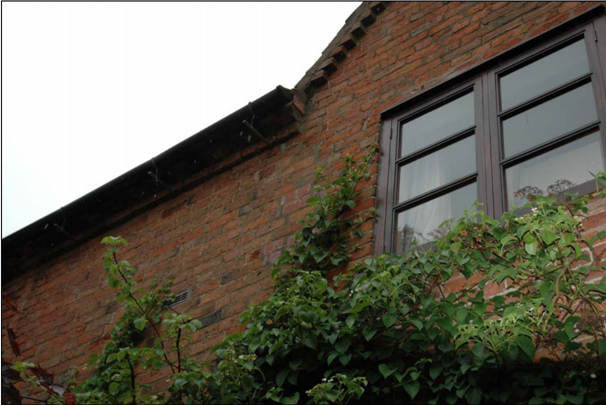
Figure 12: Building break showing east extension to the early 19 th century building
