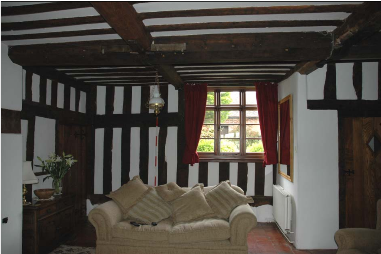
Figure 14: Drawing room timber beams
