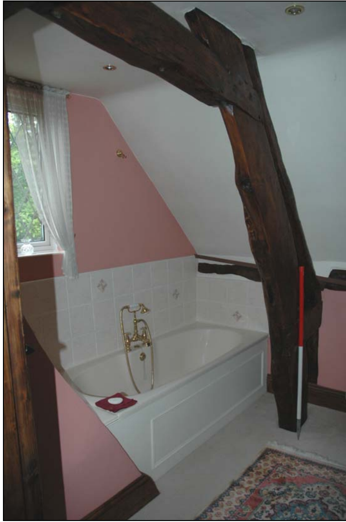
Figure 5: Cruck truss on first floor
