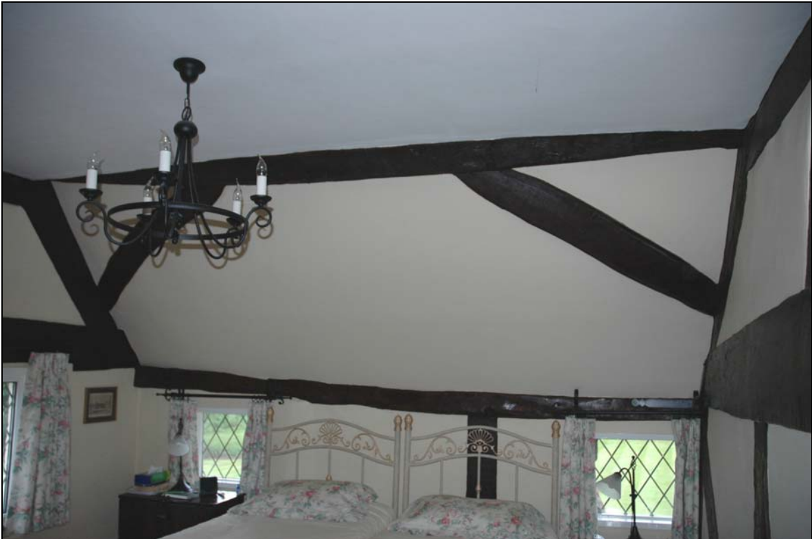
Figure 4: Wind braces in main bedroom
