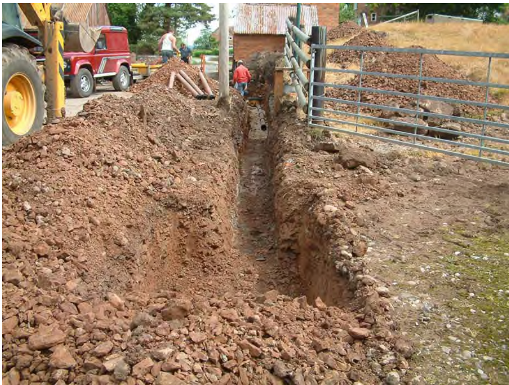
Plate 4 Trench 2, facing north
