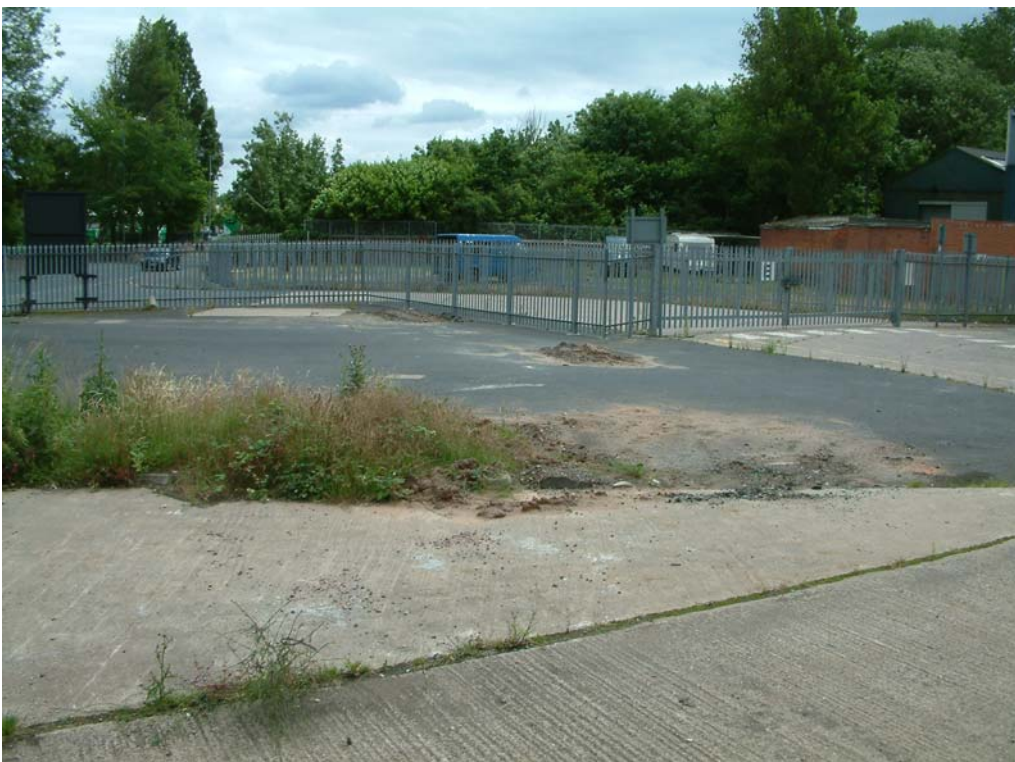
Plate 2: East entrance off Millfields Road, view north-east
