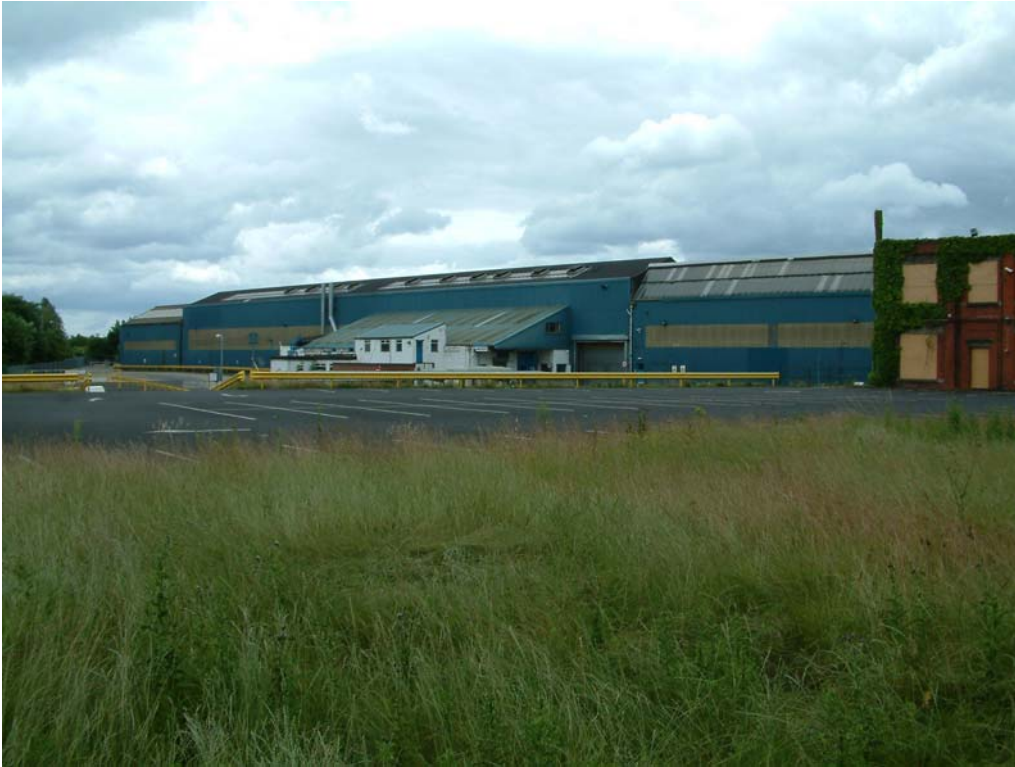
Plate 3: General view of site, south-east
