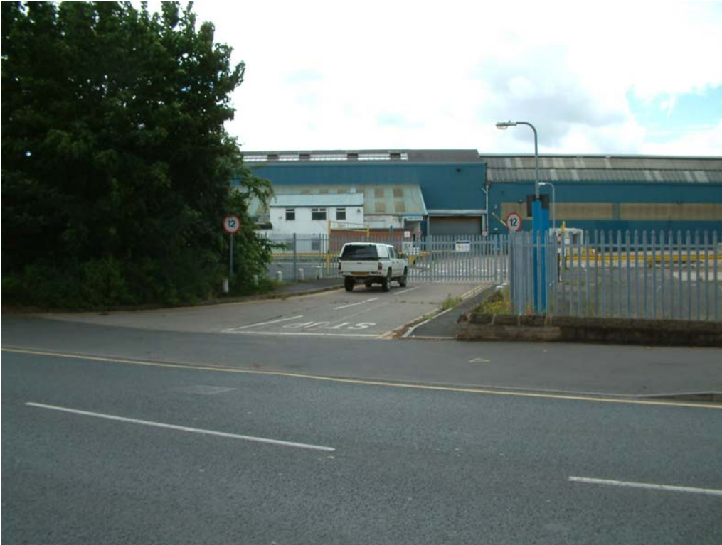
Plate 1: West entrance off Millfields Road, view south
