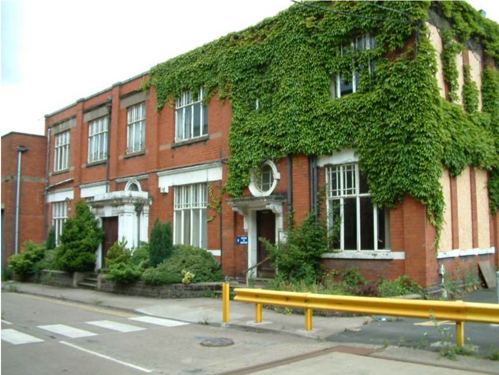
Plate 5: Office building on north side of Davis Street, view north-west
