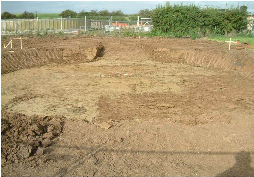
Plate 1. General view of trench 4, viewing west.
