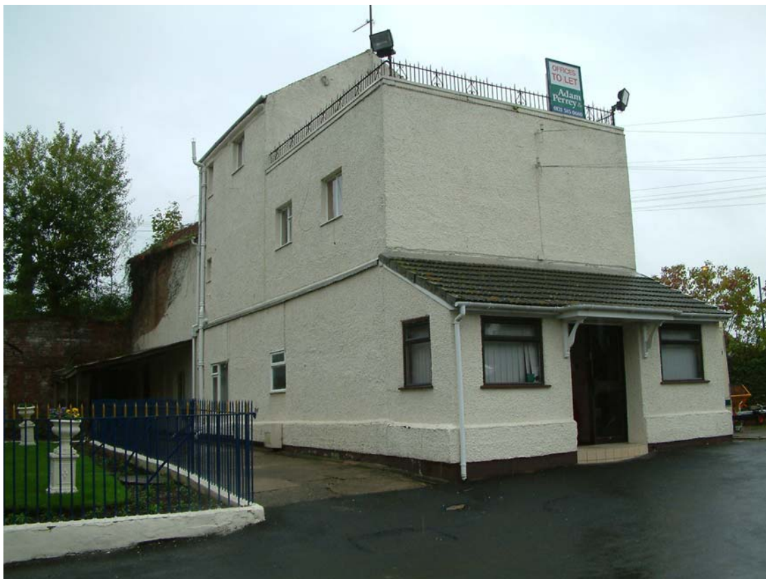
Plate 2 South and west elevations of the Engine House
