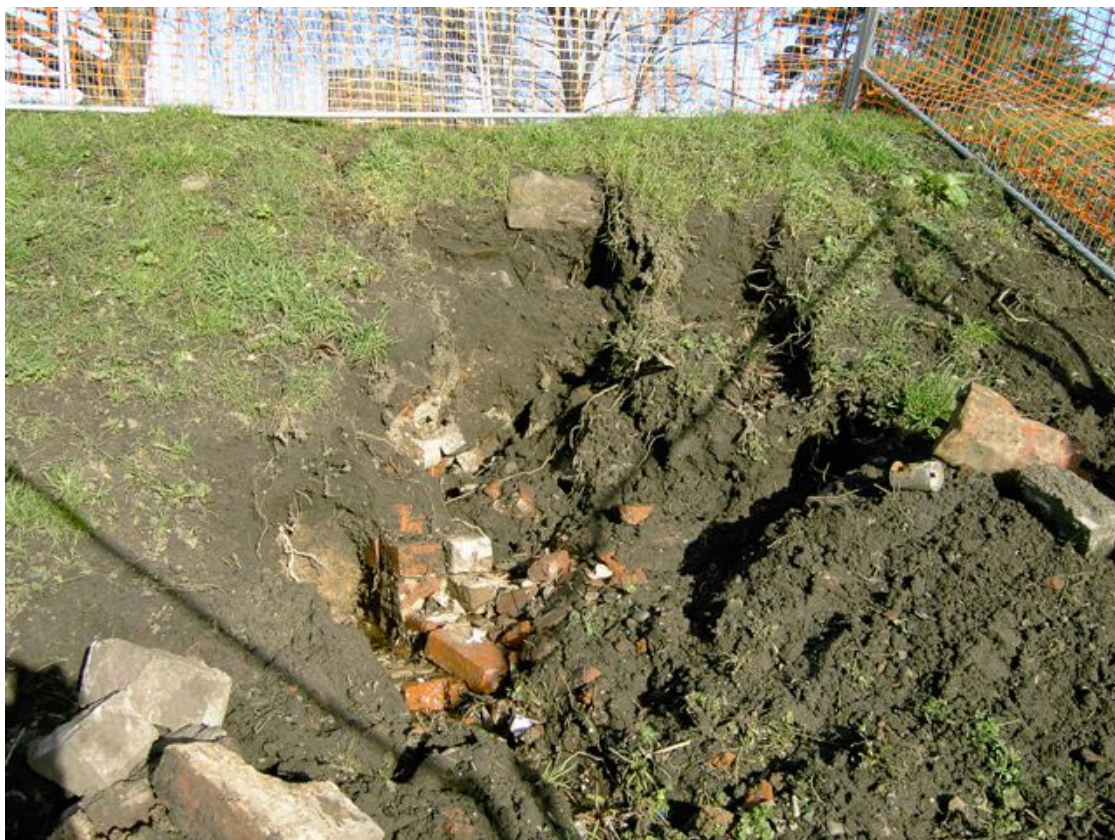
Plate 1 North wall and arch of the coal tunnel (British Waterways 2004)
