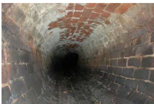
Plates 5 and 6, culvert structure running for Upper to Lower Basins, late 18 th century
