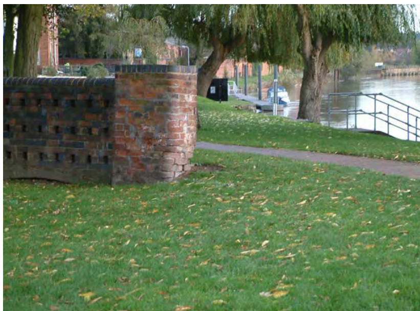
Plate 8, the existing dry dock wall
