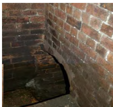
Plates 5 and 6, culvert structure running for Upper to Lower Basins, late 18 th century
