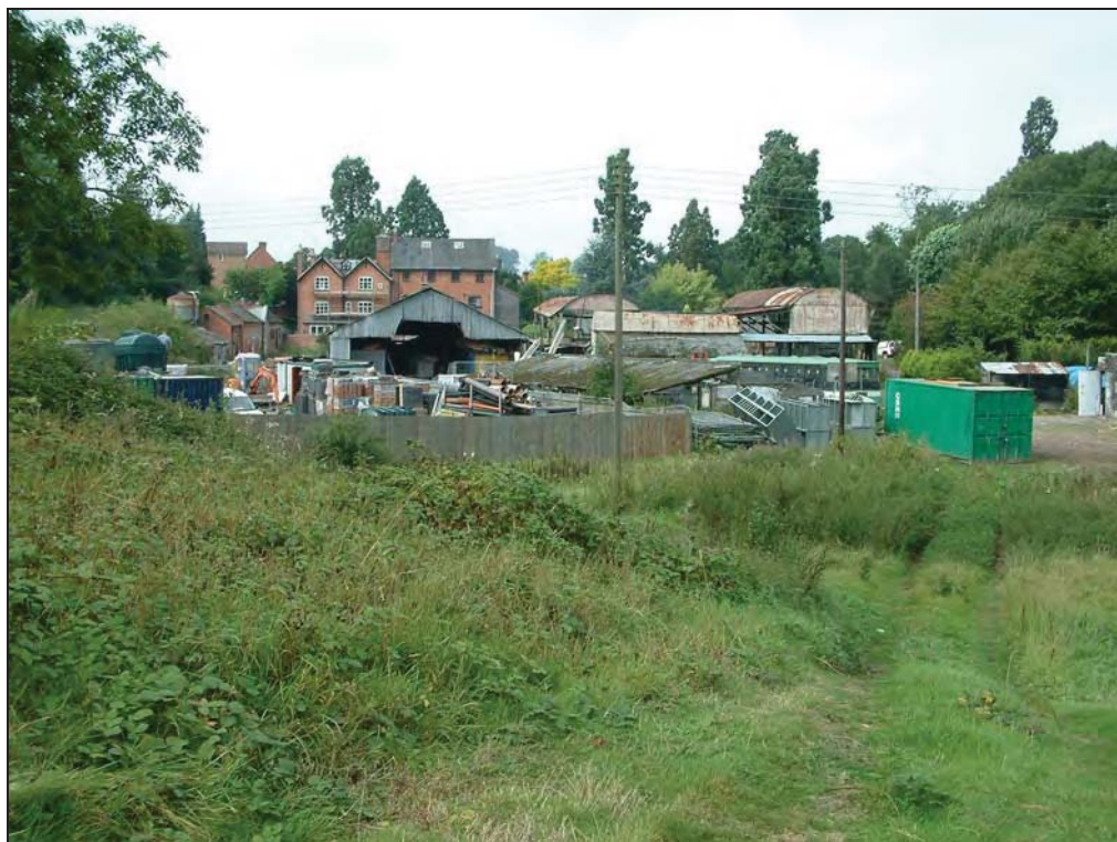
Plate 1: General view of the site from the south-west, before demolition and clearance. The taller brick building in the background is the former Town Mill
