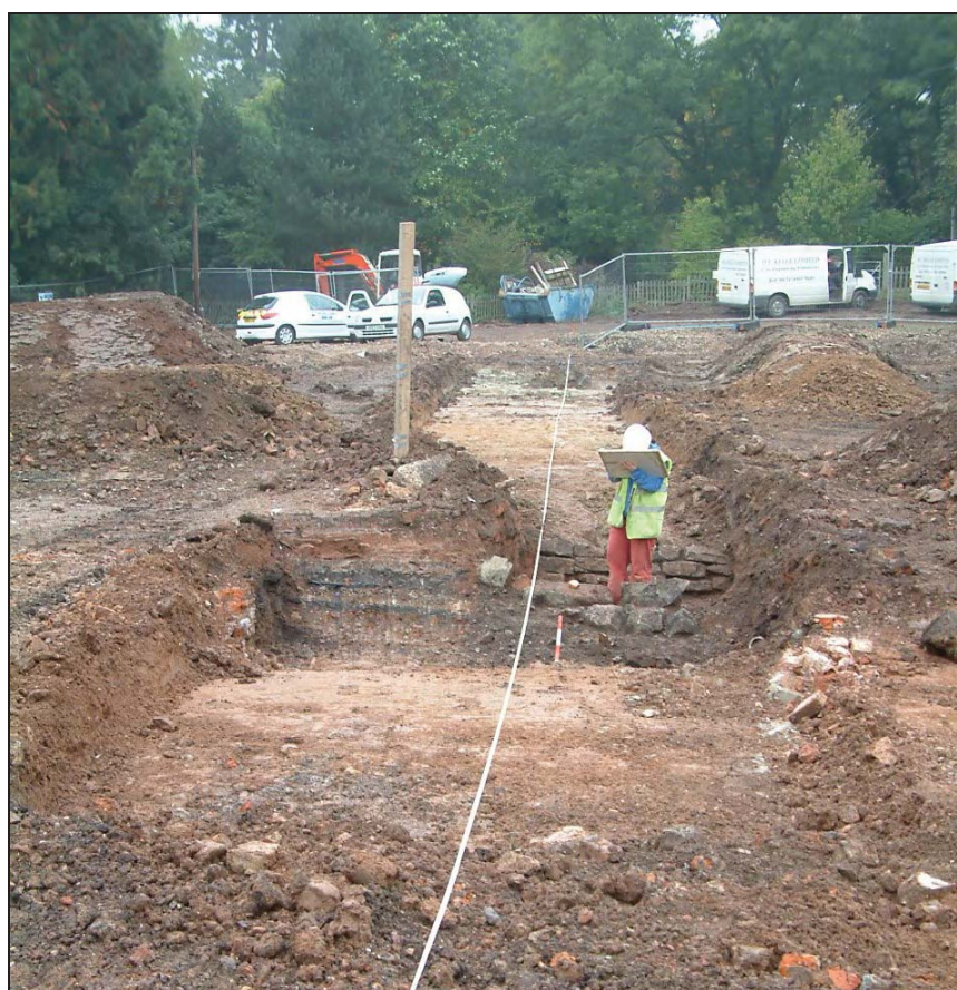
Plate 2: View along Trench 3, facing north-east. The tail race crosses the trench from left to right
