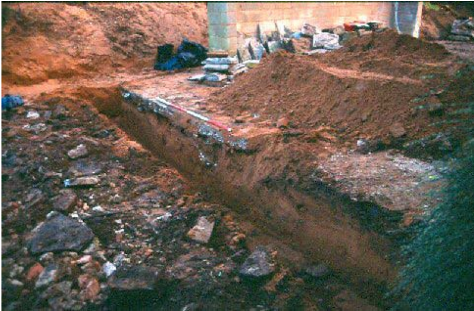
Plate 3: Trenching for new garage, looking southeast
