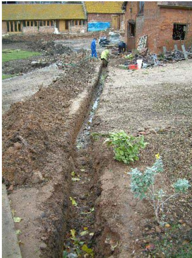
Plate 6: View north along service trench
