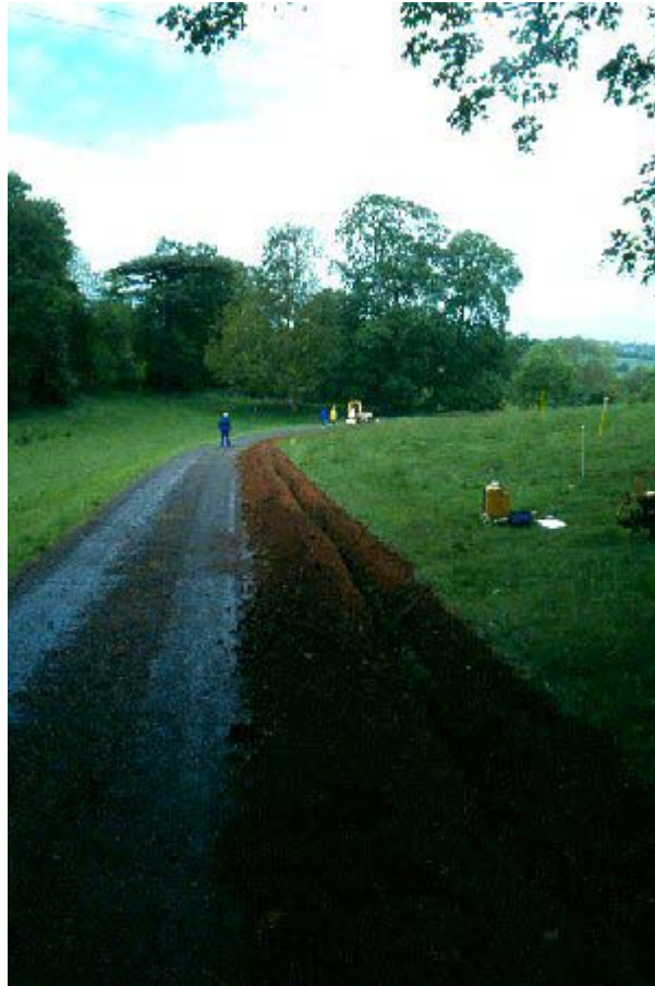
Plate 1: Gas pipeline trench from Evesham Road entrance
