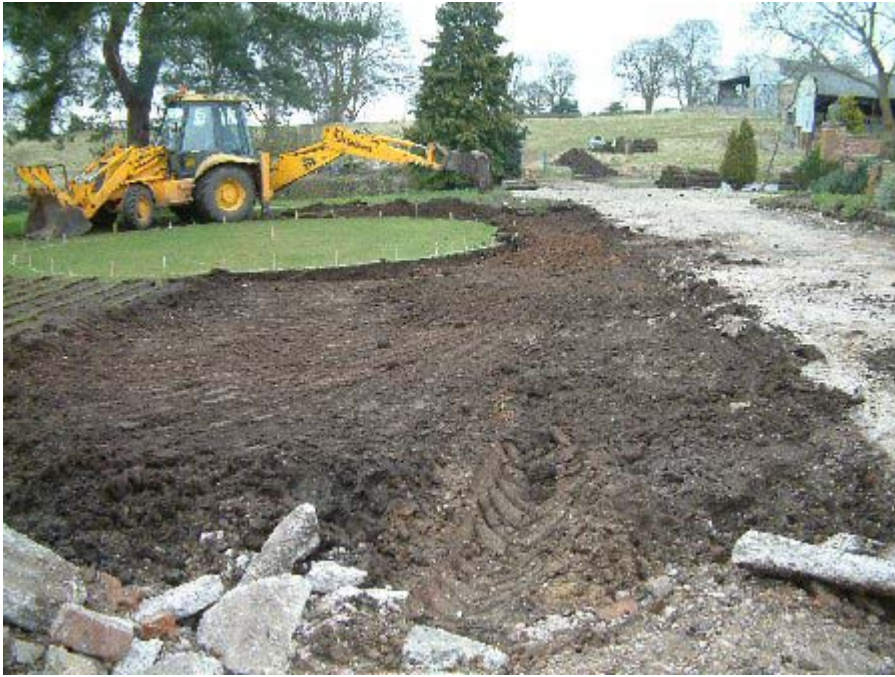
Plate 9: Machining of the new turning circle
