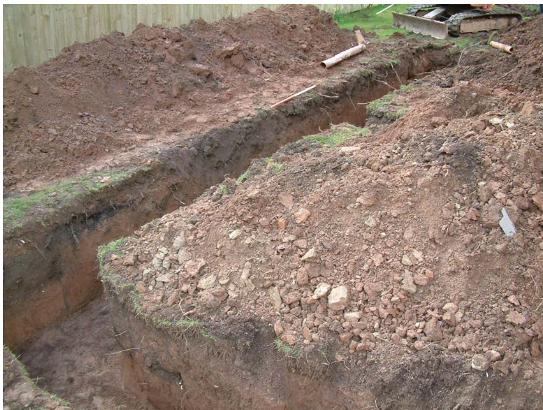
Plate 3: General view of groundworks, facing south-west
